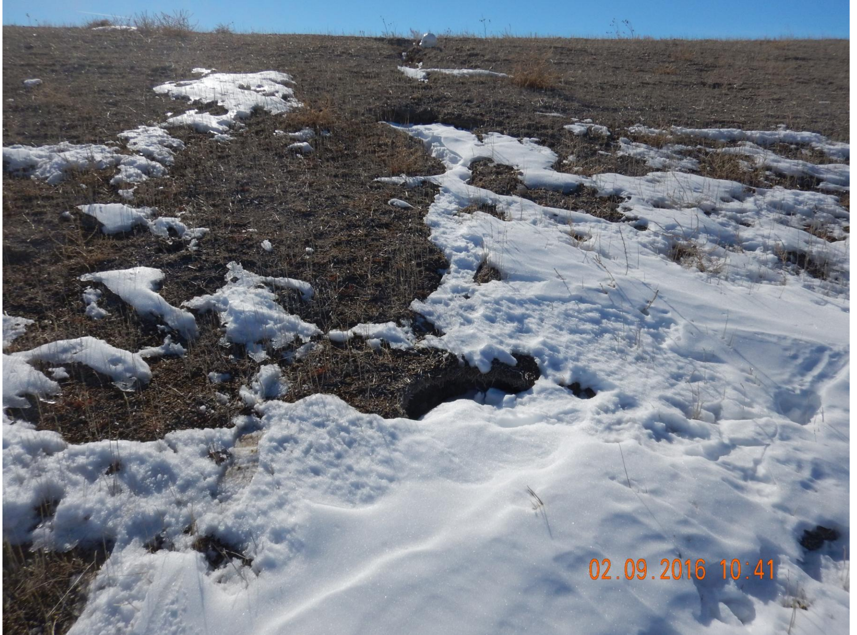
Figure 20: Photo taken from northern end berm on interim area, facing south. Photo shows rill erosion occurring on berm.
