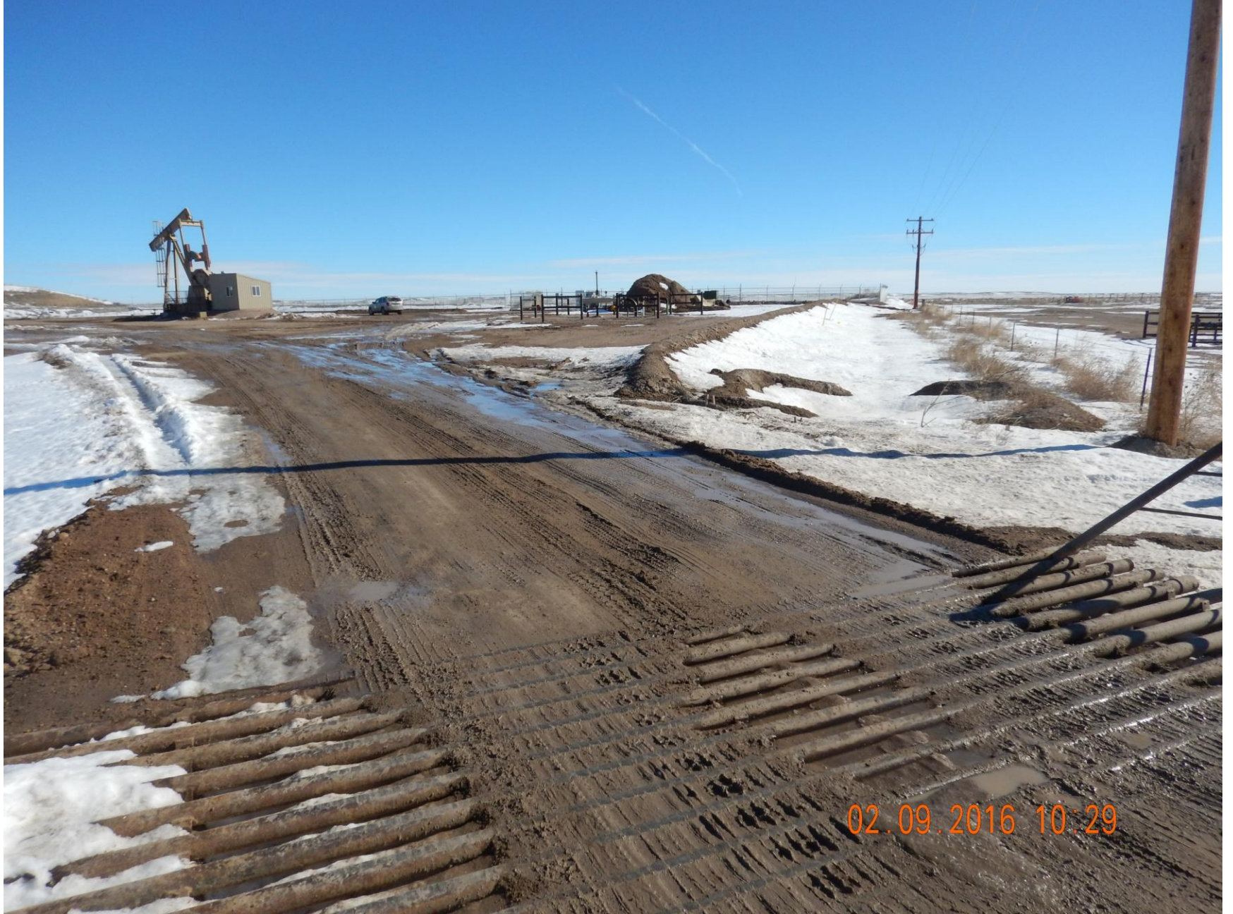
Figure 2: Photo taken from access road southwest of location, facing east. Photo of location, interim area and stormwater controls.
