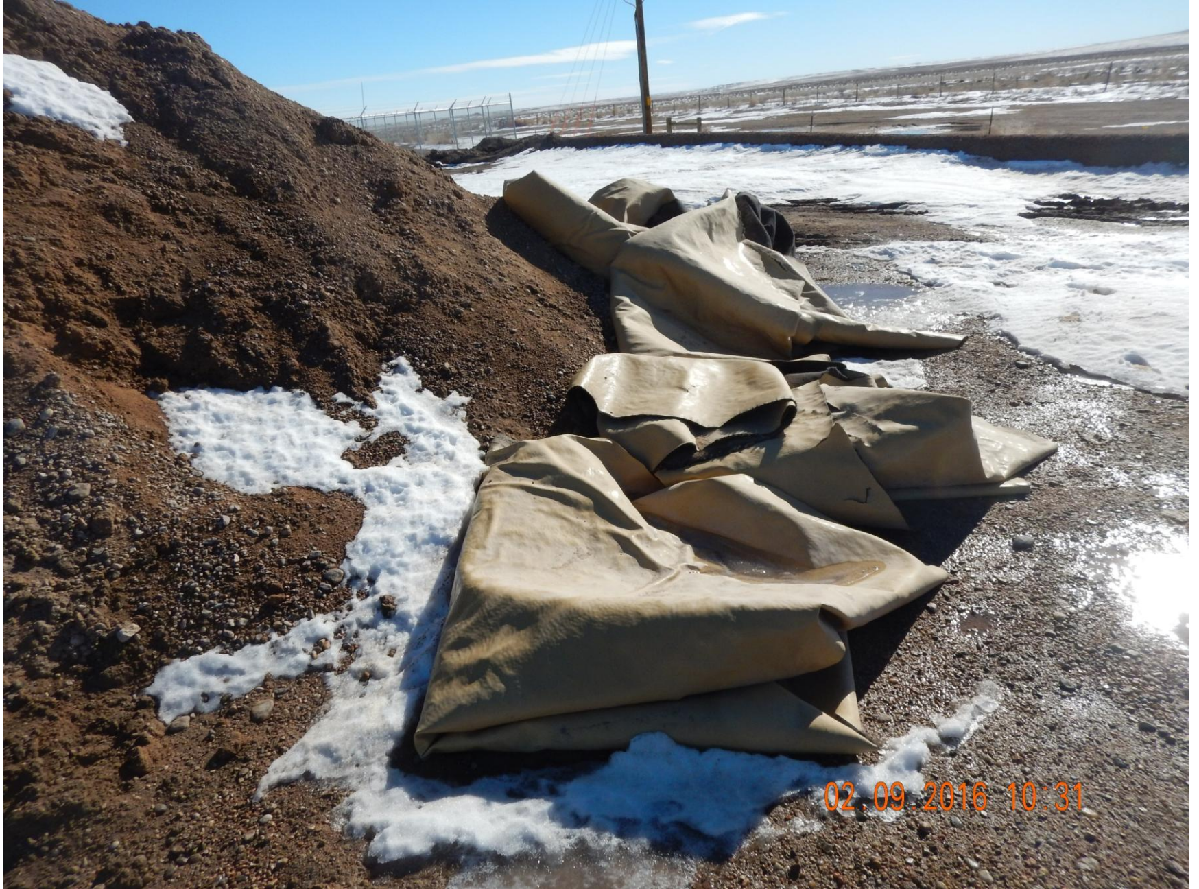
Figure 5: Photo taken from south end of location. Photo shows soil stockpile on project area, and what appears to be a tarp strewn next to soil stockpile.
