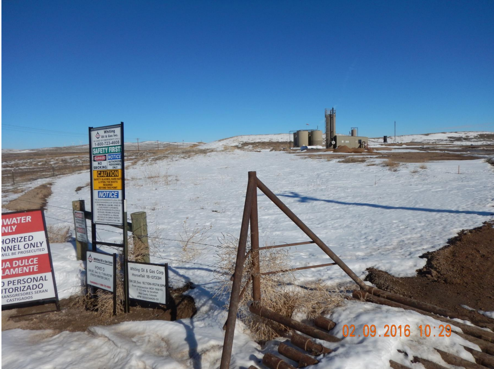
Figure 3: Photo taken from access road southwest of location, facing east. Photo shows location and interim area.
