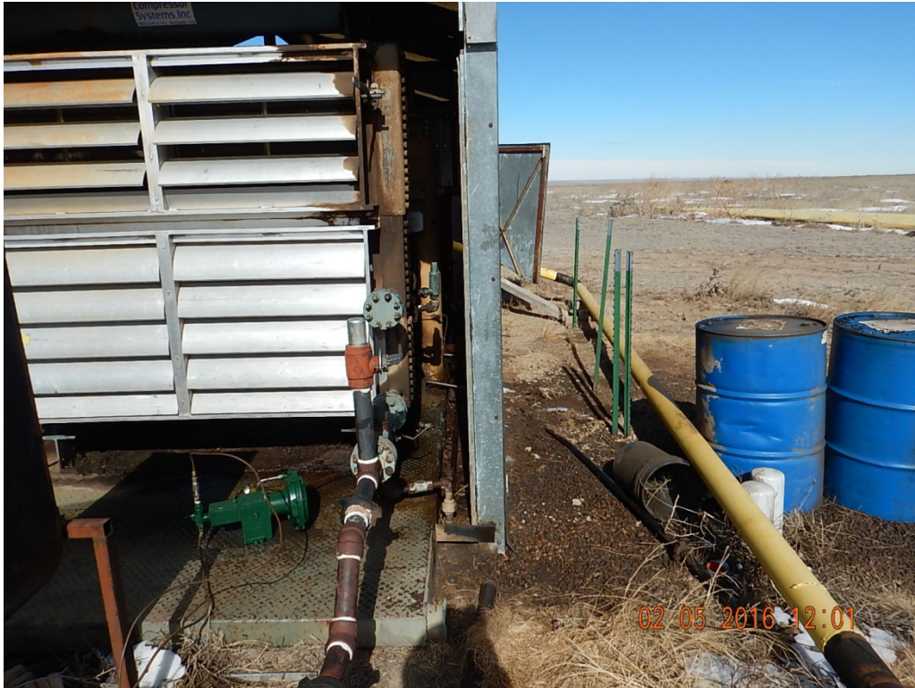
Figure 8 – Oil stained soil on east side of the compressor.
