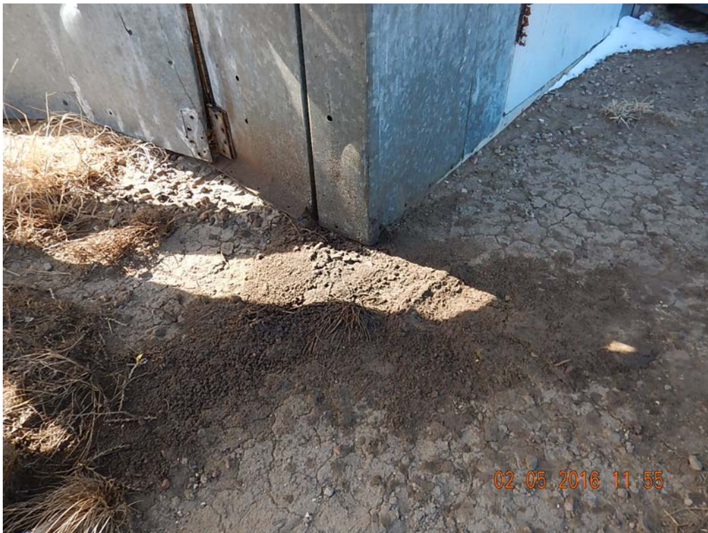
Figure 4 – Stained soil on northeast corner of compressor.
