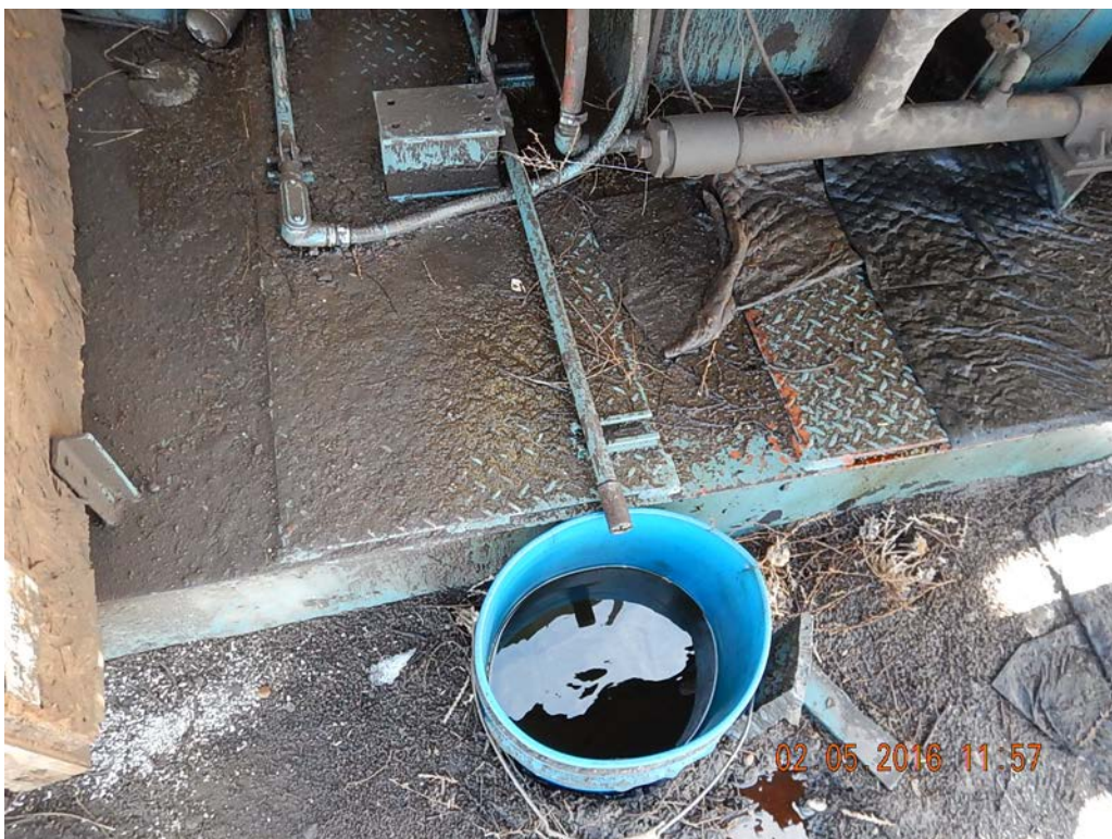
Figure 6 – Lube oil drain bucket on west side of compressor station.
