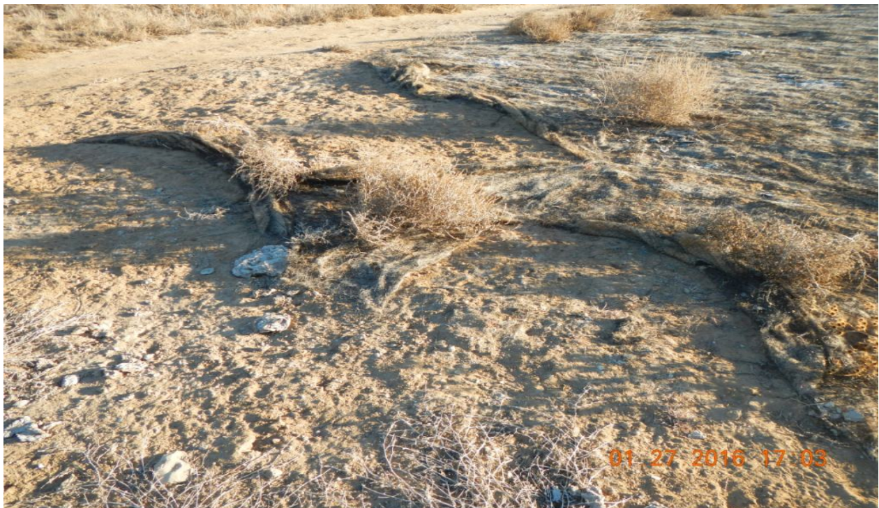
photo 4: Straw blanket is in disrepair at the northeast corner of the location.
