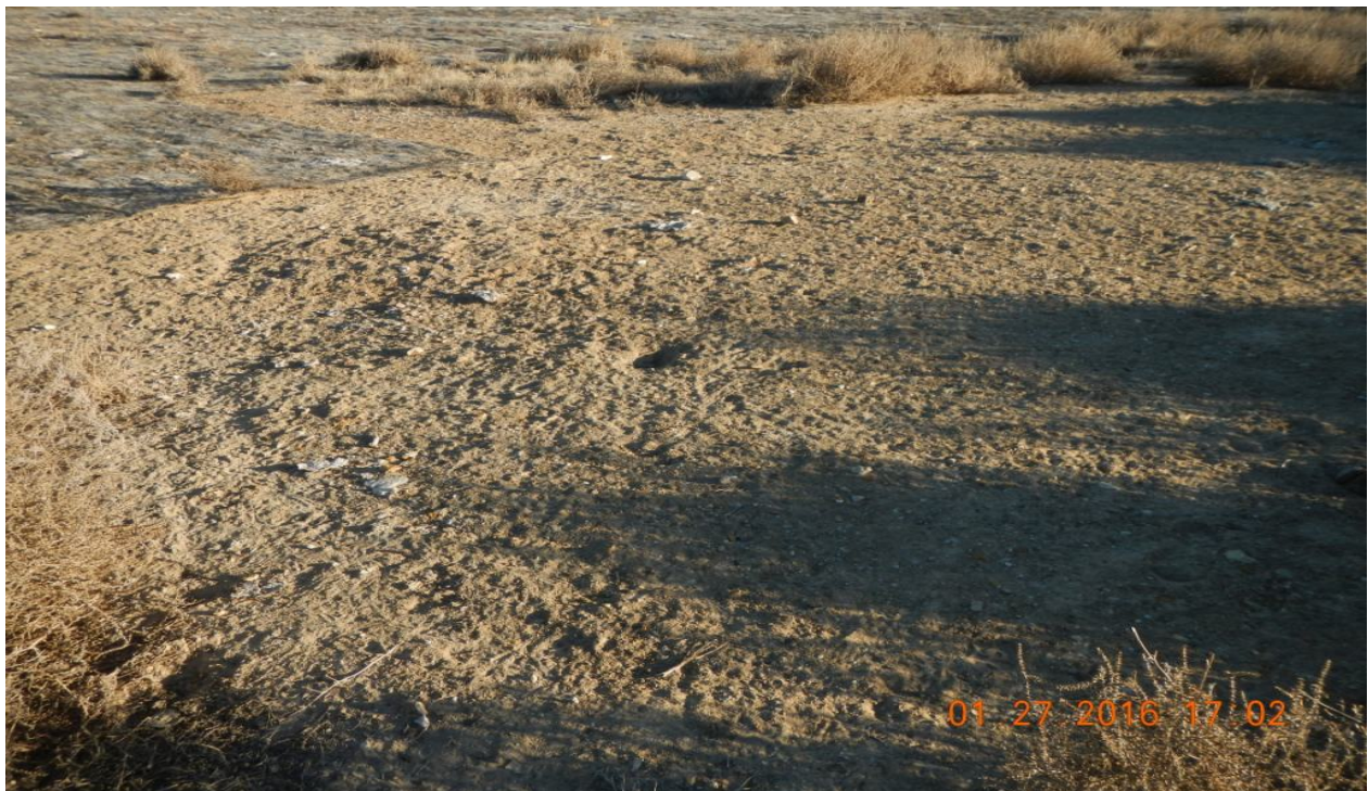
photo 8: Northwest corner of the location. Vegetation is not establishing where straw blanket was not installed.
