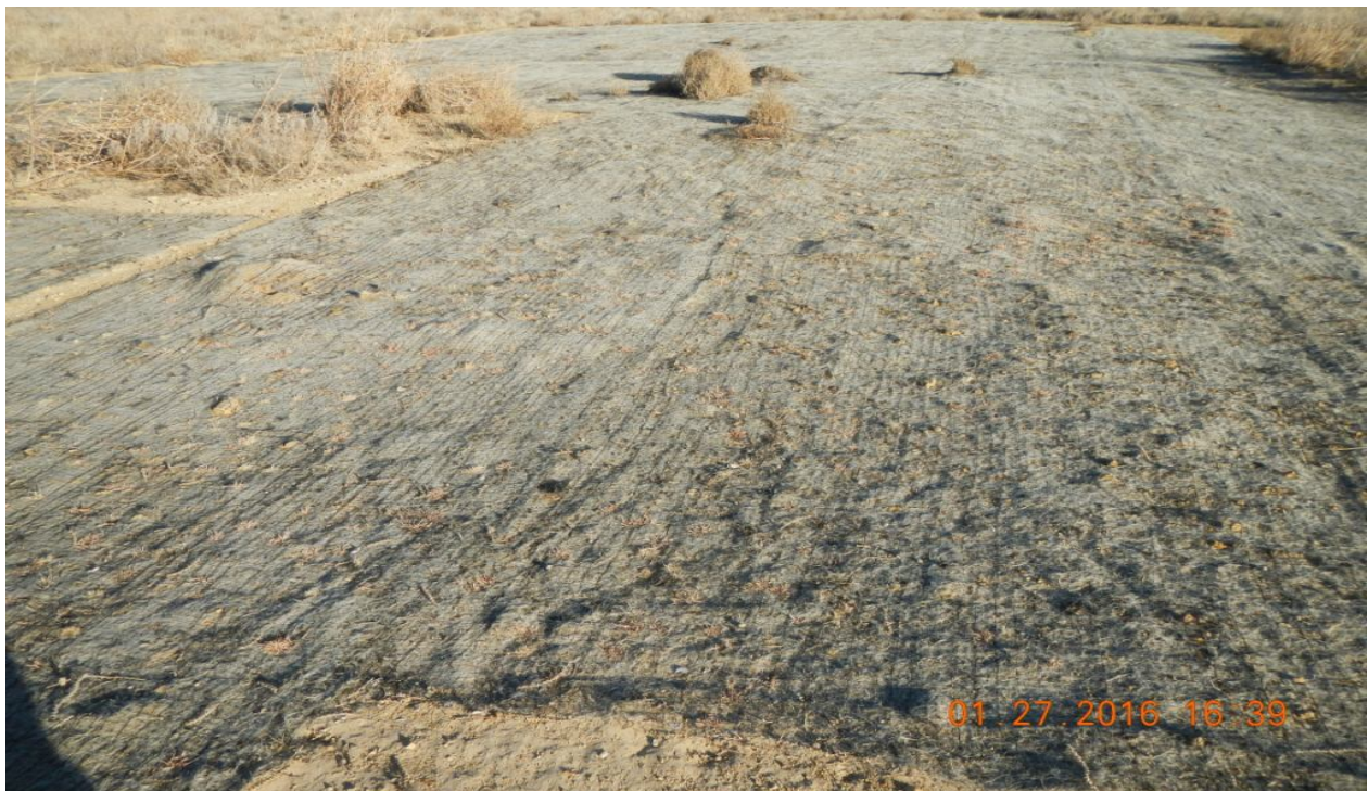
photo 4: Blanket has been installed east portion of the location.
