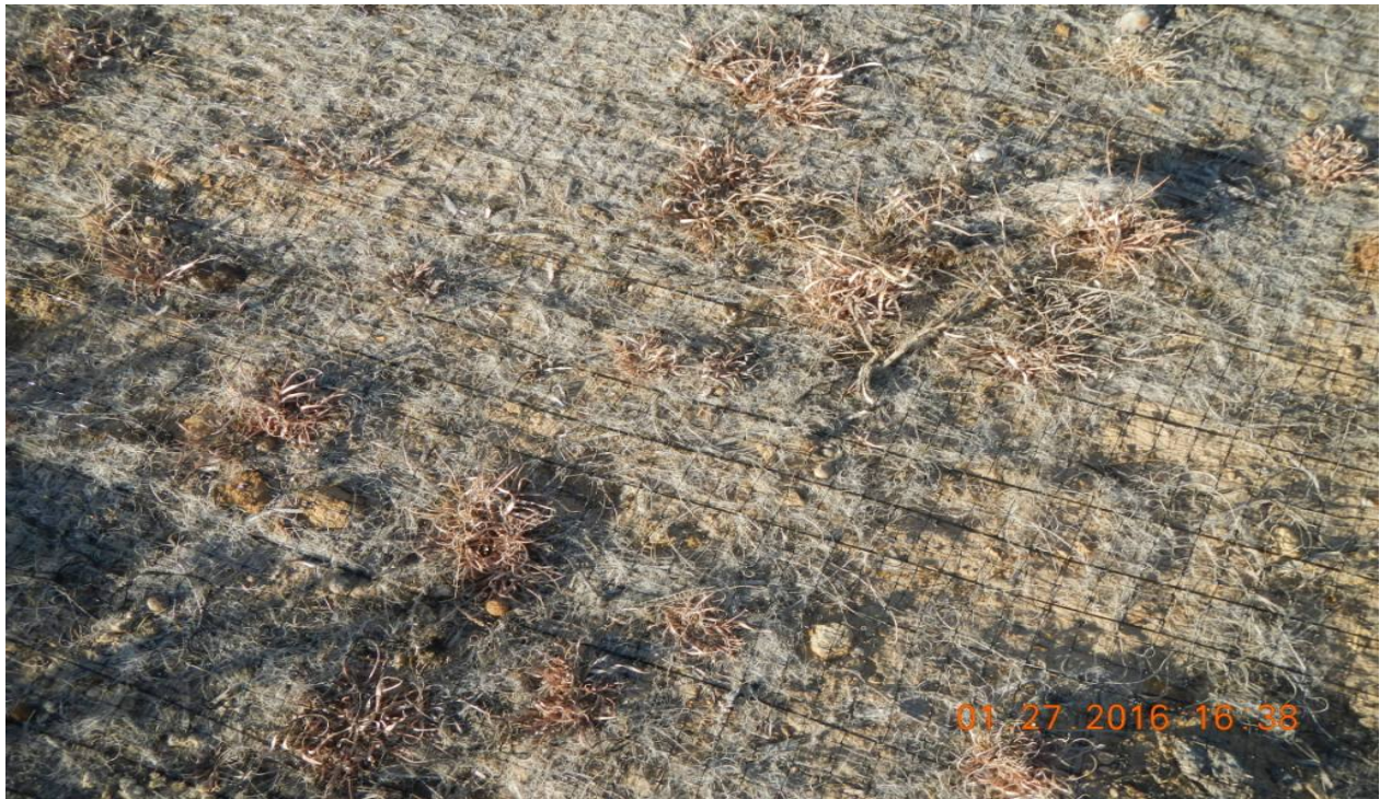
photo 5: Vegetation appears to be establishing where the blanket has been installed.
