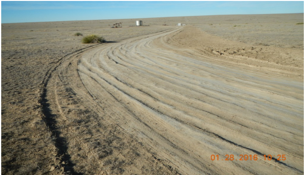
photo 5: Access is not being restricted along the access road. Evidence of rutting exists.
