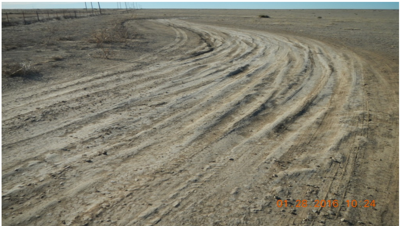
photo 4: Evidence of rutting occurring along the access road.
