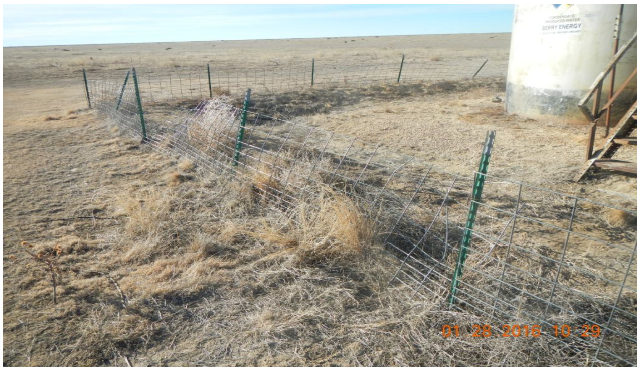
photo 10: Fence around the tank battery is in disrepair.
