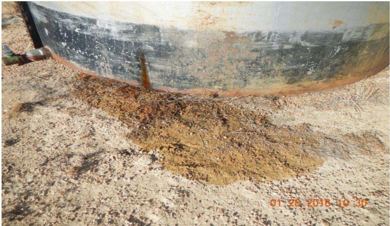
photo 11: There is an area (~3'x1') of oil stained soil next to the tank battery.
