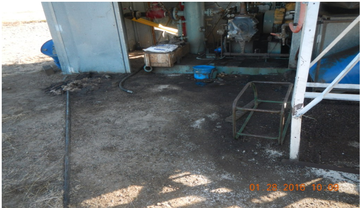
photo 5: Oil stained soil around the west side of the compressor.
