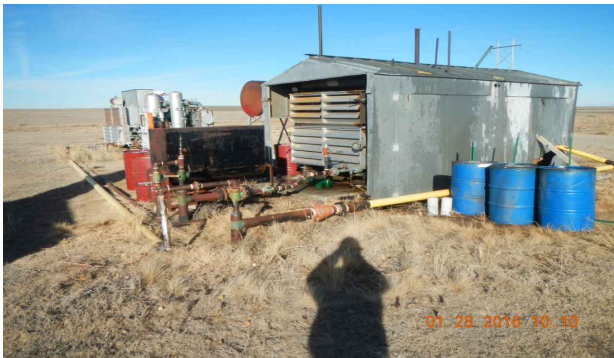
photo 10: Facing northwest. No secondary containment around barrels.
