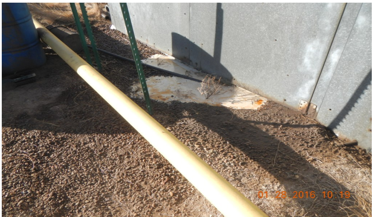
photo 12: Oily fluid coming out of the east side of the compressor shed.
