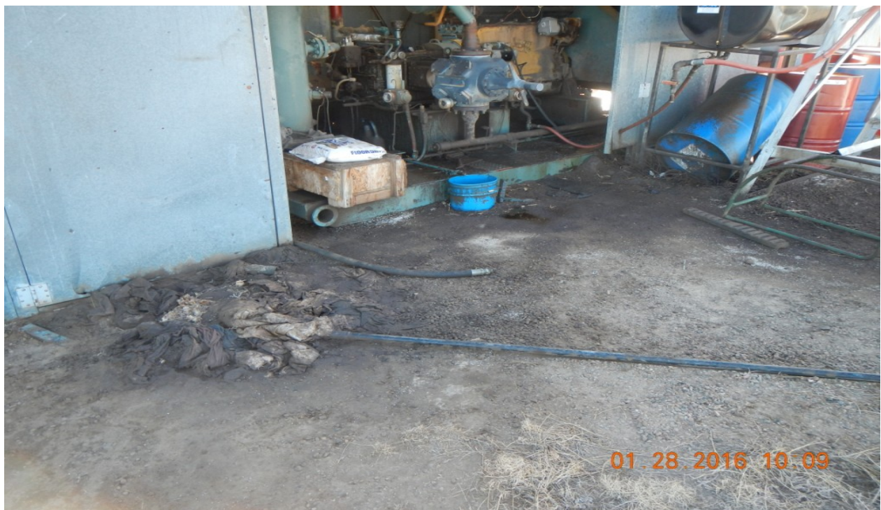
photo 6: Oil stained soil around the west side of the compressor.
