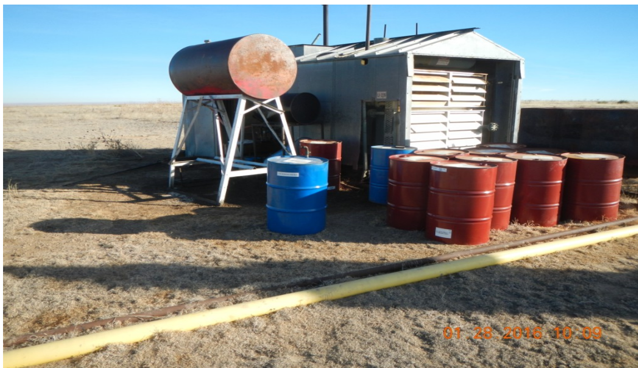
photo 4: Facing northeast. No secondary containment around barrels and fuel tank.
