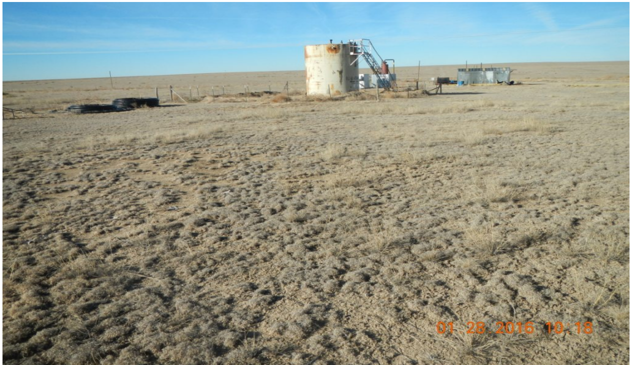
photo 11: Facing southwest toward the tank battery and the compressor.
