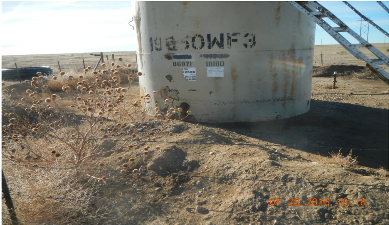
photo 5: Tank was not properly labeled and did not have a sign. Tank does not appear to be in use.
