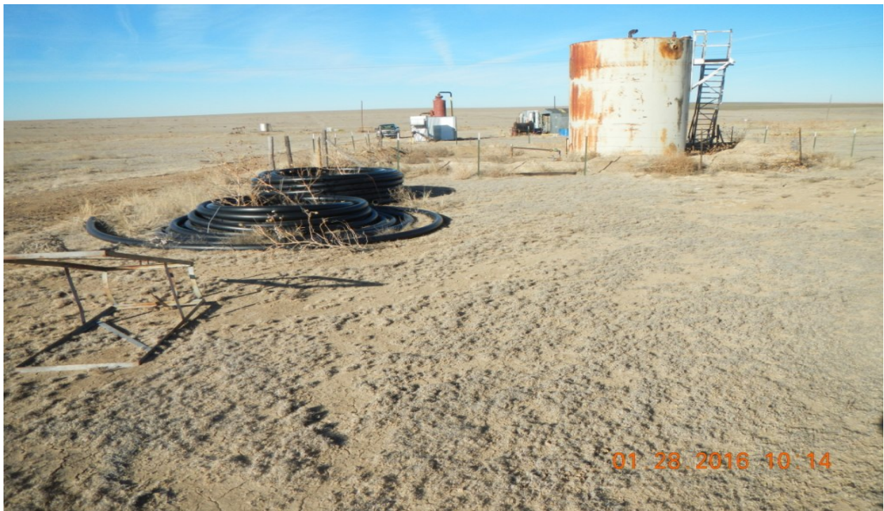
photo 6: Facing west. Unused equipment is being stored near the tank battery.
