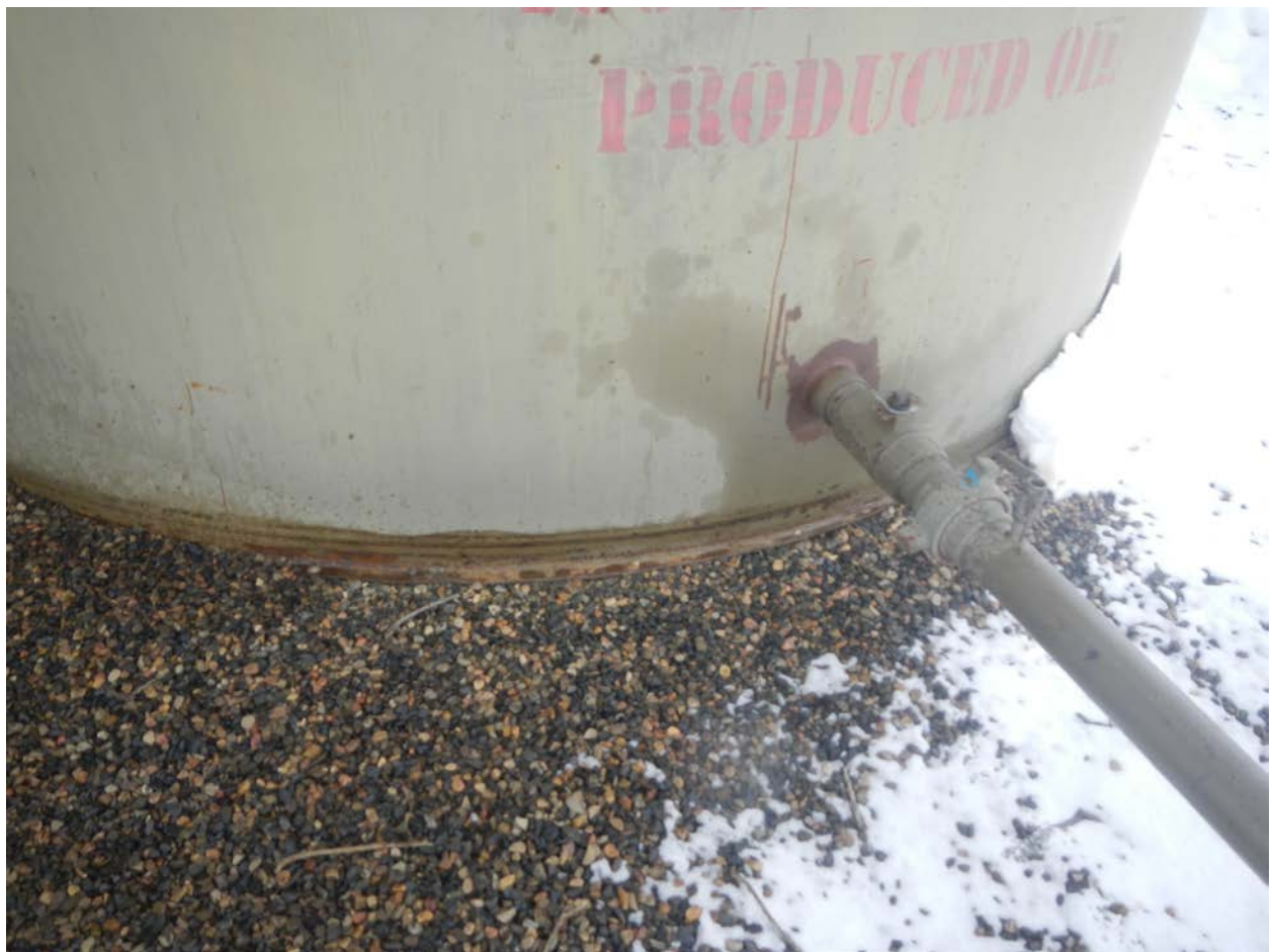
Note "high water" mark on tank.
