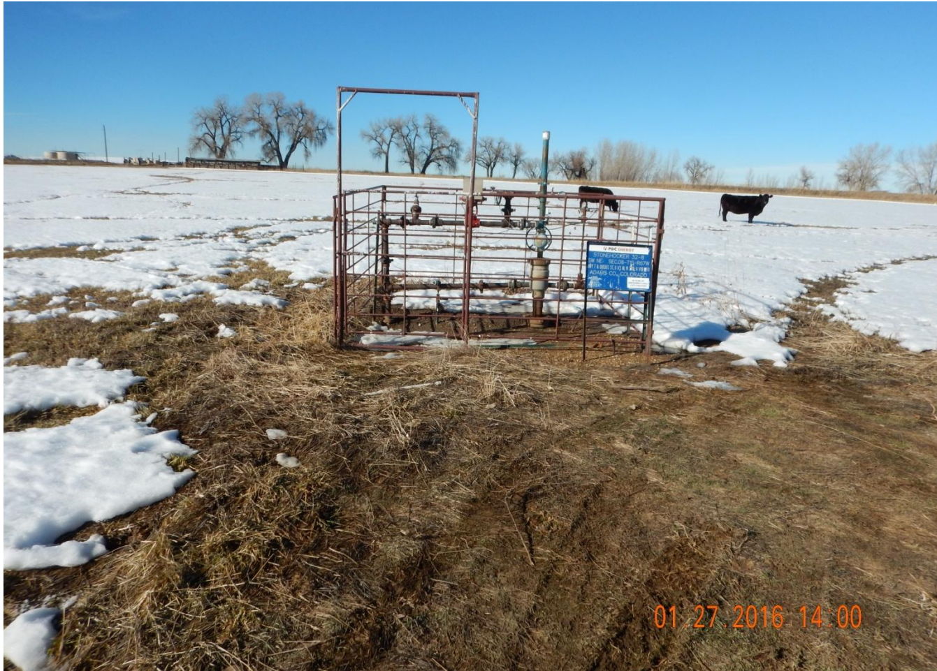
Photo 2. Photo taken of PR well 001-09387, confirming the AL status of 001-09559. It appears 001-09559 was never built at location. This is a well release on an active location.
