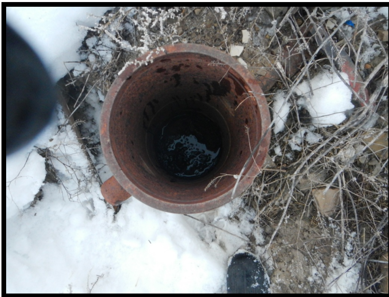
Photo#2: Looking down casing at water level 2ft. From top of Casing .
