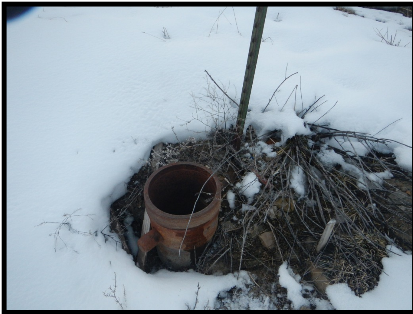
Photo#1: Open Pipe / Casing on Location.
