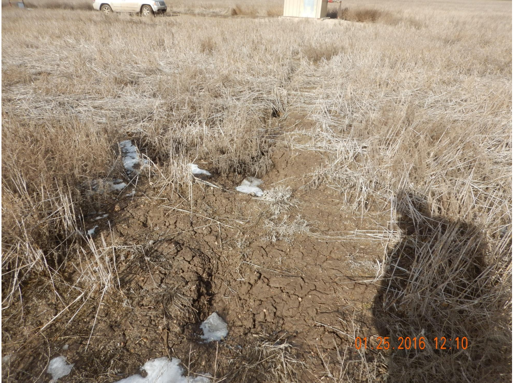
Figure 5: Photo taken south of location, facing north. Photo shows subsidence along pipeline to location.
