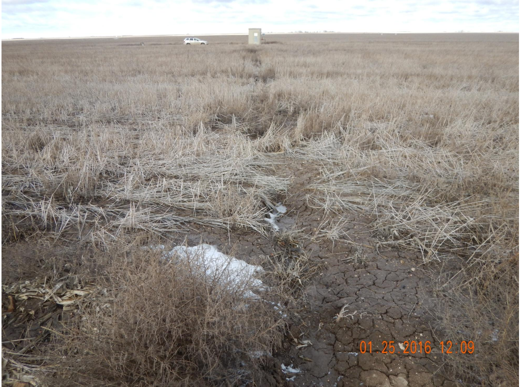
Figure 3: Photo taken south of location, facing north. Photo shows subsidence along pipeline to location.
