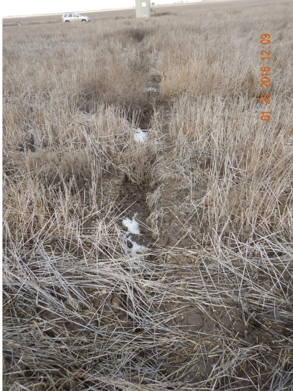
Figure 4: Photo taken south of location, facing north. Photo shows subsidence along pipeline to location.
