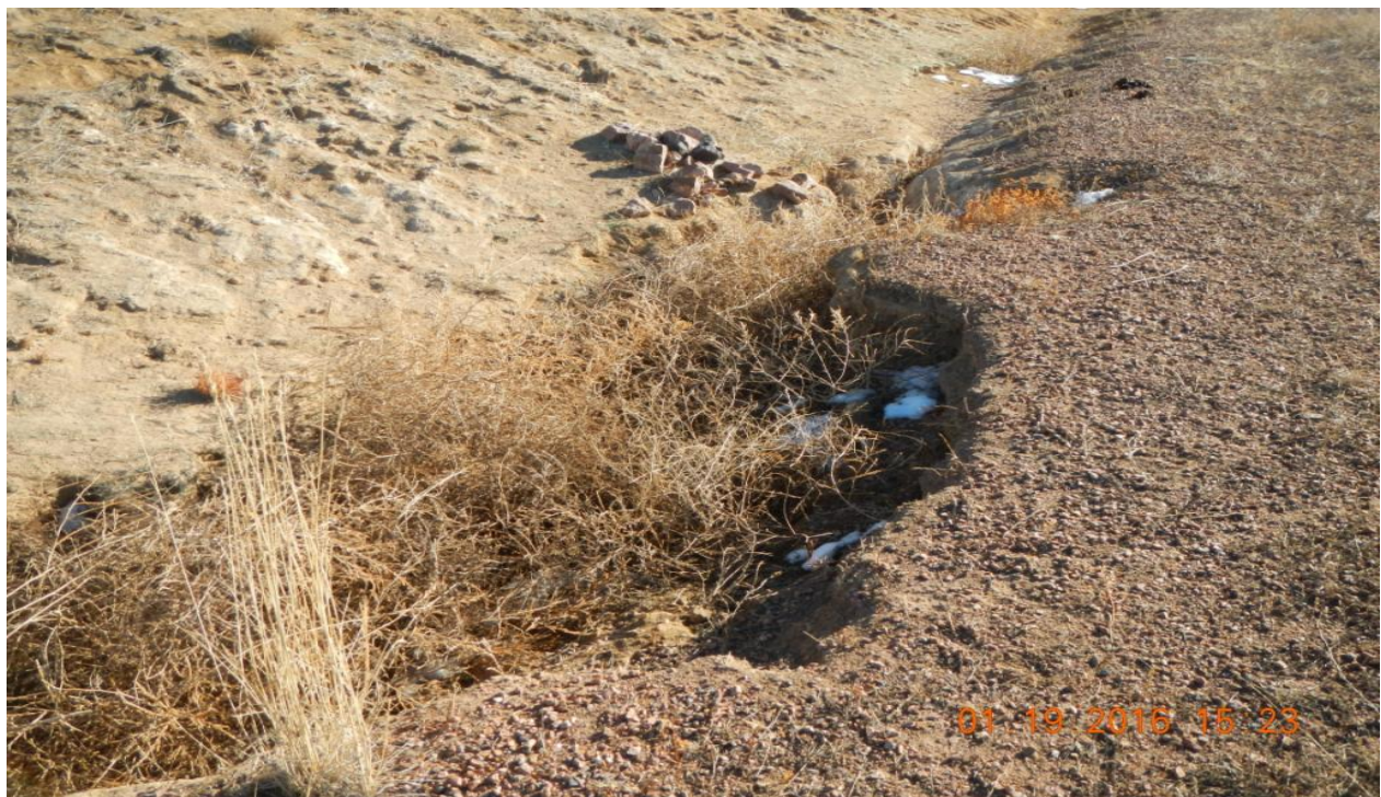
Photo 8: Erosion occurring along the east side of the access road. Rock check dams have been washed away.
