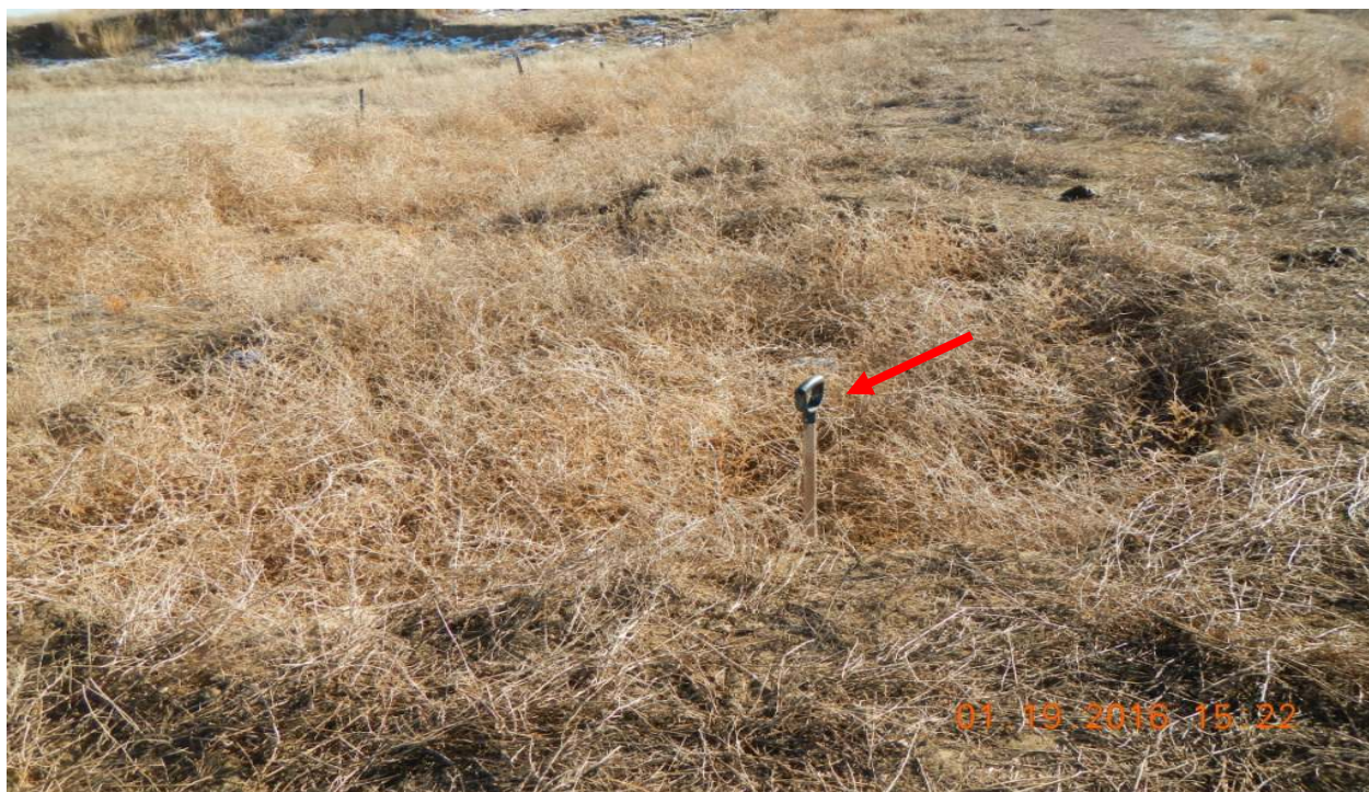
photo 5: An area of subsidence was noticed along the access road which is obscured by weed debris. Arrow indicates 3ft. shovel placed in the hole. Lat/Long: 38.74998,-104.55221
