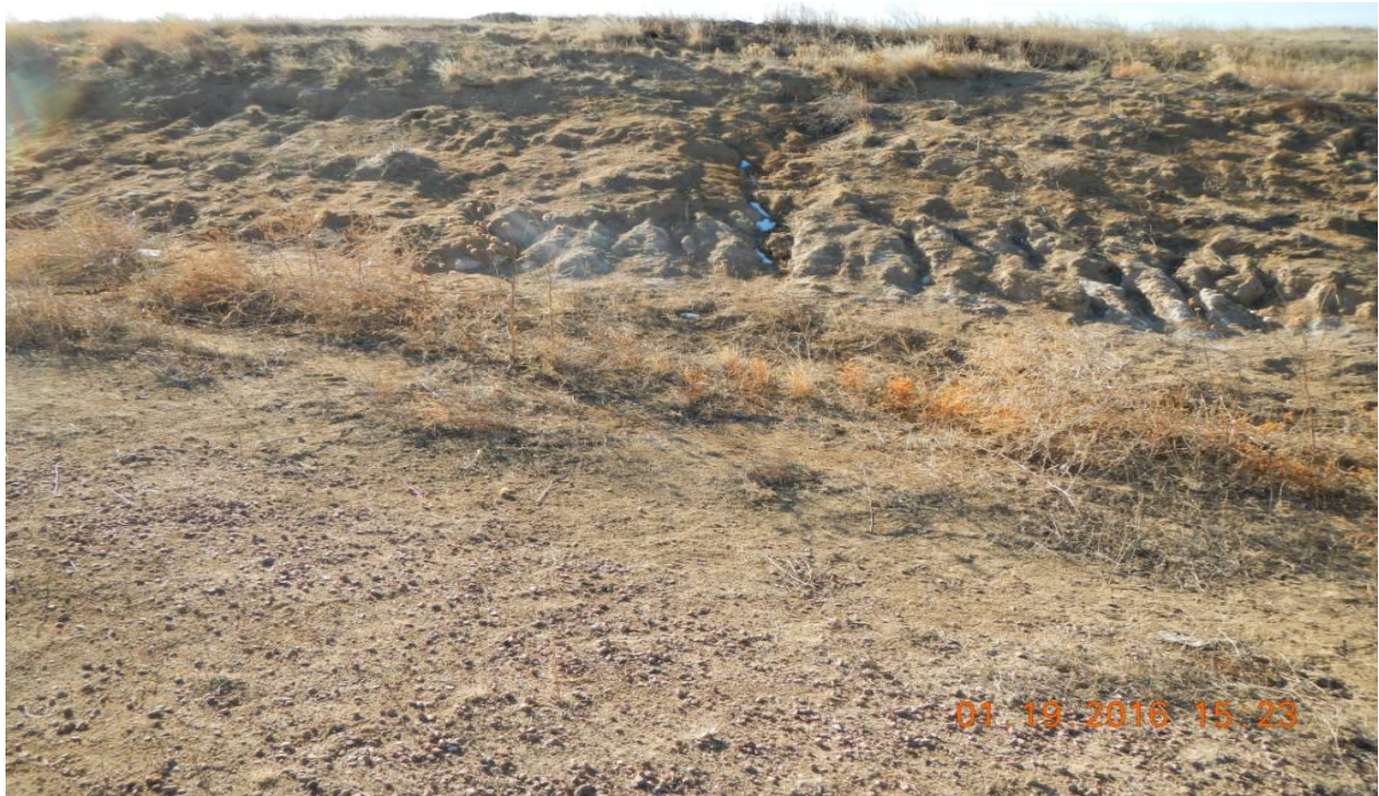
Photo 9: Erosion occurring along the west side of the access road.
