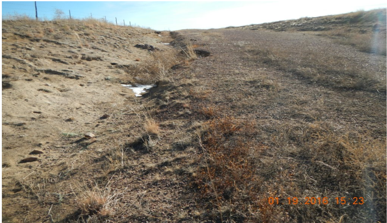
Photo 7: Facing south along the access road. Erosion is occurring along both sides of the access road in this area. Lat/Long: 38.74923,-104.55223
