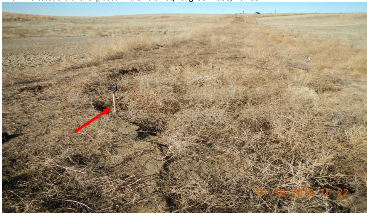
photo 6: Facing back towards the north at the area of subsidence along the access road. Arrow indicates 3ft. shovel placed in the hole. Lat/Long: 38.74998,-104.55221
