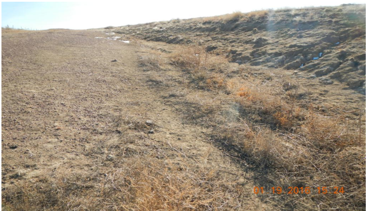
Photo 10: Erosion occurring along the west side of the access road.
