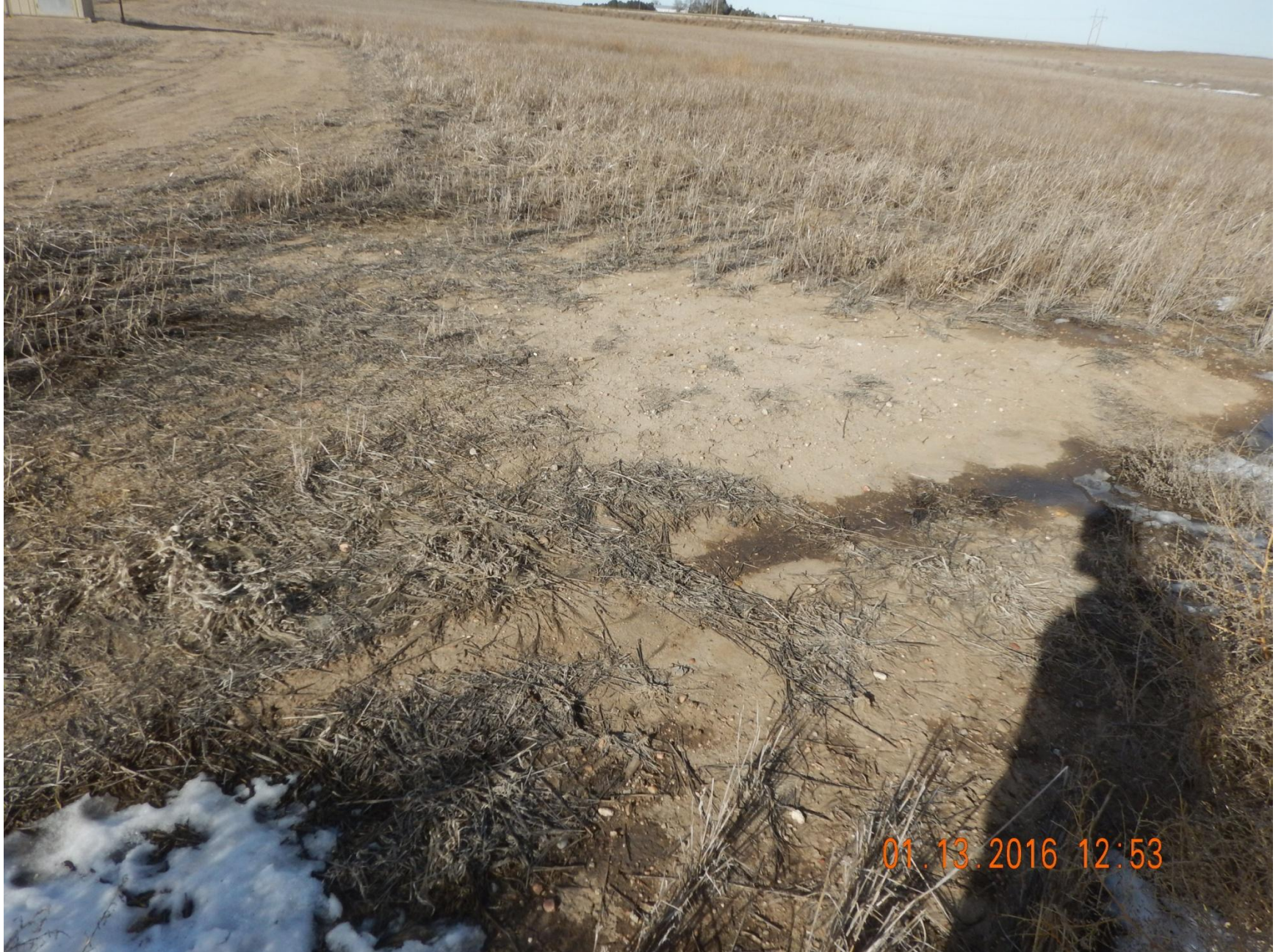
Figure 3: Photo taken from the east end of location, facing north. Photo shows portions of the interim area with sparse vegetation and exposed soil. Note the depression in the ground forming along pipeline.
