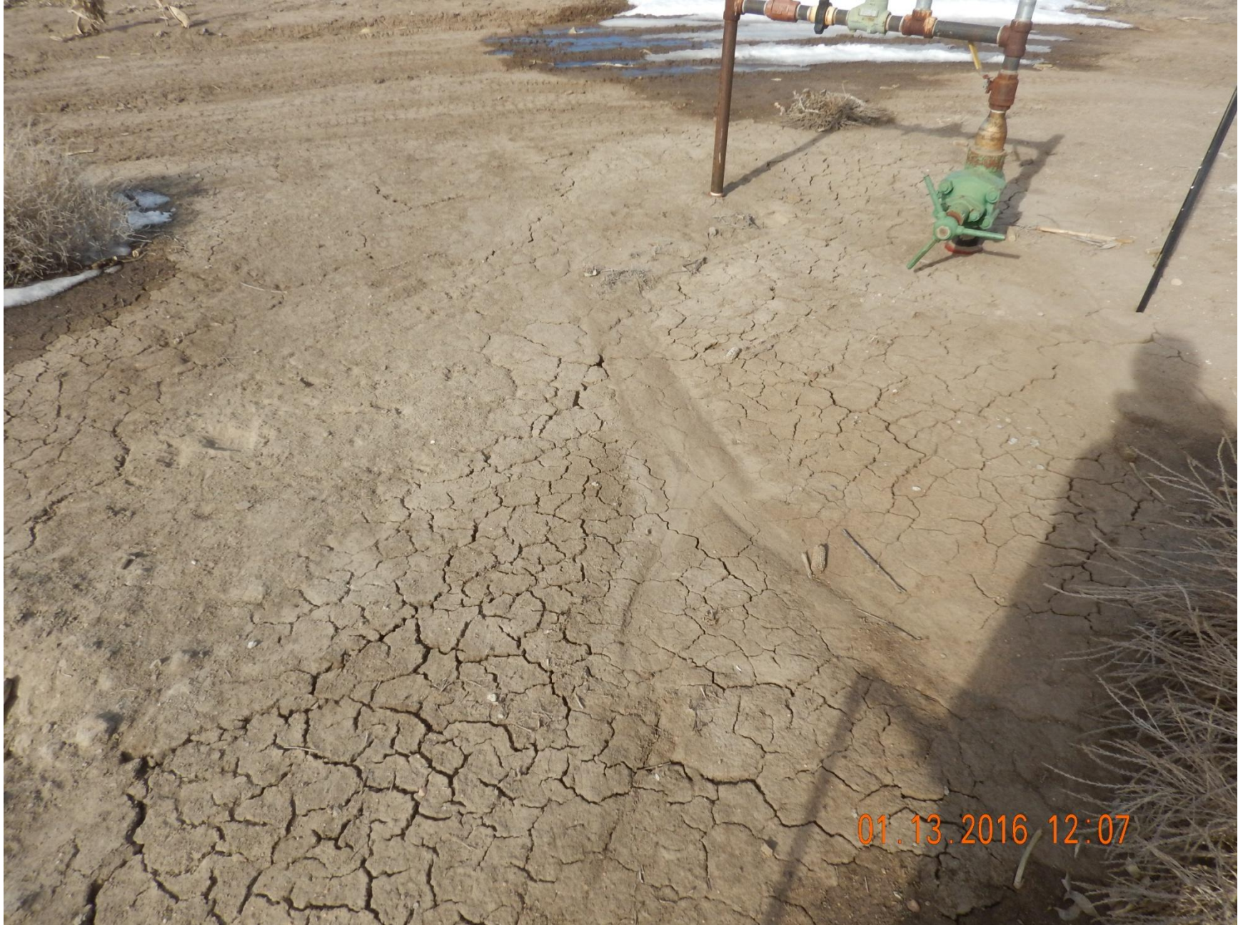
Figure 5: Photo taken at wellhead. Photo shows erosion starting to occur from the project area.
