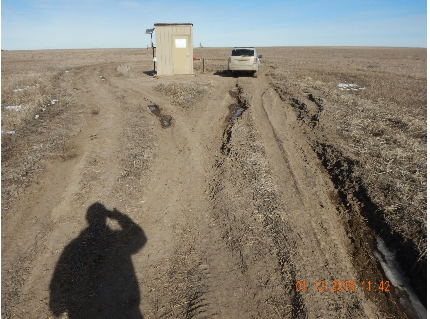
Figure 3: Photo taken from the south end of location, facing north. Photo shows access road in disrepair.
