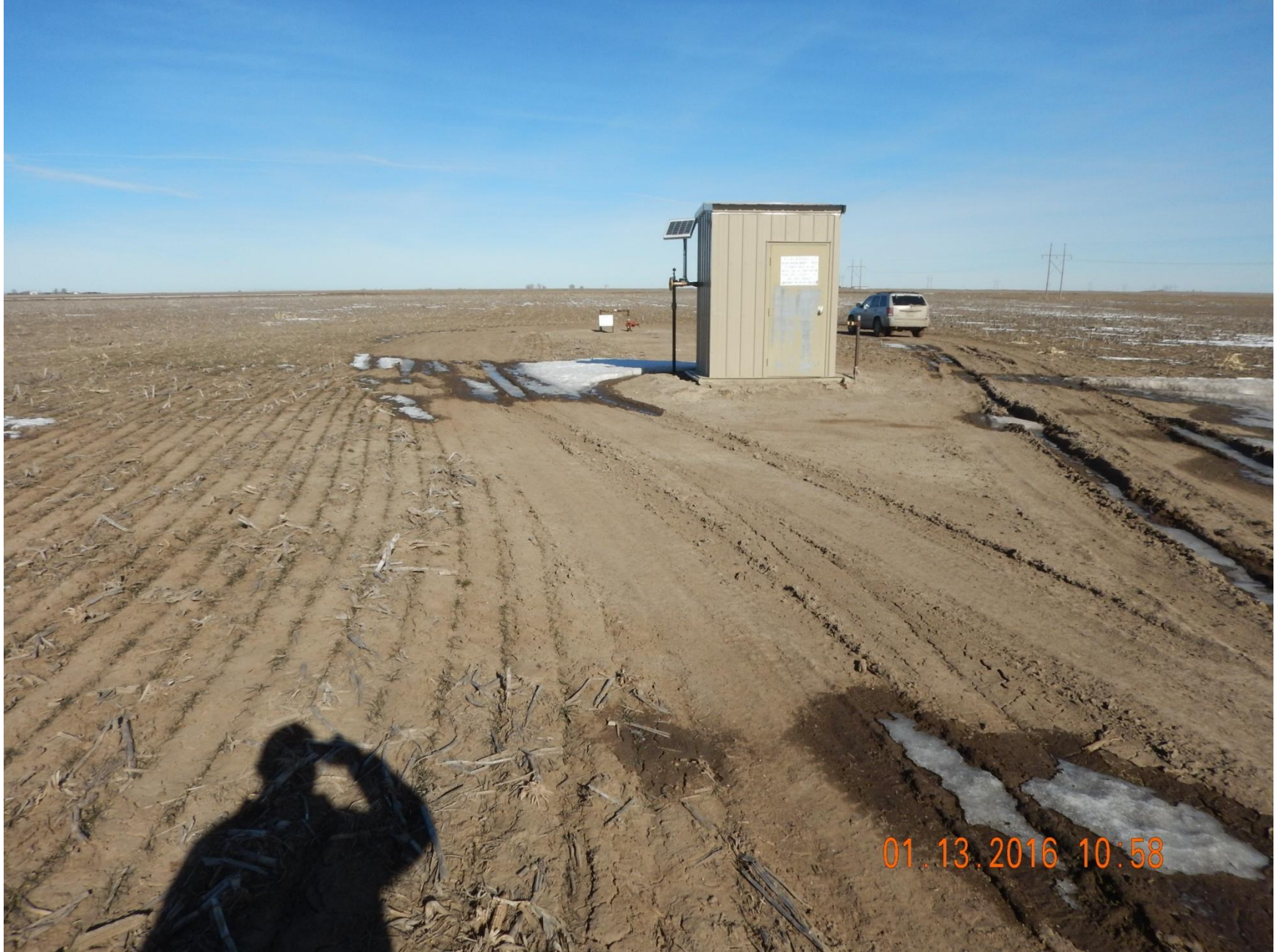
Figure 2: Photo taken from south end of location, facing north. Photo shows project and reclamation area.
