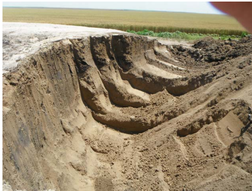
Bottom after excavation
