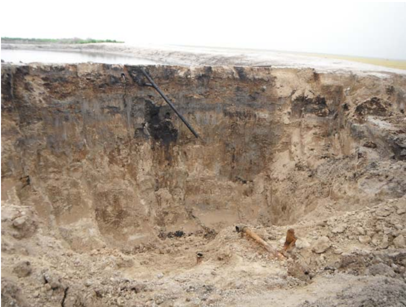
Partially excavated skim pit
