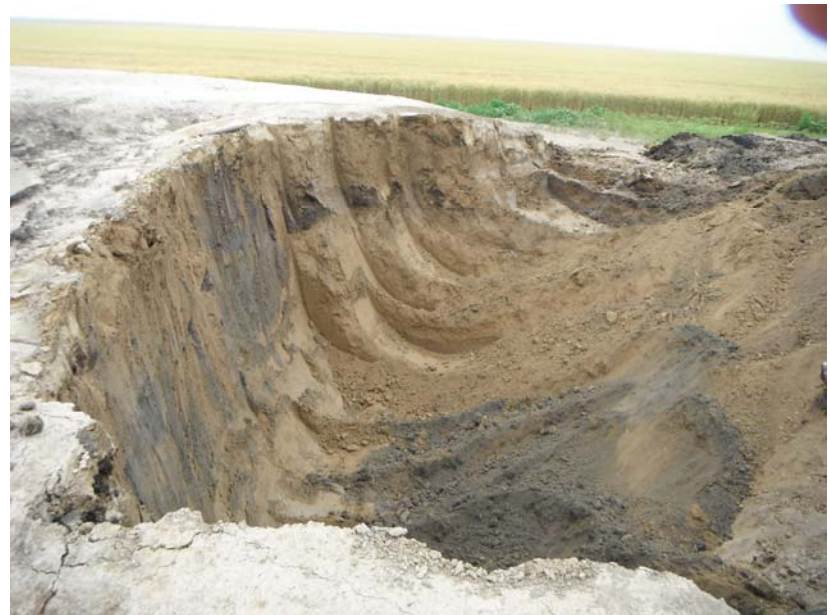
Excavation of impacted soil
