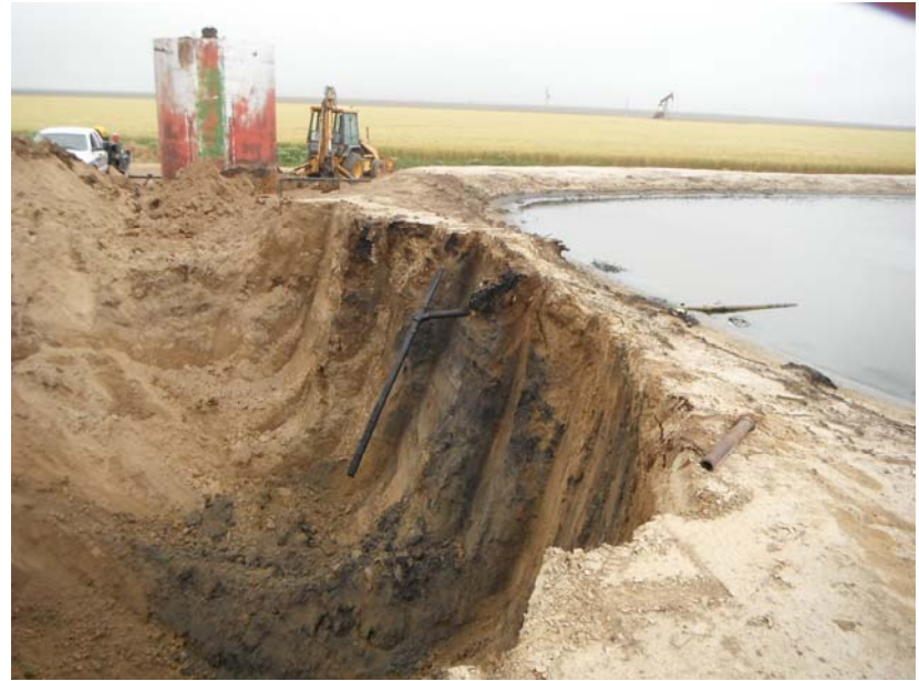
North wall shared with evaporation pit
