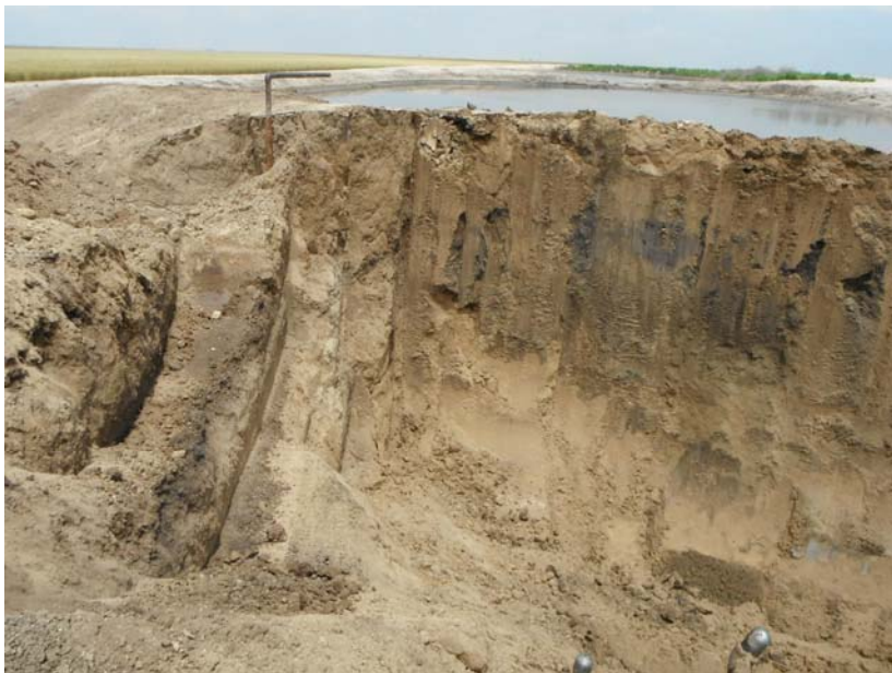
North (shared) wall after excavation
