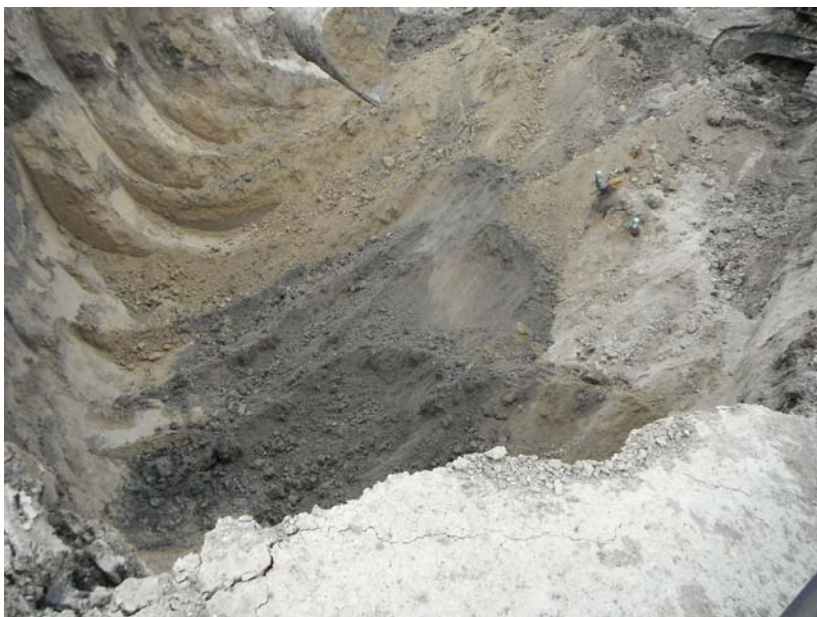
Excavation of skim pit south wall
