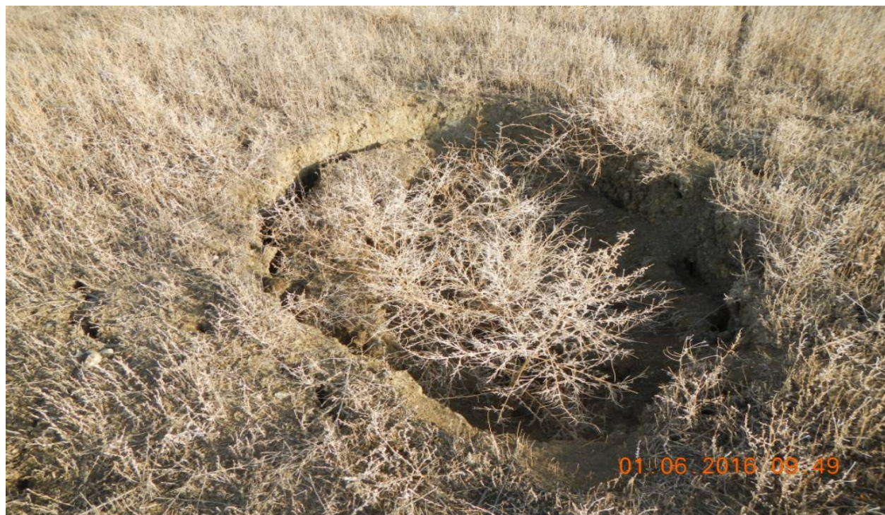
Photo 8: Another area of subsidence noticed at the location. Lat/Long:38.99608/-103.27706.
