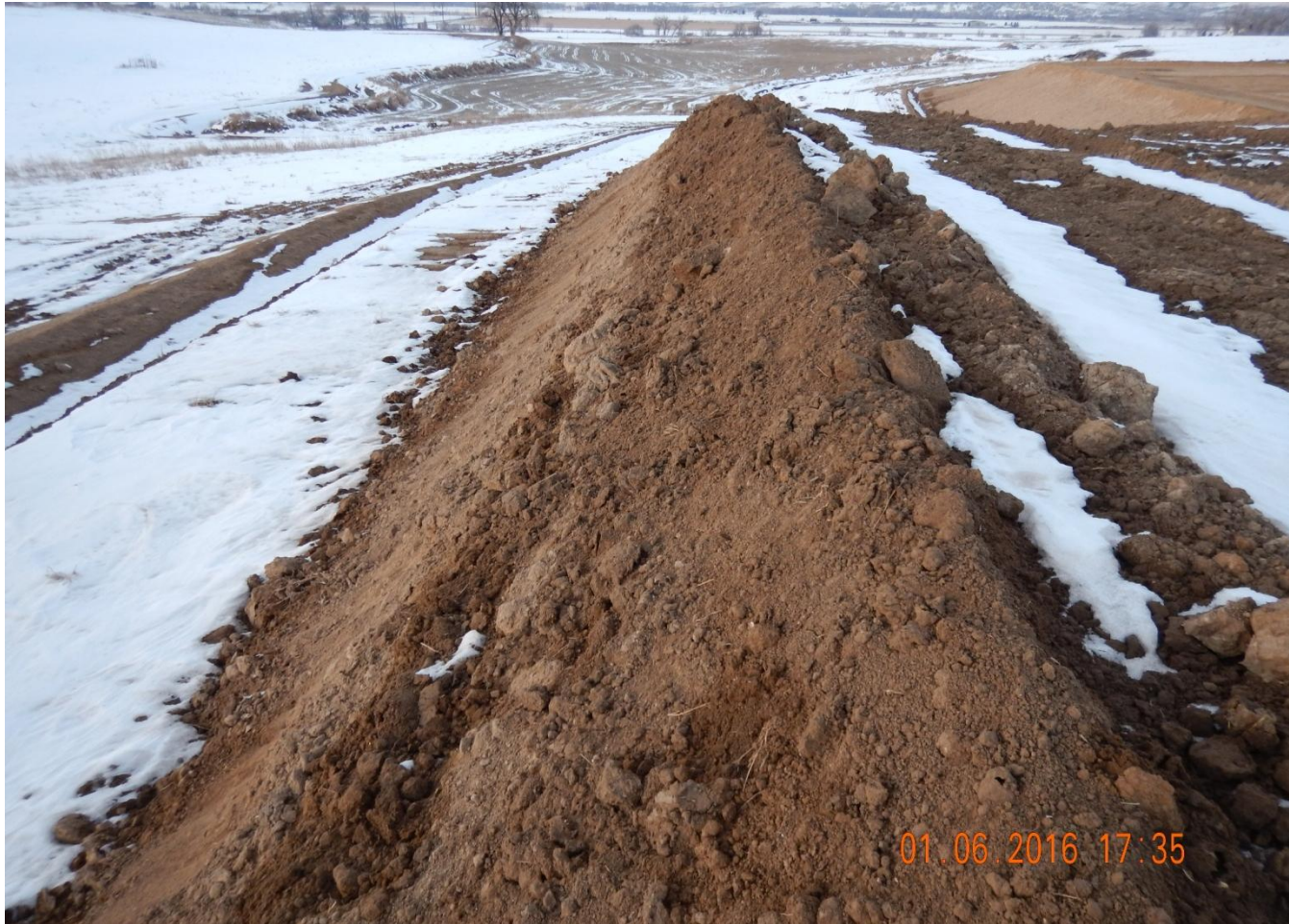
Photo 2. Photo taken from southwestern topsoil stockpile, facing North. All stockpiled soils shall be protected from degradation. The west-facing topsoil stockpile is steep and erodible. May need to stabilize slope like the east-facing slope (Refer to Photo 3).
