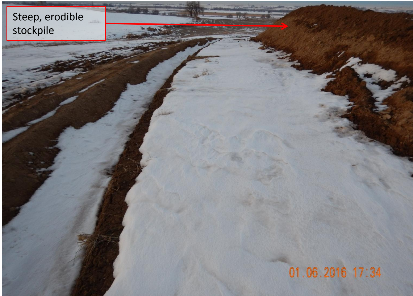
Photo 1. Photo taken from southwestern location, facing North. Stormwater BMP installed in center of photo. All stockpiled soils shall be protected from degradation. The west-facing topsoil stockpile is steep and erodible. Refer to photo 2.
