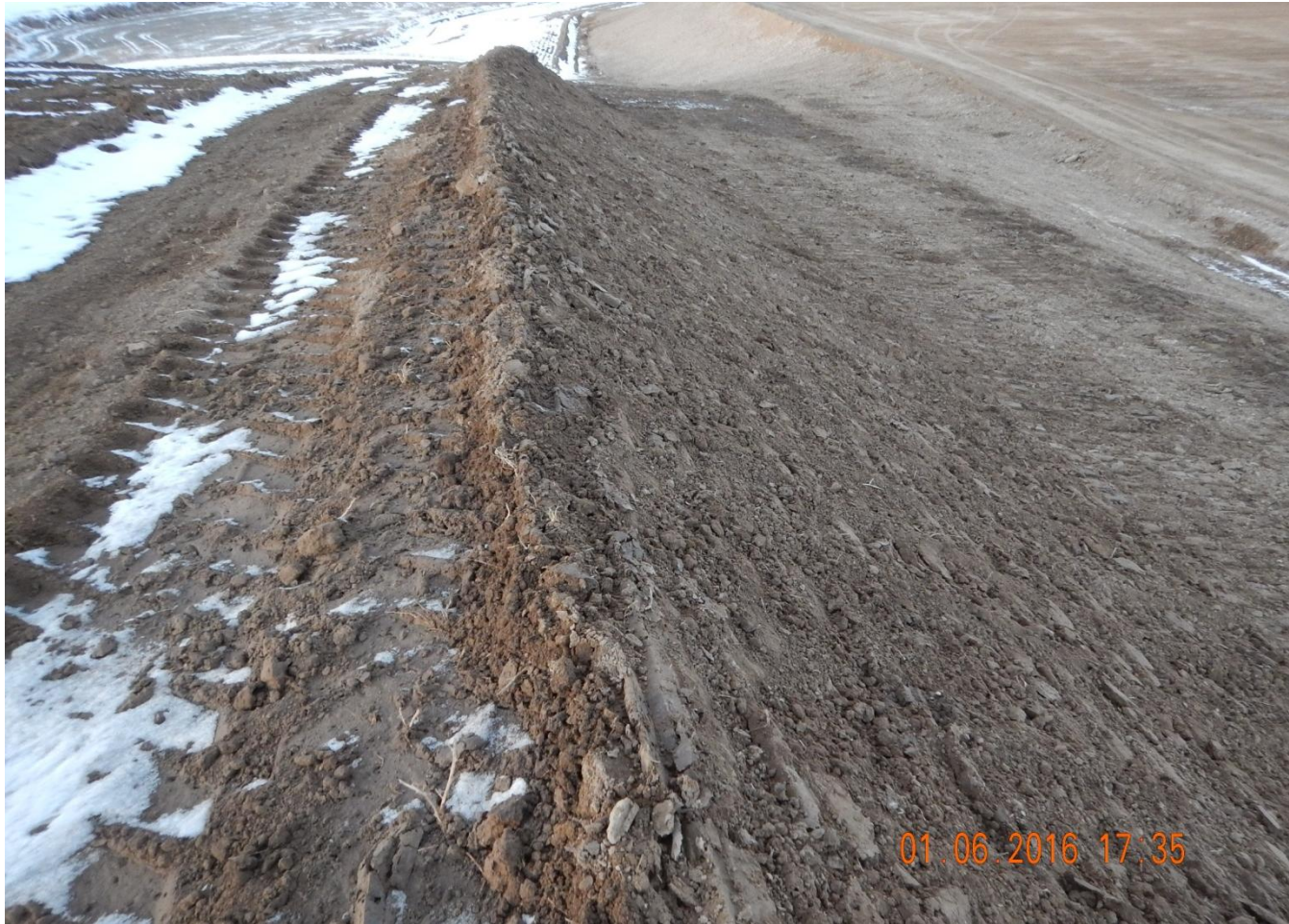
Photo 3. Photo taken from southwestern topsoil stockpile, facing North. East-facing topsoil stockpile properly tracked and slope is not too steep.
