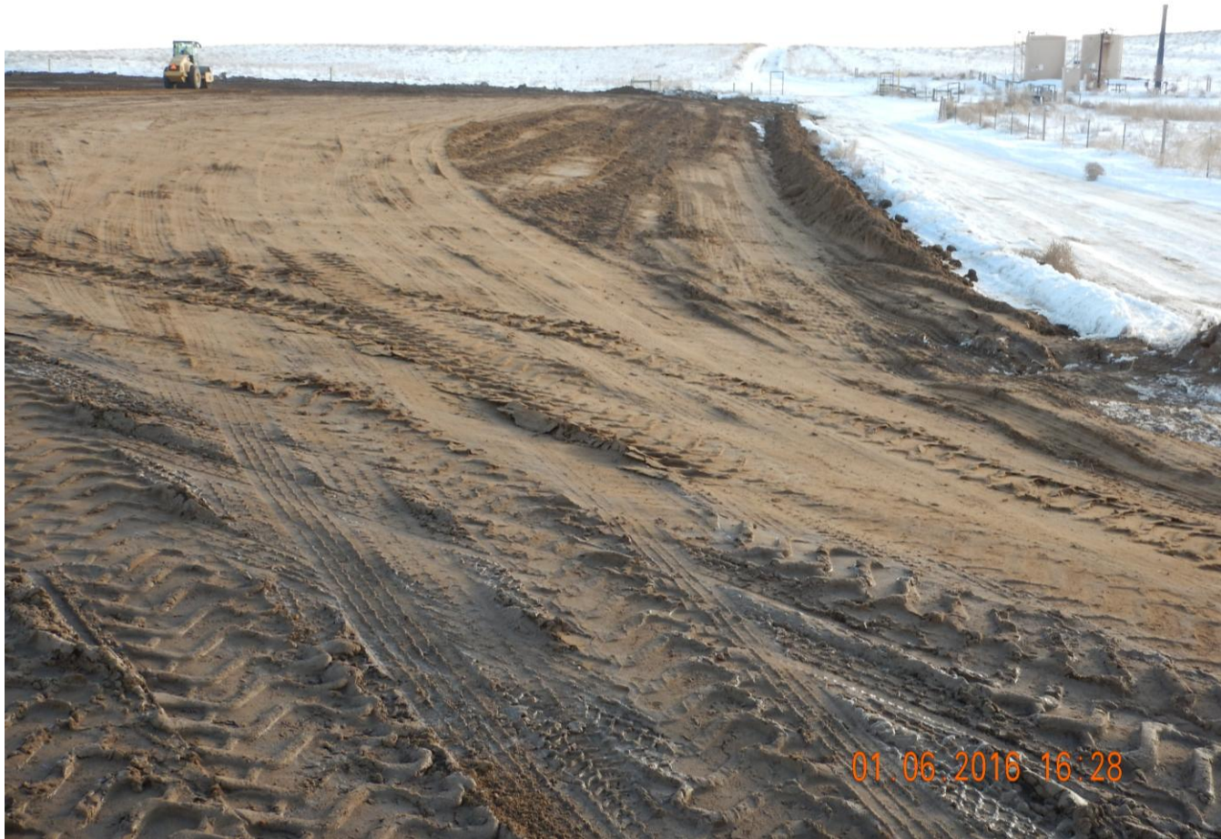
Photo 1. Photo taken from northwest location, facing South. Stormwater BMPs installed in center of photo.
