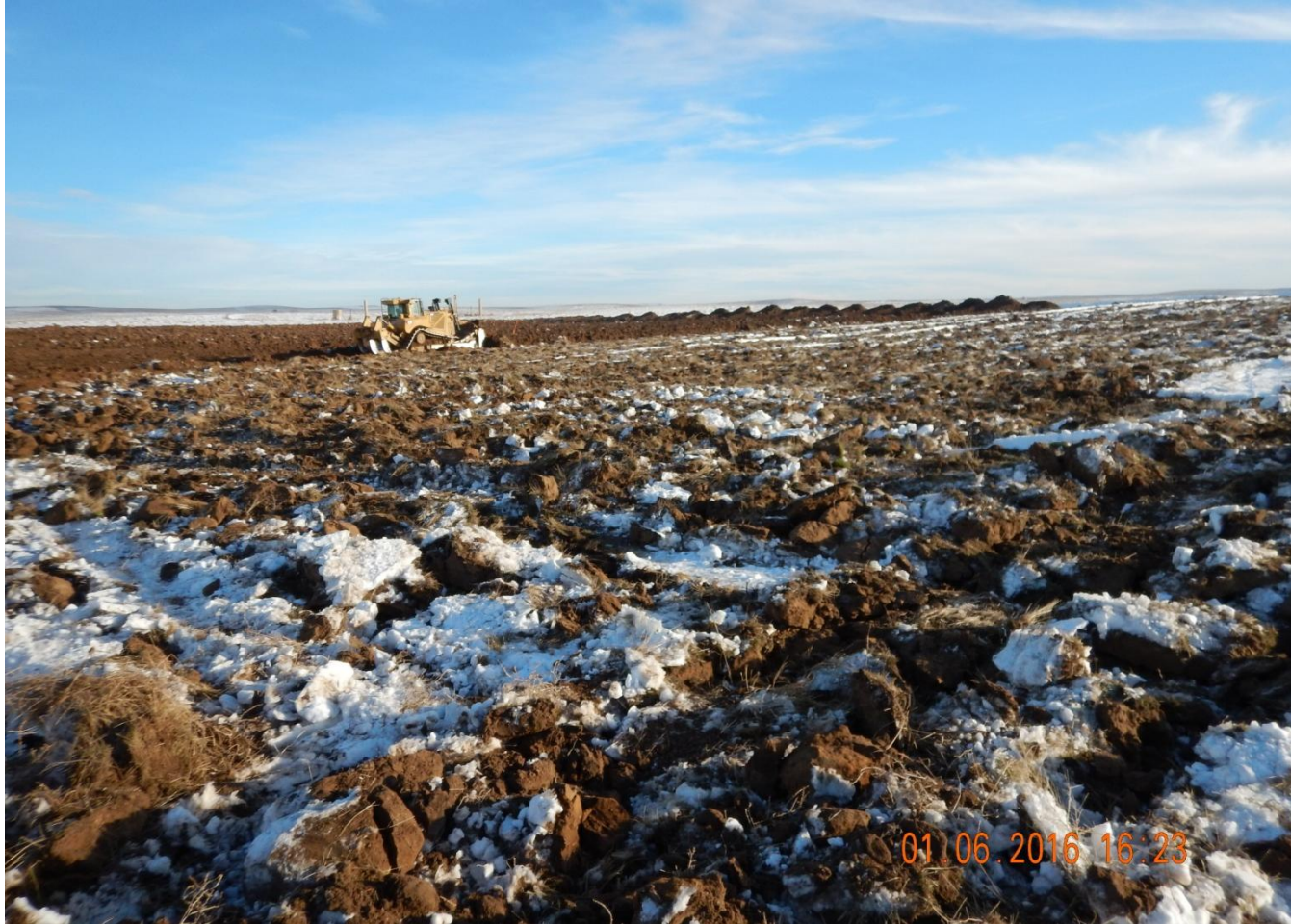
Photo 6. Photo taken from northwest location, facing Southeast. Topsoil salvage in process.
