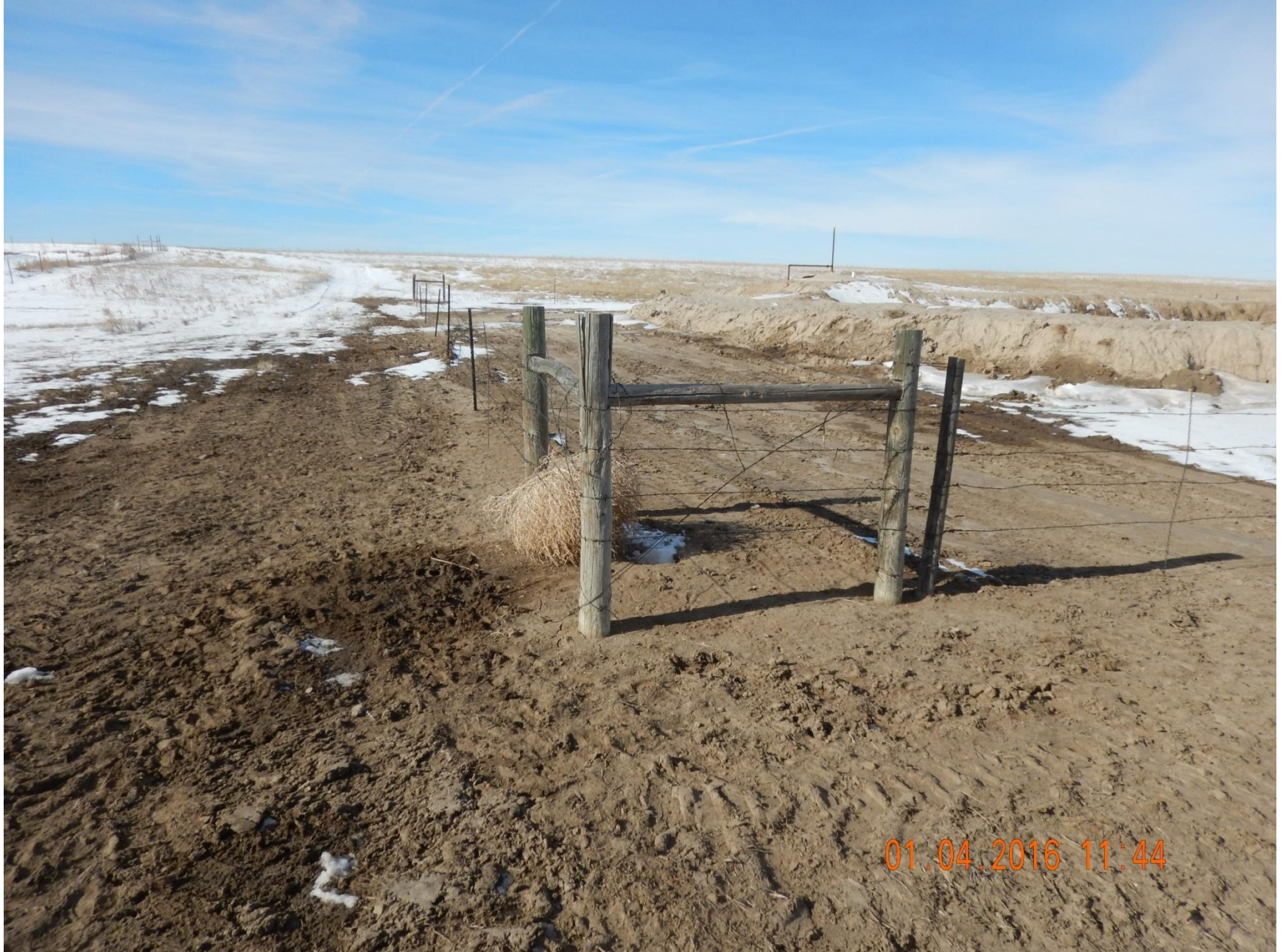
Figure 10: Photo taken southeast end of pit location, facing west. Photo shows stormwater and sediment control BMPs have not been installed.
