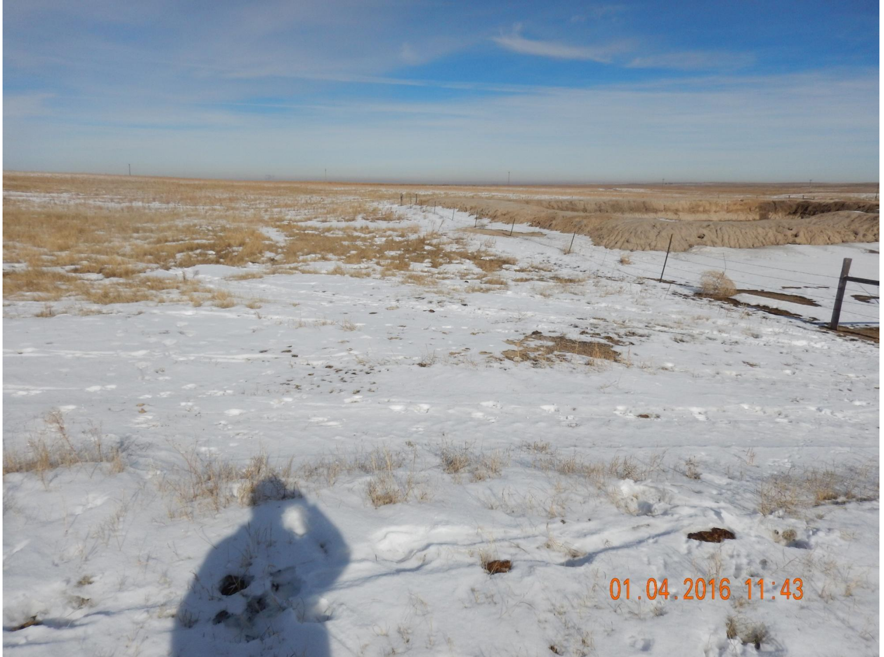
Figure 8: Photo taken from southwest of pit location, facing north. Photo shows stormwater and sediment control BMPs have not been installed.
