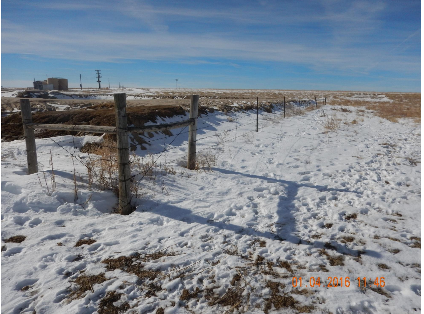
Figure 13: Photo taken northeast end of pit location, facing west. Photo shows stormwater and sediment control BMPs have not been installed.
