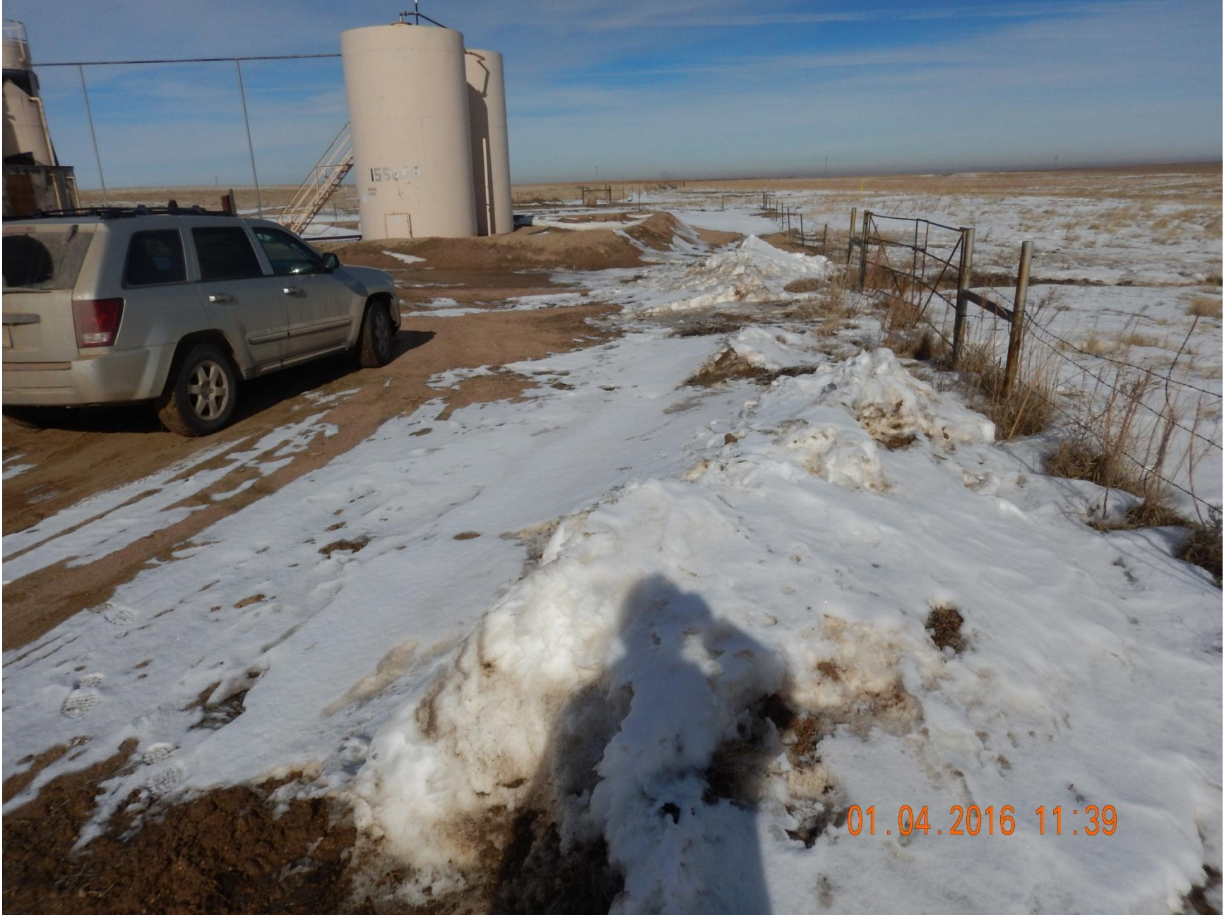
Figure 2: Photo taken from east end of location facing north. Photo shows stormwater and sediment control BMPs have not been installed.
