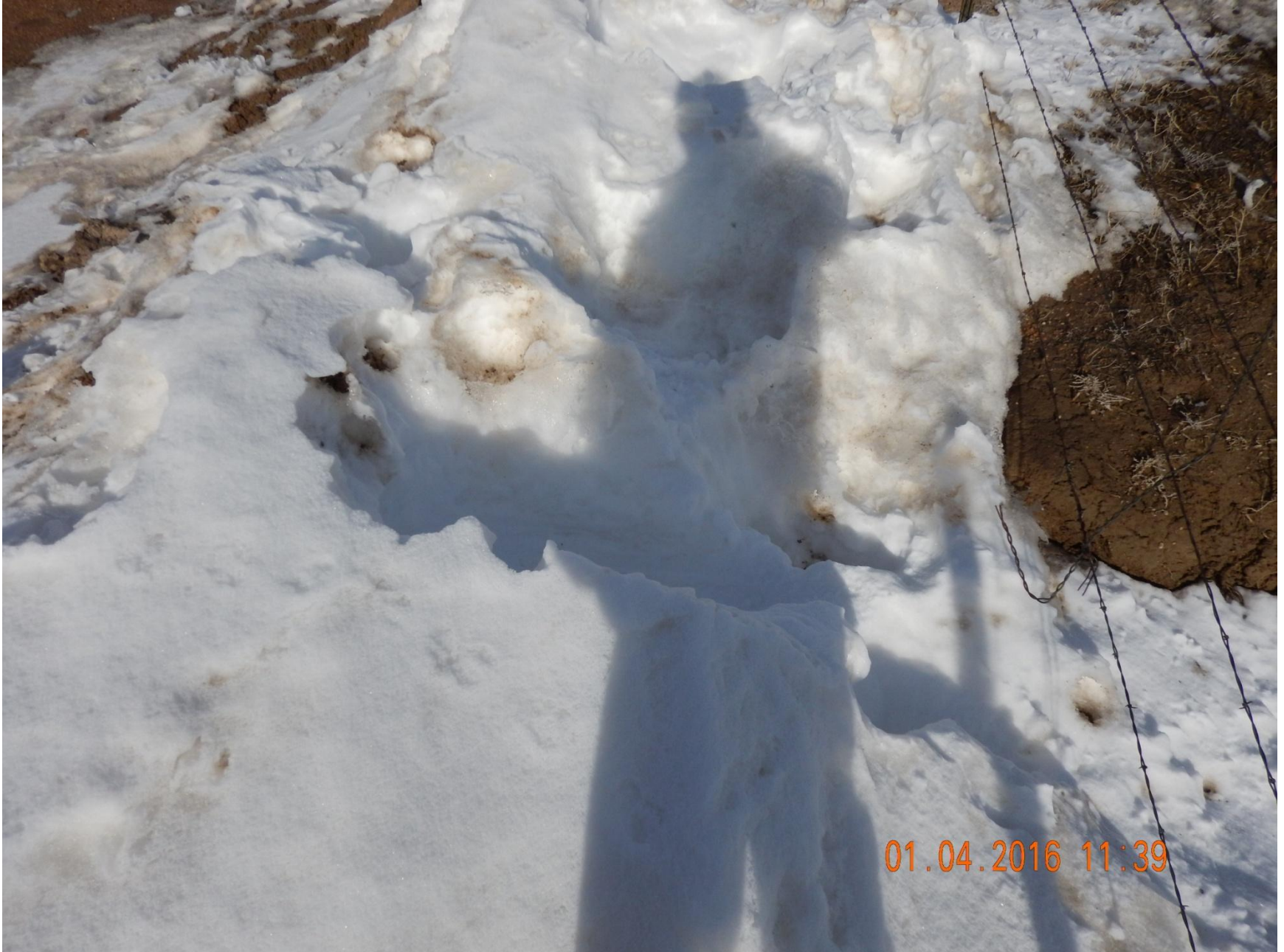
Figure 3: Photo taken from east end of location. Initially though pile was a berm installed for stormwater management. After digging it was determined berm was a snow stock pile, not a stormwater and sediment control BMP.
