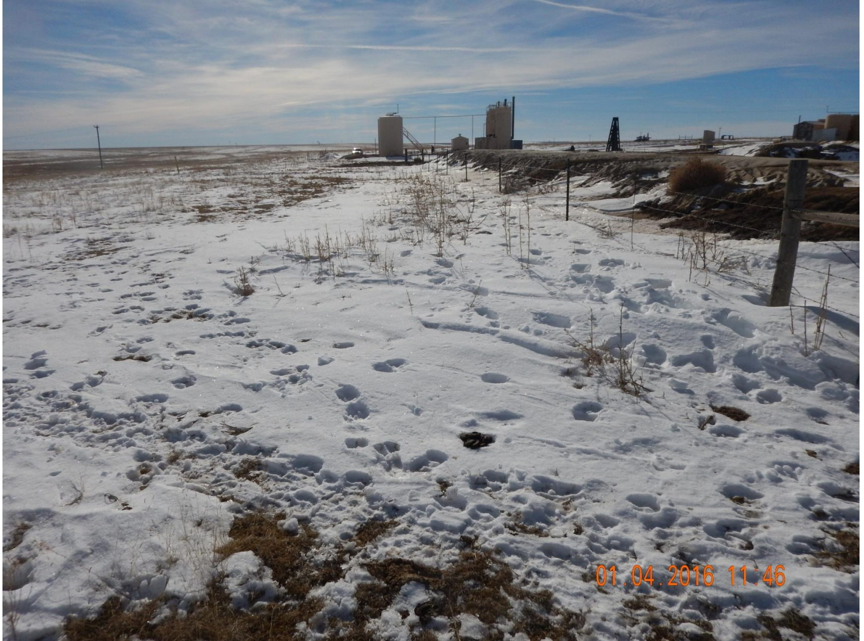
Figure 12: Photo taken from northeast end of pit location, facing south. Photo shows stormwater and sediment control BMPs have not been installed.
