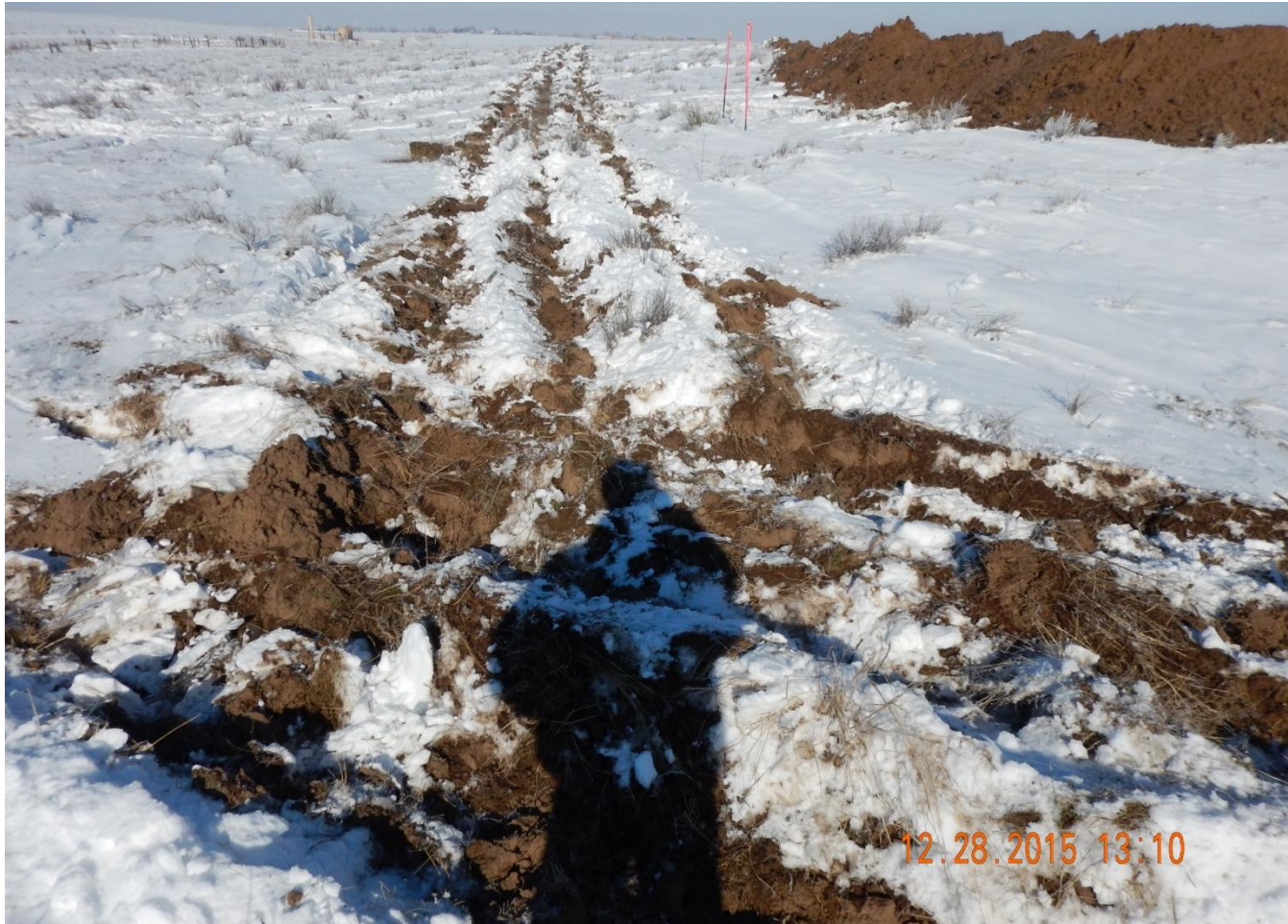
Photo 1. Photo taken from southwest location, facing North. Surface water drainage located cross- and down-gradient from disturbance (Refer to photo 8). Surface roughening (ripping) is a temporary BMP and should be used in conjunction with other BMPs. Western edge of disturbance should incorporate additional BMPs because of surface water drainage.
