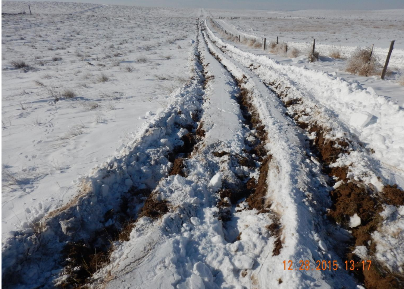
Photo 5. Photo taken from northeast location, facing West. Surface roughening (ripping) is a temporary BMP. May need additional stormwater BMPs because of surface water drainage located cross- and down-gradient from disturbance.
