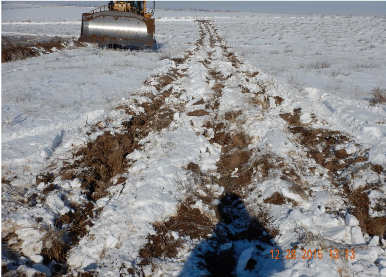
Photo 4. Photo taken from southeast location, facing North. Surface roughening (ripping) is a temporary BMP. May need additional stormwater BMPs because of surface water drainage located cross- and down-gradient from disturbance.
