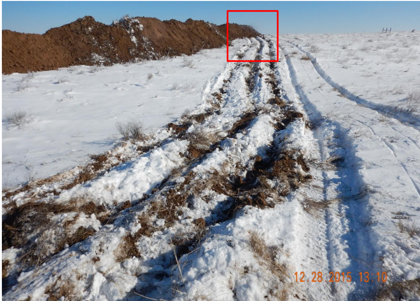
Photo 2. Photo taken from southwest location, facing East. Surface water drainage located cross- and down-gradient (Refer to photo 8). Surface roughening (ripping) is a temporary BMP and should be used in conjunction with other BMPs. Southern edge of disturbance should incorporate additional BMPs because of surface water drainage. Do not fill or drive over stormwater BMPs. Operator fixed issue while I was onsite. Refer to photo 7.
