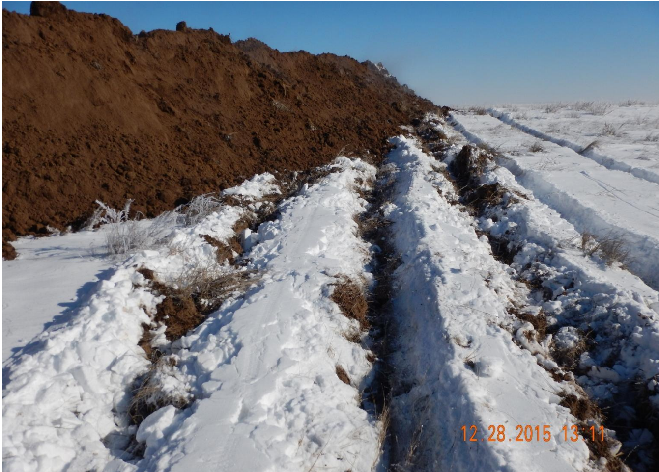
Photo 3. Photo taken from southern location, facing East. Do not fill or drive over stormwater BMPs. Operator fixed issue while I was onsite. Refer to photo 7.
