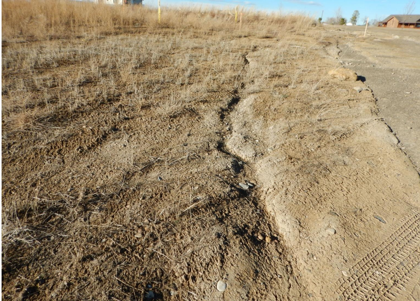
Photo 4. Photo taken from northern entrance, facing North. Need to stabilize and control erosion.
