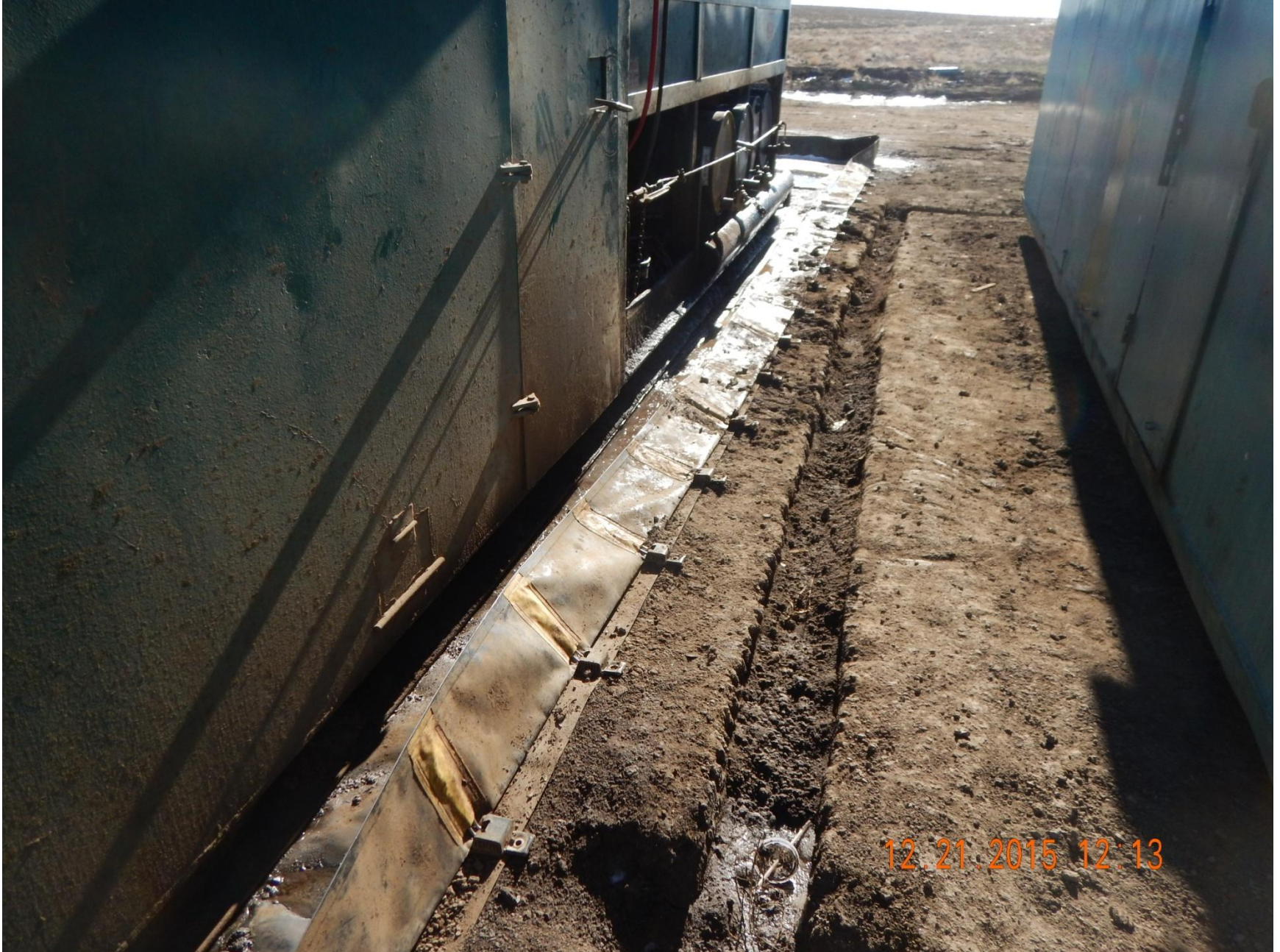
Figure 18: Photo taken at tanks on the south end of location. Photo shows containment BMP not properly functioning.
