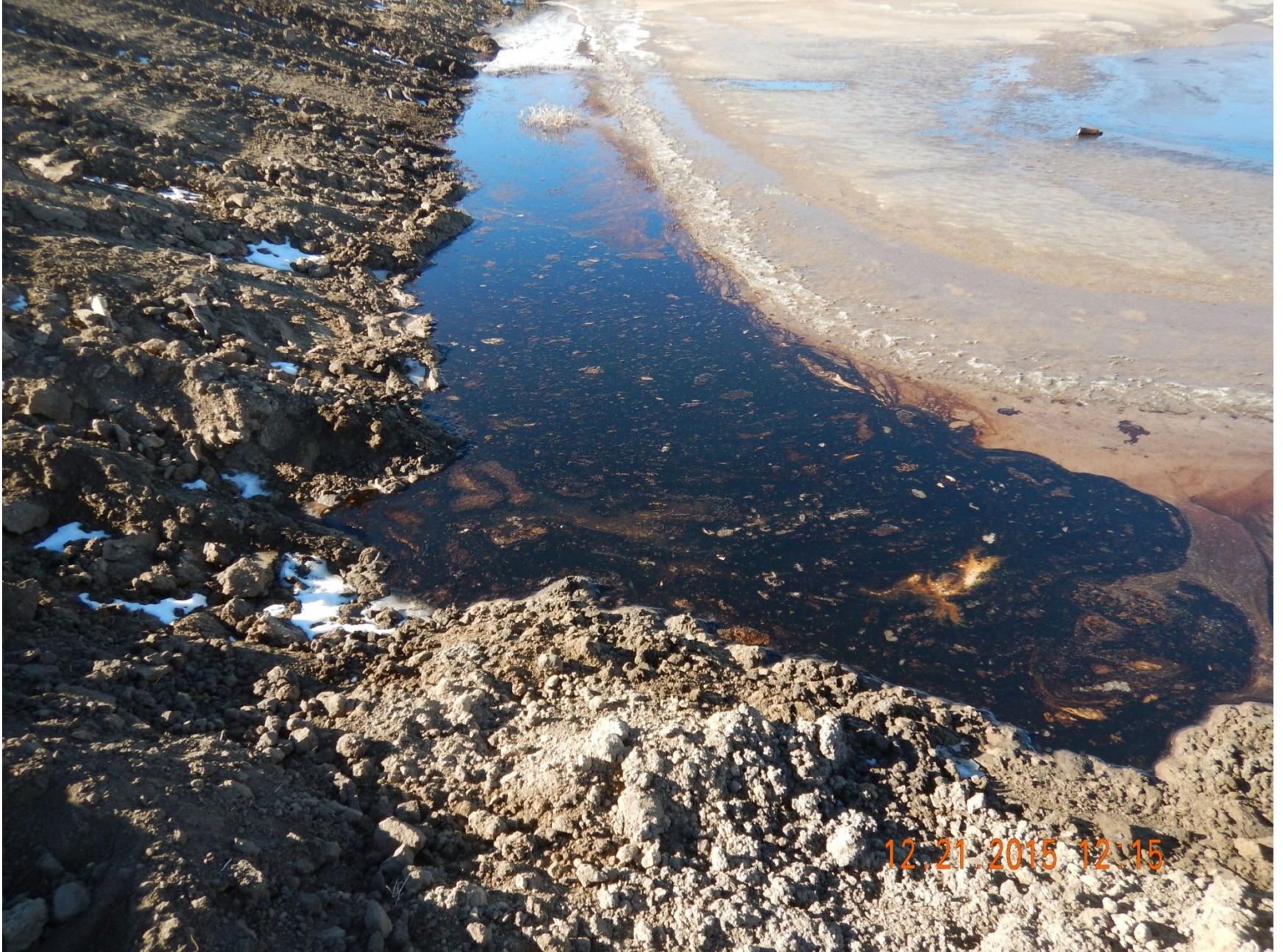
Figure 16: Photo taken at southern pit. Photo shows oily water. Pit does not appear to be lined.
