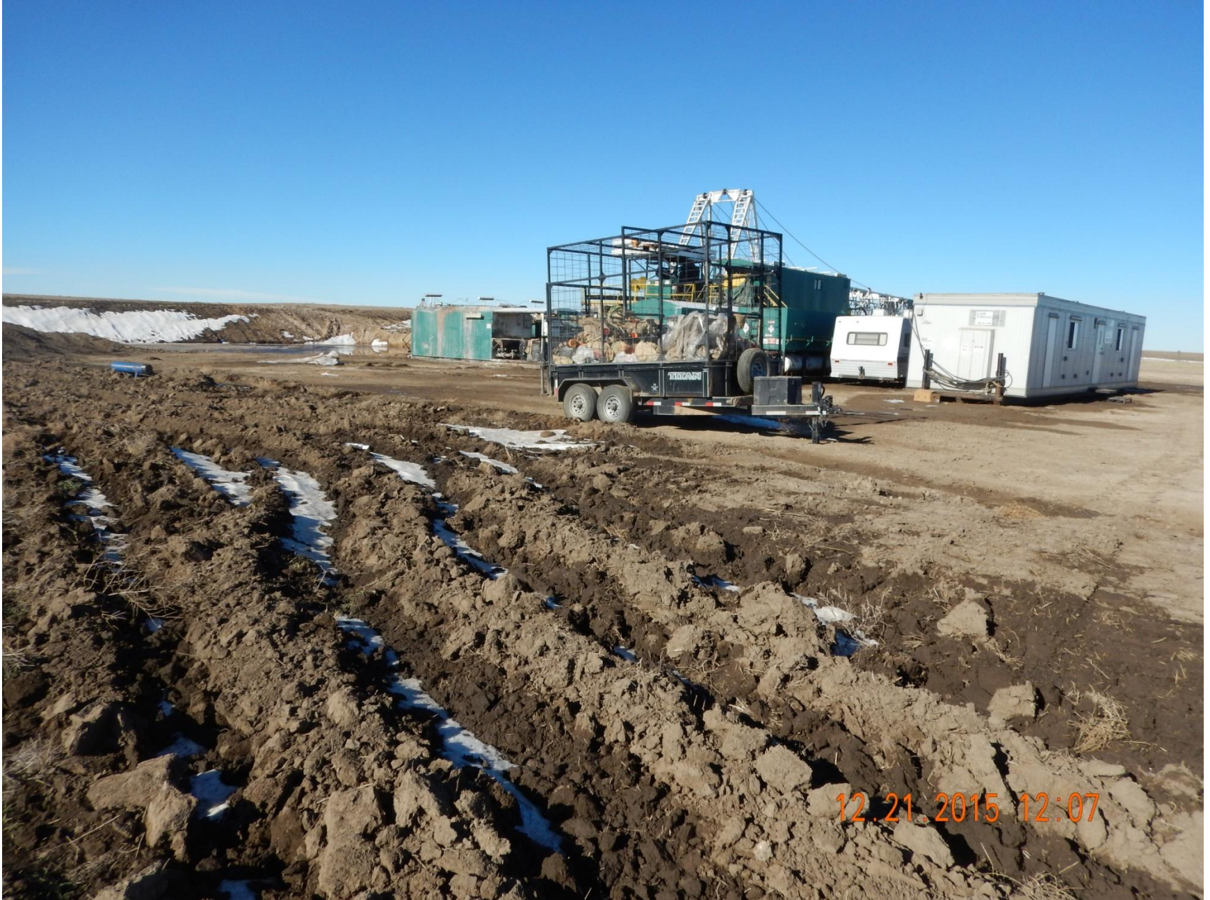
Figure 5: Photo taken from southeast end of location, facing northwest. Photo shows caged-trailer used for debris management. Note door to cage not properly shut.
