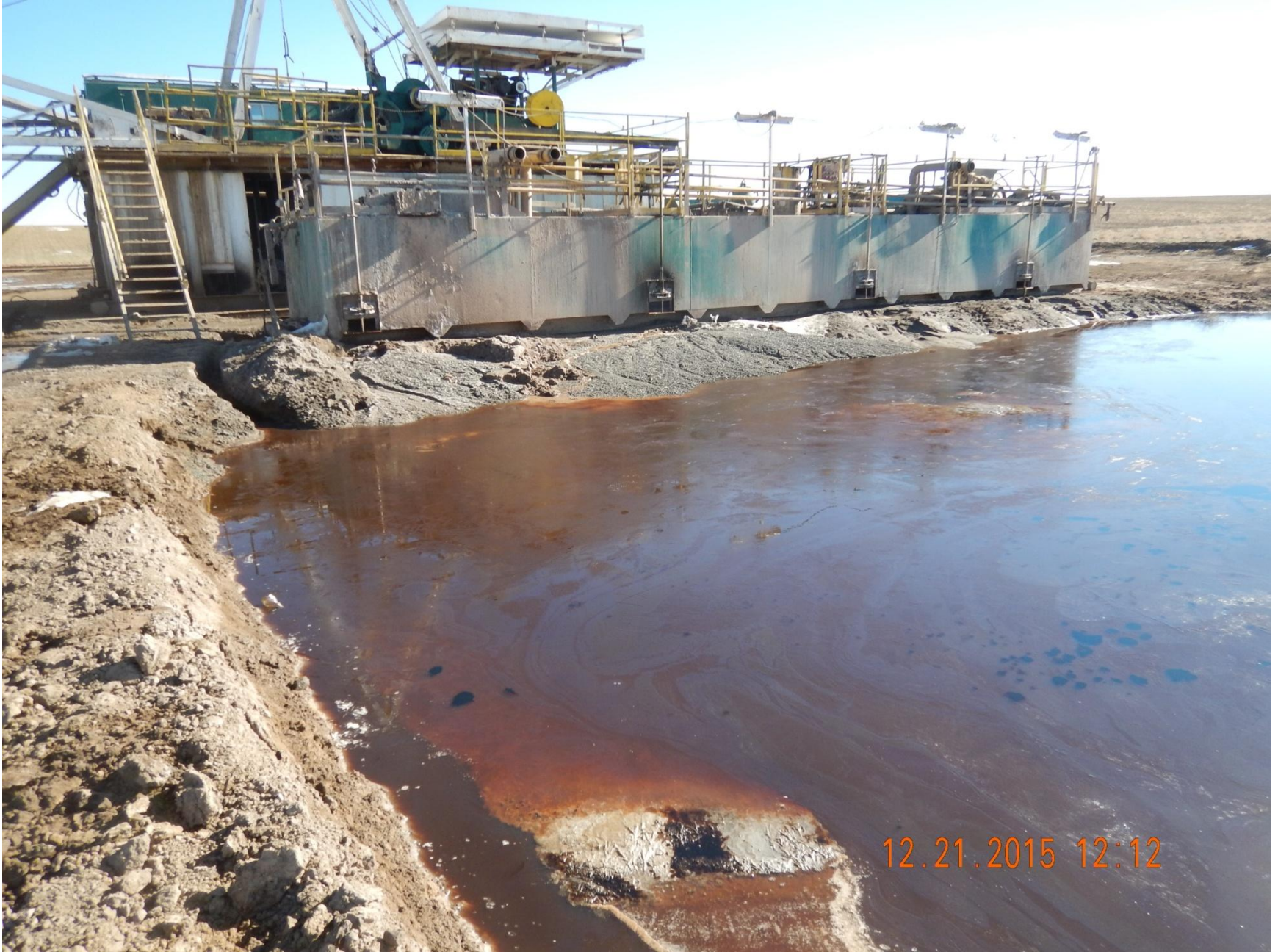
Figure 13: Photo taken at southern pit. Photo shows oily water. Pit does not appear to be lined.
