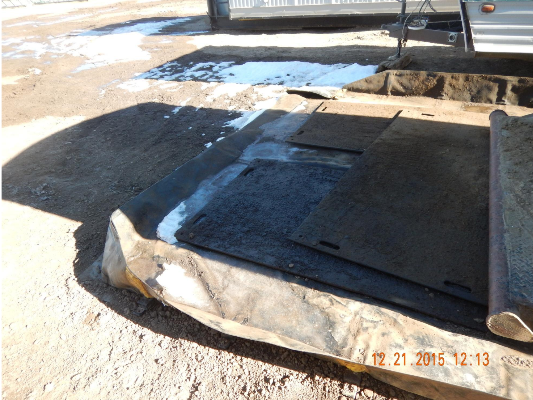
Figure 17: Photo taken at tanks on the south end of location. Photo shows containment BMP not properly functioning.
