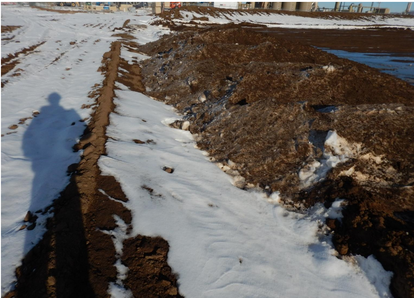
Photo 3. Photo taken from western location, facing North. DO NOT scrape sediment into stormwater ditches. Stormwater ditches need to be maintained.
