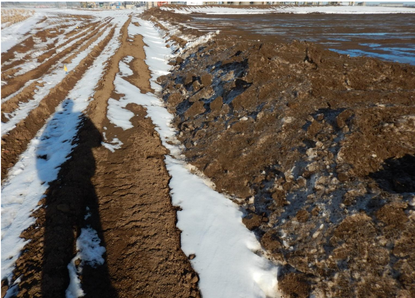
Photo 2. Photo taken from western location, facing North. DO NOT scrape sediment into stormwater ditches. Stormwater ditches need to be maintained.
