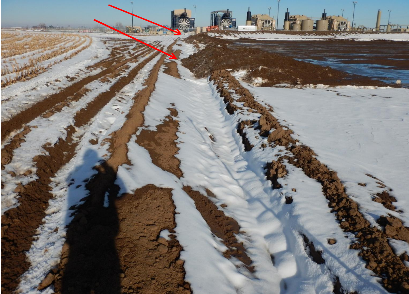
Photo 1. Photo taken from western location, facing North. Stormwater BMP installed in center of photo. DO NOT scrape sediment into stormwater ditches. Stormwater ditches need to be maintained. Refer to close up photos 2-3.
