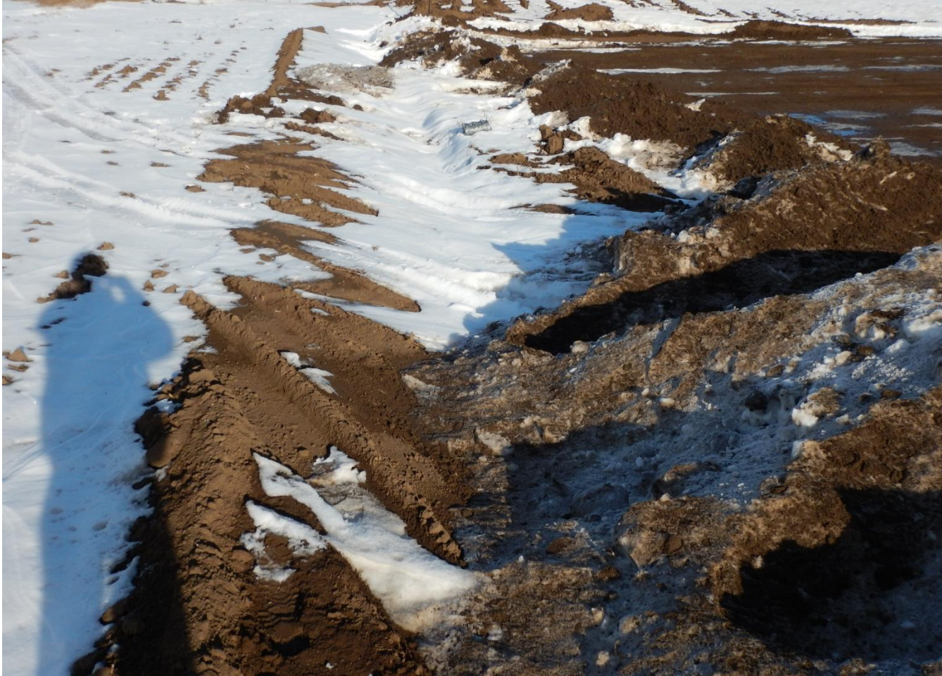
Photo 4. Photo taken from western location, facing North. Only access/exit southern main location. Western vehicle traffic is damaging stormwater ditches. Stormwater ditches need to be maintained.
