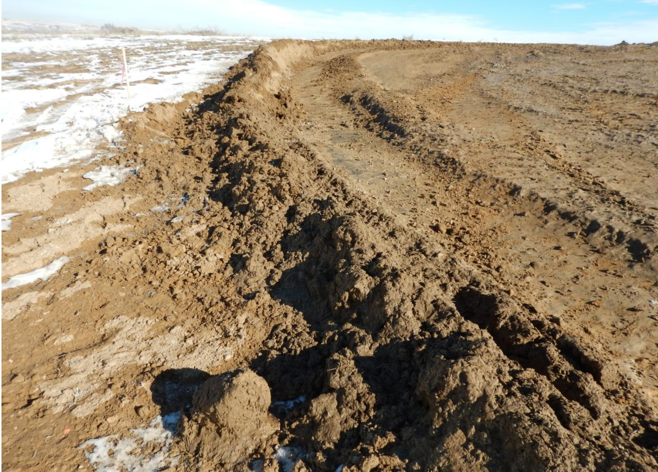
Photo 6. Photo taken from northwestern area of west drill pad, facing North. Stormwater BMPs have not been installed prior to construction.
