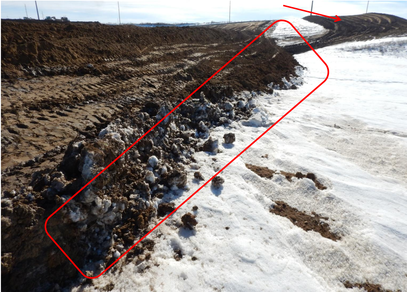
Photo 5. Photo taken from western area of west drill pad, facing South. Topsoil stockpile towards the right of the picture. Stormwater BMPs have not been installed prior to construction.
