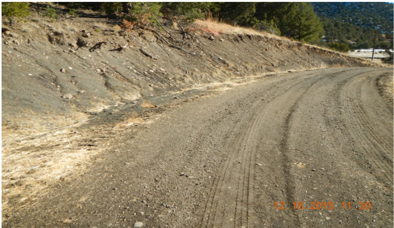
Photo 4: Facing east towards access road.
