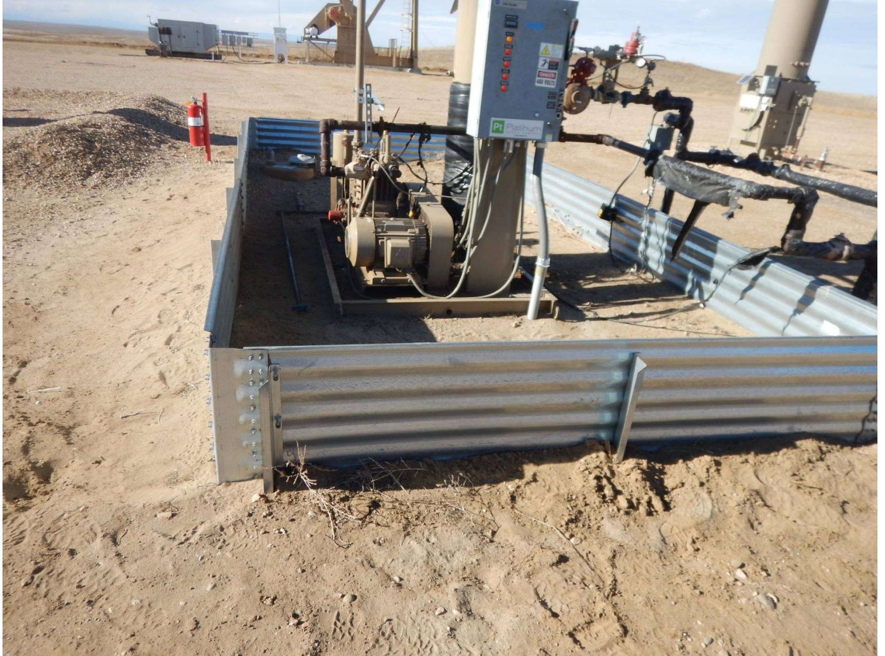
Figure 1: Photo of repaired containment BMP.
