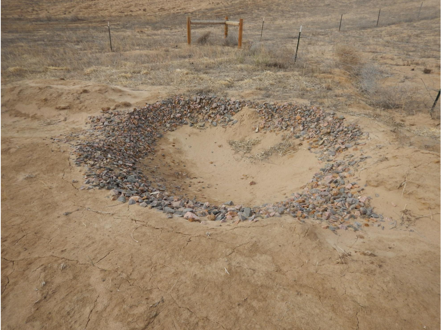
Figure 25: Photo taken from the northwest end of location. Photo of sediment trap BMP.
