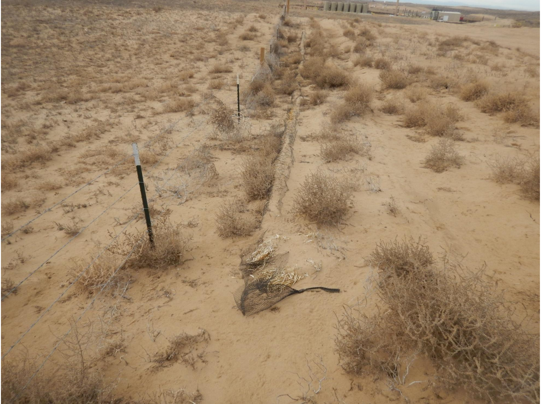
Figure 9: Photo taken from south end of location, facing west. Photo shows stormwater and sediment control BMP in disrepair.
