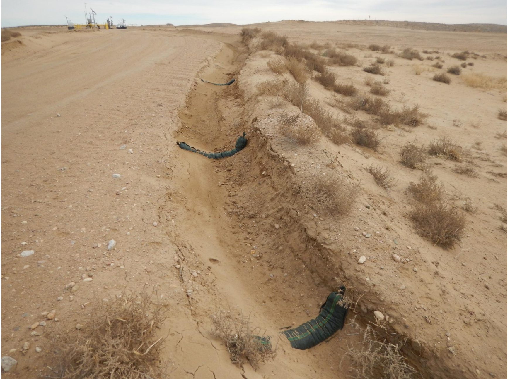
Figure 2: Photo taken from southwest end of location, facing east. Photo of stormwater and sediment control BMP on access road. Photo shows sediment filling, and flowing over BMPs.
