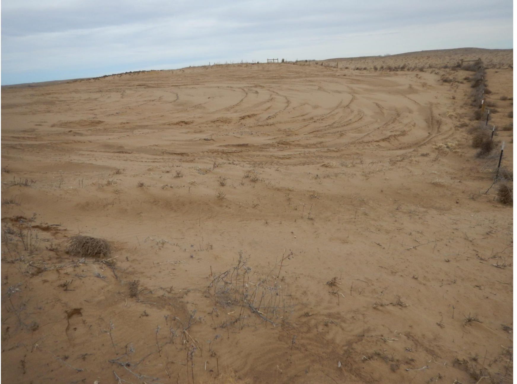
Figure 11: Photo taken from southeast end of location, facing east. Photo shows insufficient stormwater and sediment control BMPs on interim area.
