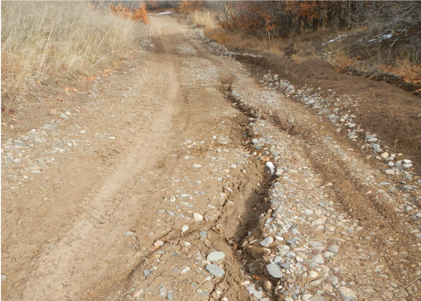
Photo 5. View of access road near well pad entrance facing northward. Stormwater erosion is occurring on the access road surface.
