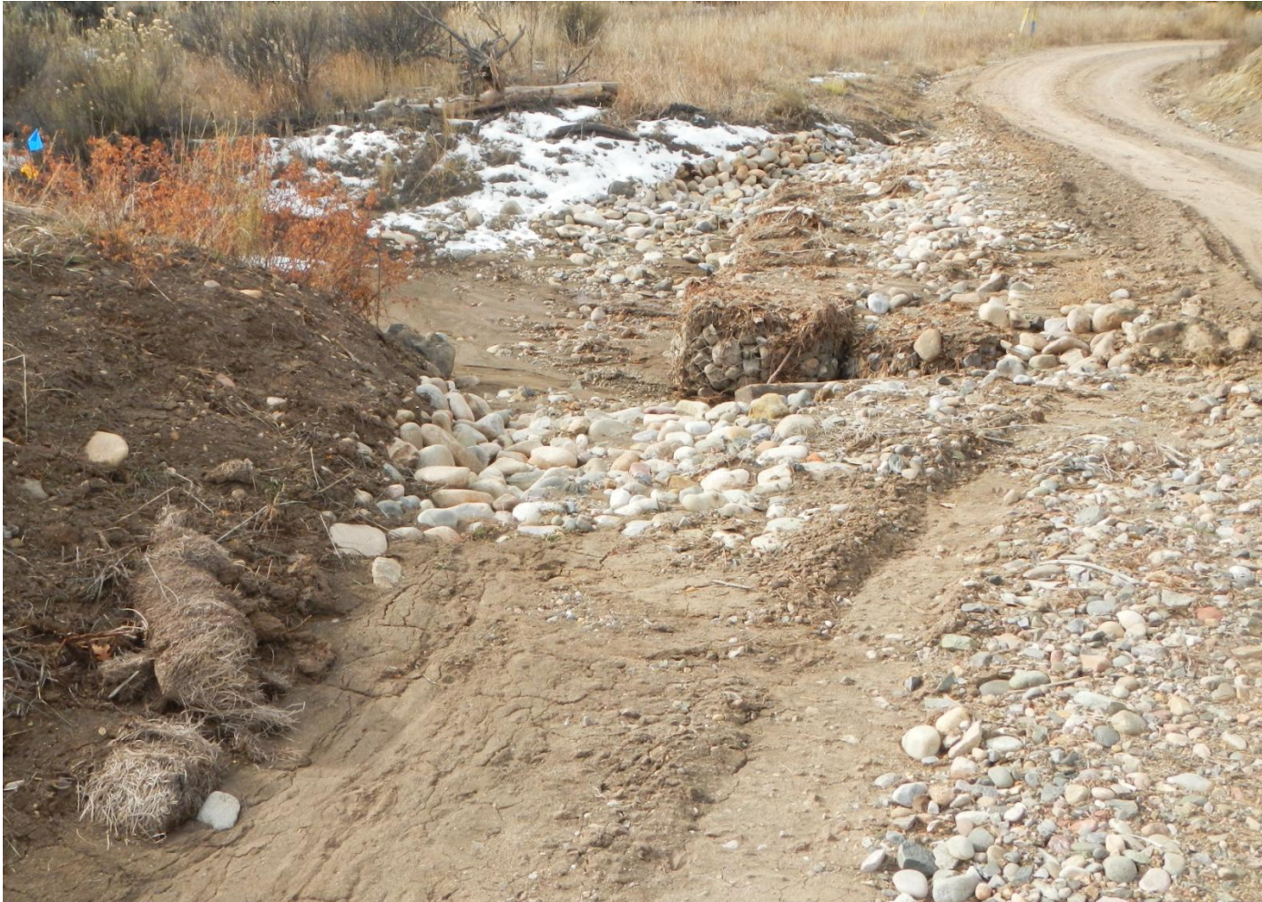
Photo 1. View of downstream portion of the low water crossing along Budd Road. A dilapidated straw wattle is present on the left hand side of photo and erosion is occurring where stormwater flows around the gabions and erodes at the edges.
