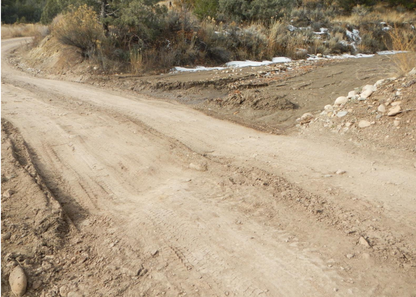
Photo 2. View of upstream portion of the low water crossing along Budd Road. Sediment deposits indicate that the bottom of the upstream channel are approximately 4-5 inches higher than the elevation at the crossing. This indicates that the low water crossing likely fills with sediment during storm events and becomes impassable.
