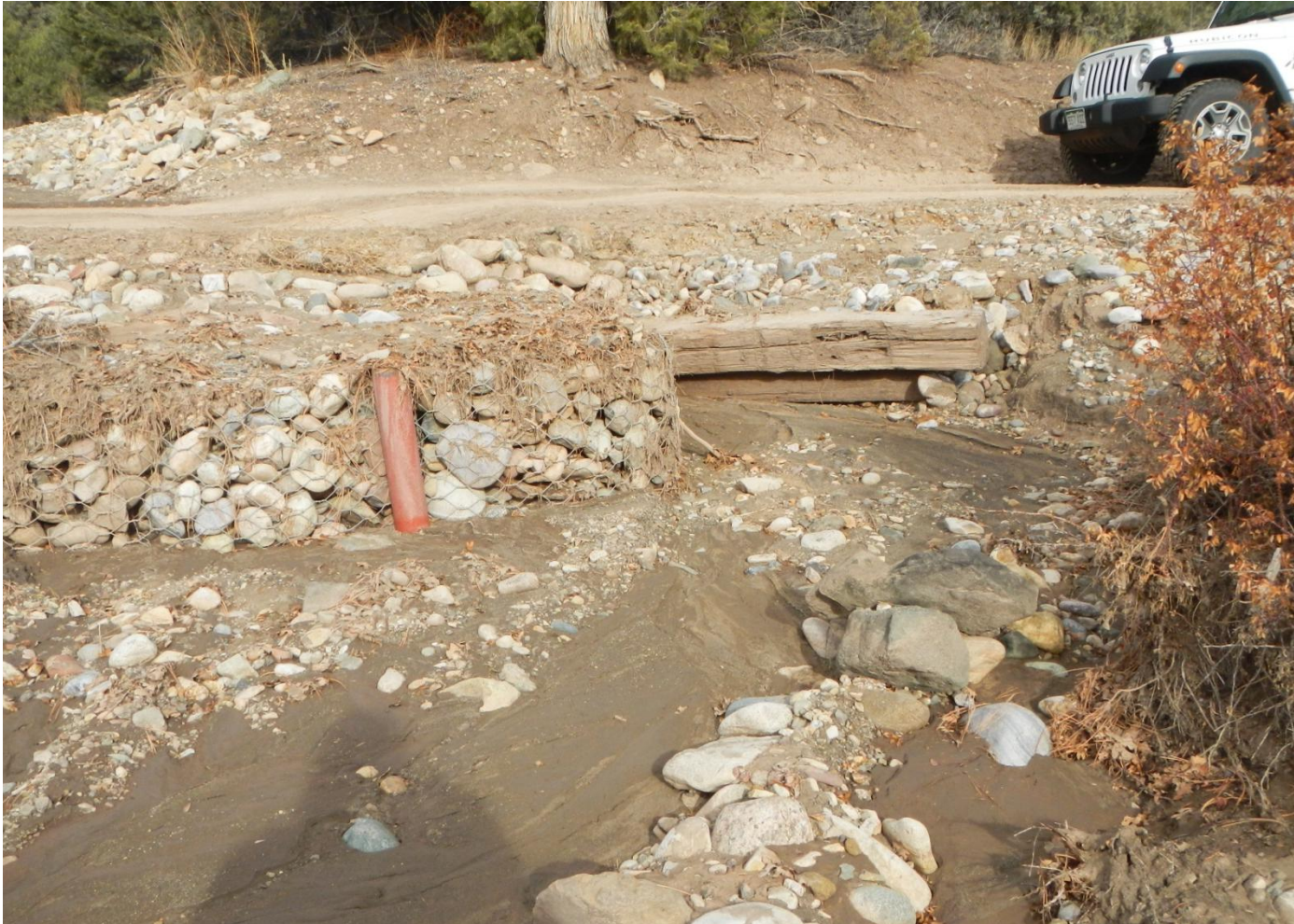
Photo 4. View of area where stormwater flows are eroding around gabions facing upstream toward crossing.
