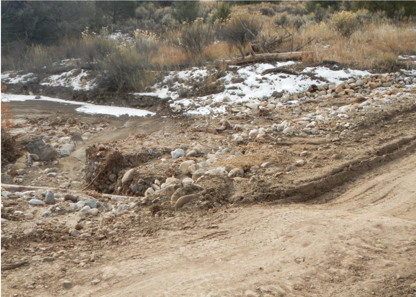
Photo 3. View of area where stormwater flows over the road and erodes the edges of the gabions facing downstream.
