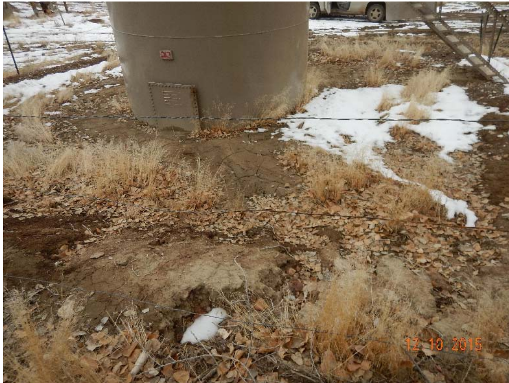
Stormwater moving into berm containment
