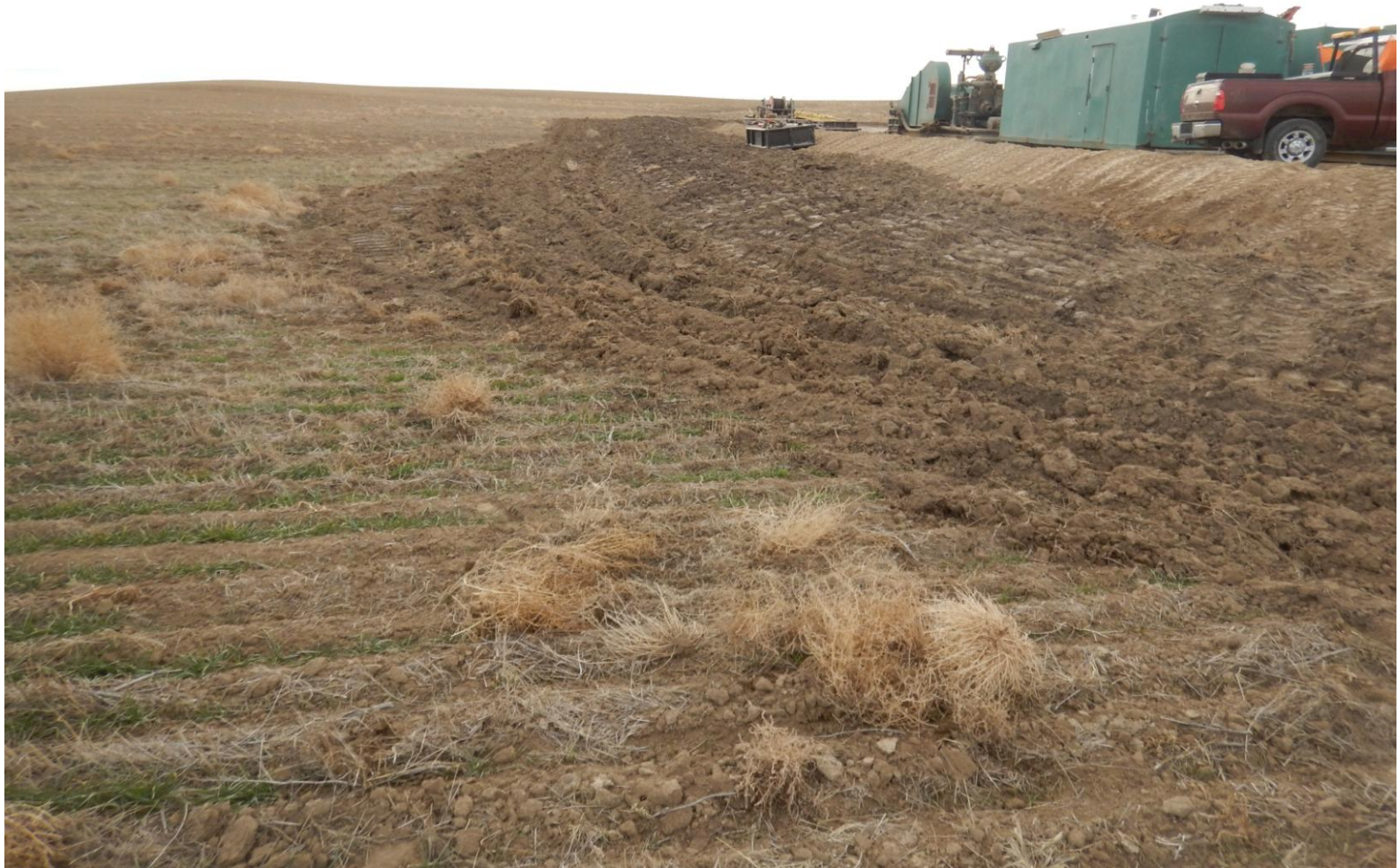
Figure 8: Photo taken from the northeast portion of location, facing south. Photo shows surface roughening (sediment control BMP).
