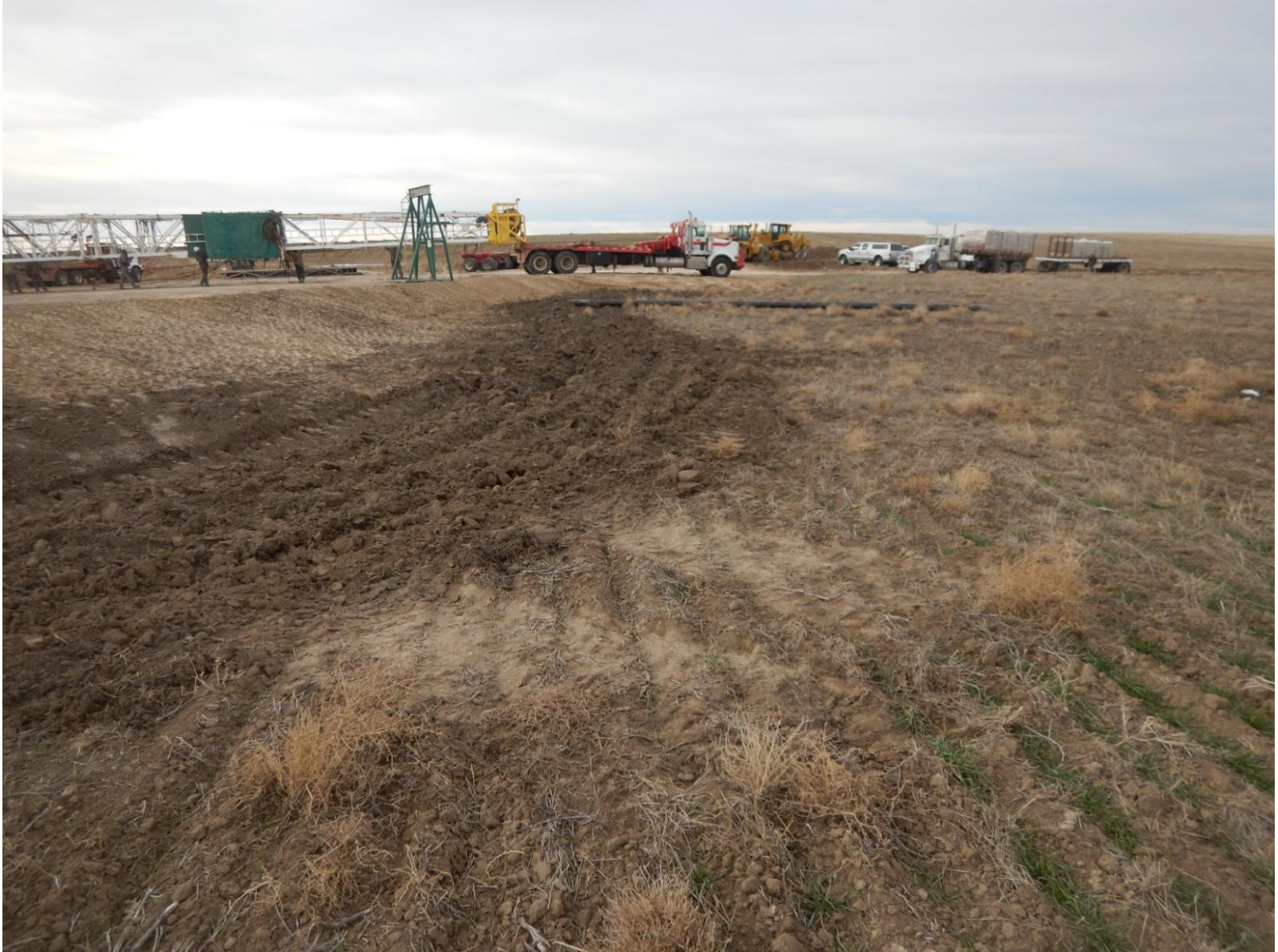
Figure 9: Photo taken from Northeast portion of location, facing west. Photo shows surface roughening (sediment control BMP). Photo shows equipment (appears to be a large pipe), placed off of location.
