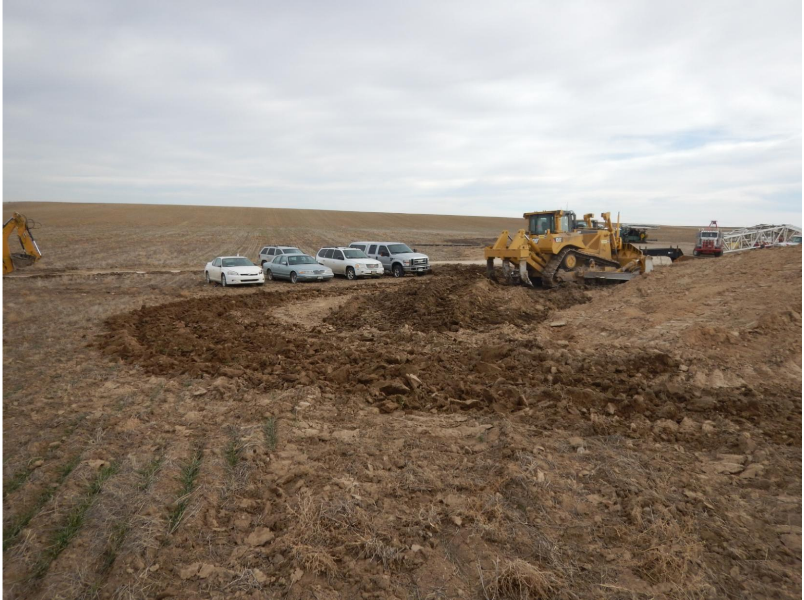
Figure 5: Photo taken from Northwest portion of location, facing east. Photo shows topsoil berm (right of photo), surface roughening (sediment control BMP) and construction in process.
