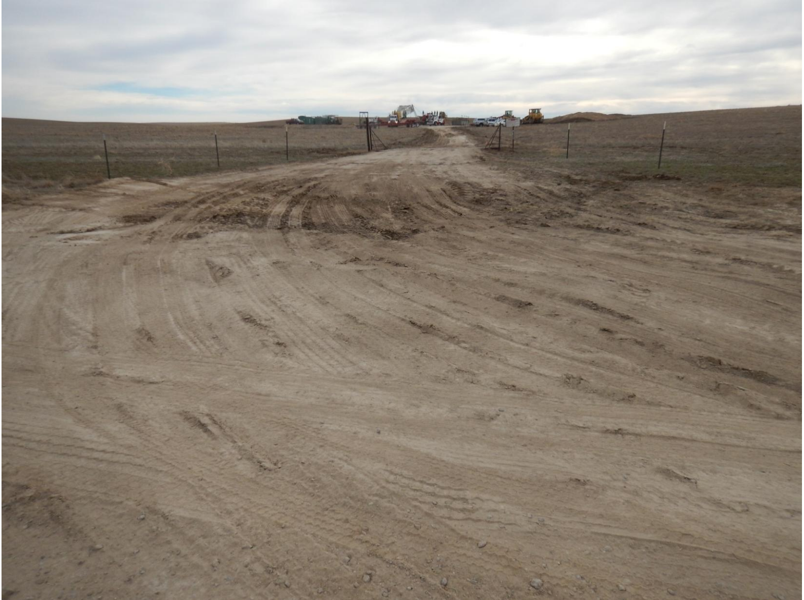
Figure 3: Photo taken from County Rd. 0 facing south towards location. Photo shows inadequate stormwater BMPs for site's access road.
