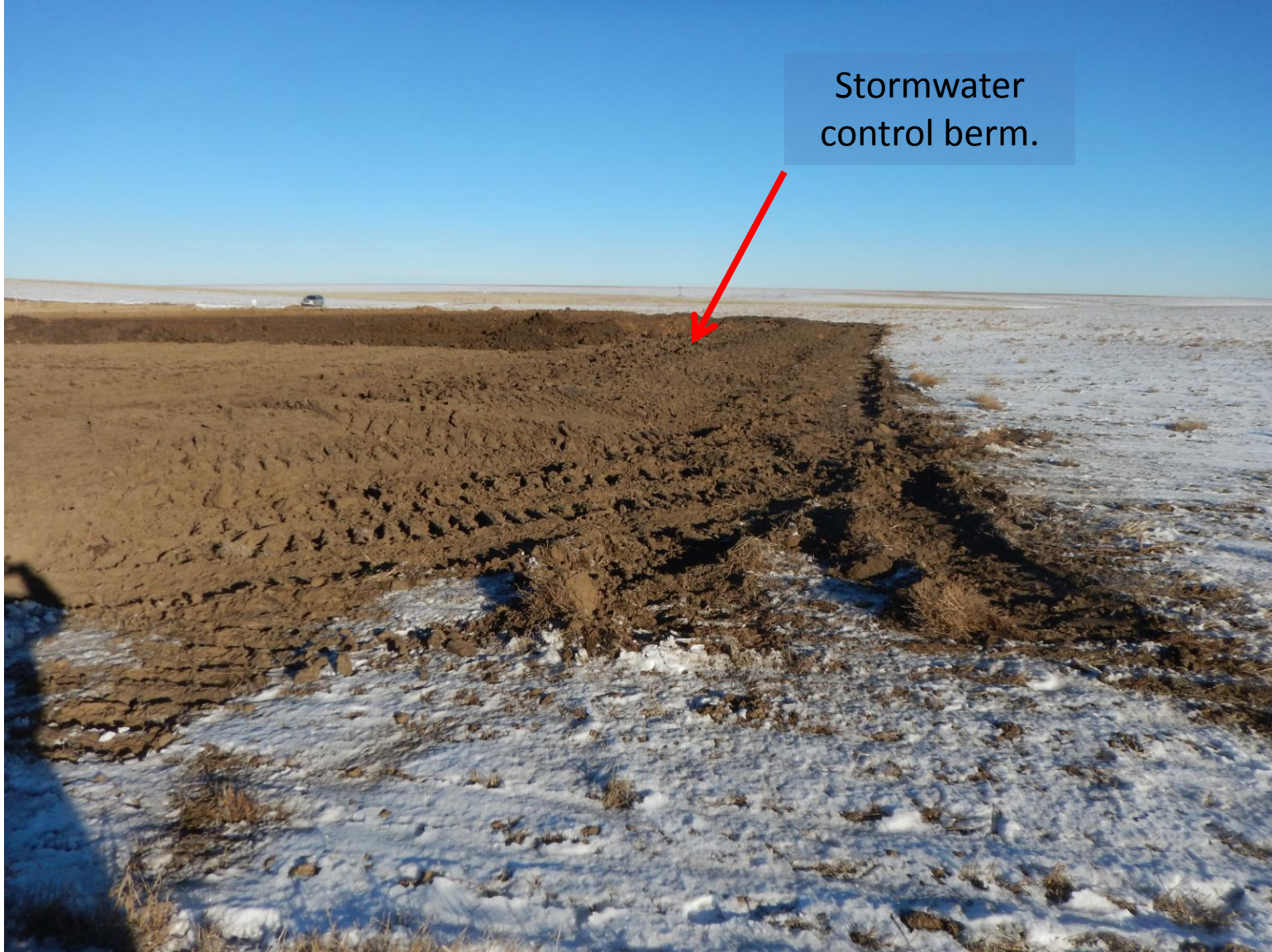
Figure 13: Photo taken from southeast corner of location, facing north. Photo of stormwater diversion berm on east end of location as per operator BMP.
