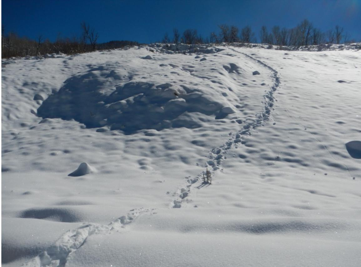
Photo #1: Cut Slope subsidence / sloughing.
