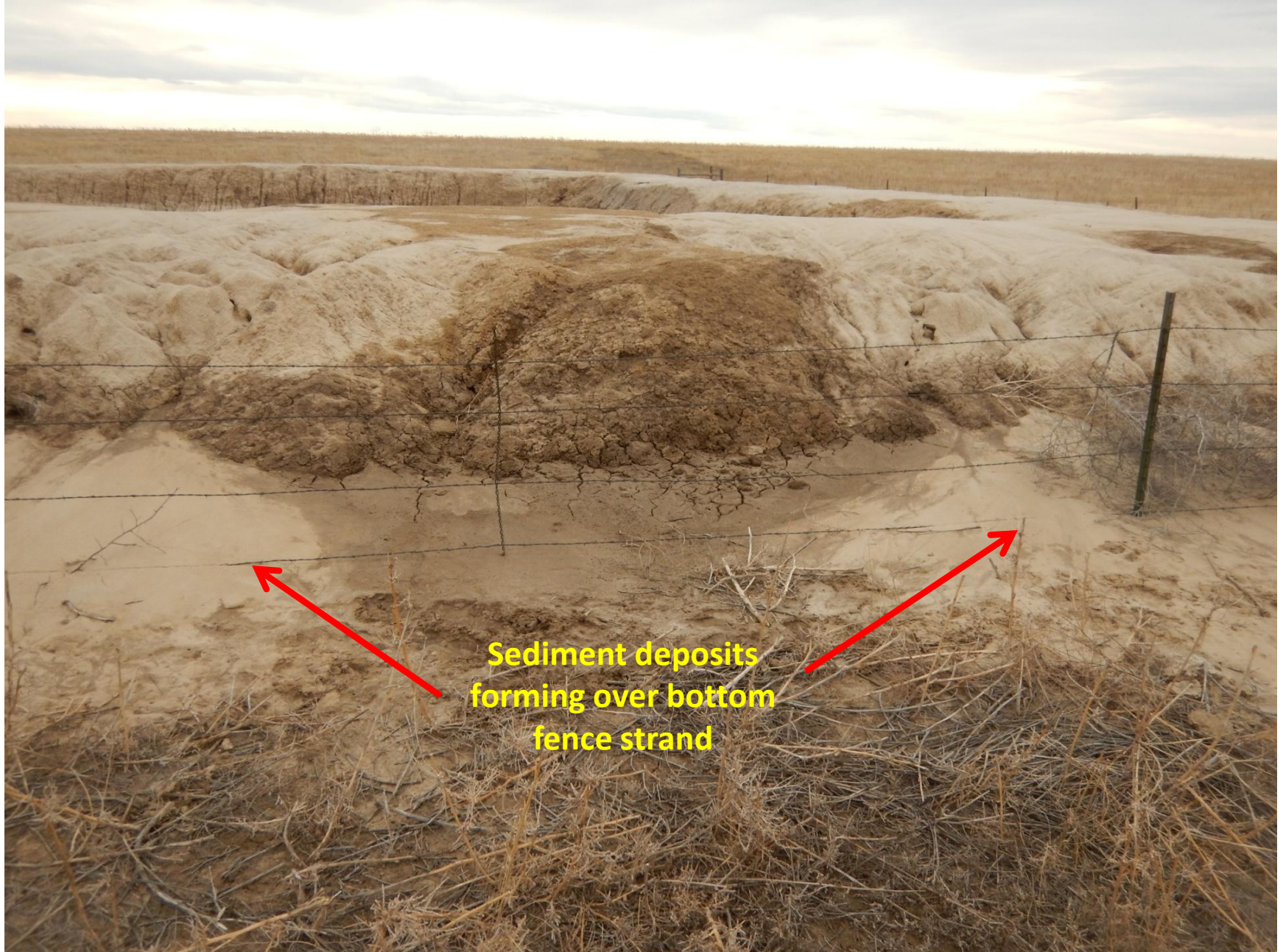
Figure 18: Photo taken from east end of pit location. Photo shows stormwater erosion on pit's containment berm, sediment deposition off of location, and insufficient stormwater BMPs.
