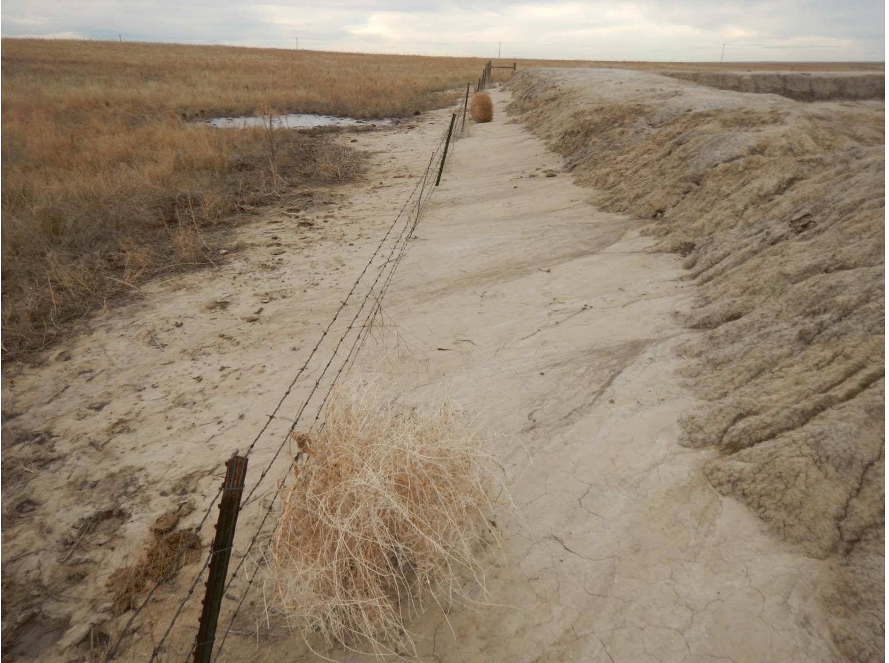
Figure 29: Photo taken from west end of pit location facing north . Photo shows stormwater deposition off of location, insufficient stormwater BMPs and weed debris.
