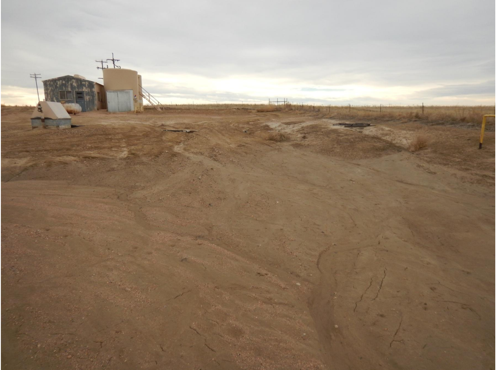
Figure 6: Photo taken from north end of location facing west. Photo shows surface erosion on location and insufficient stormwater BMPs.
