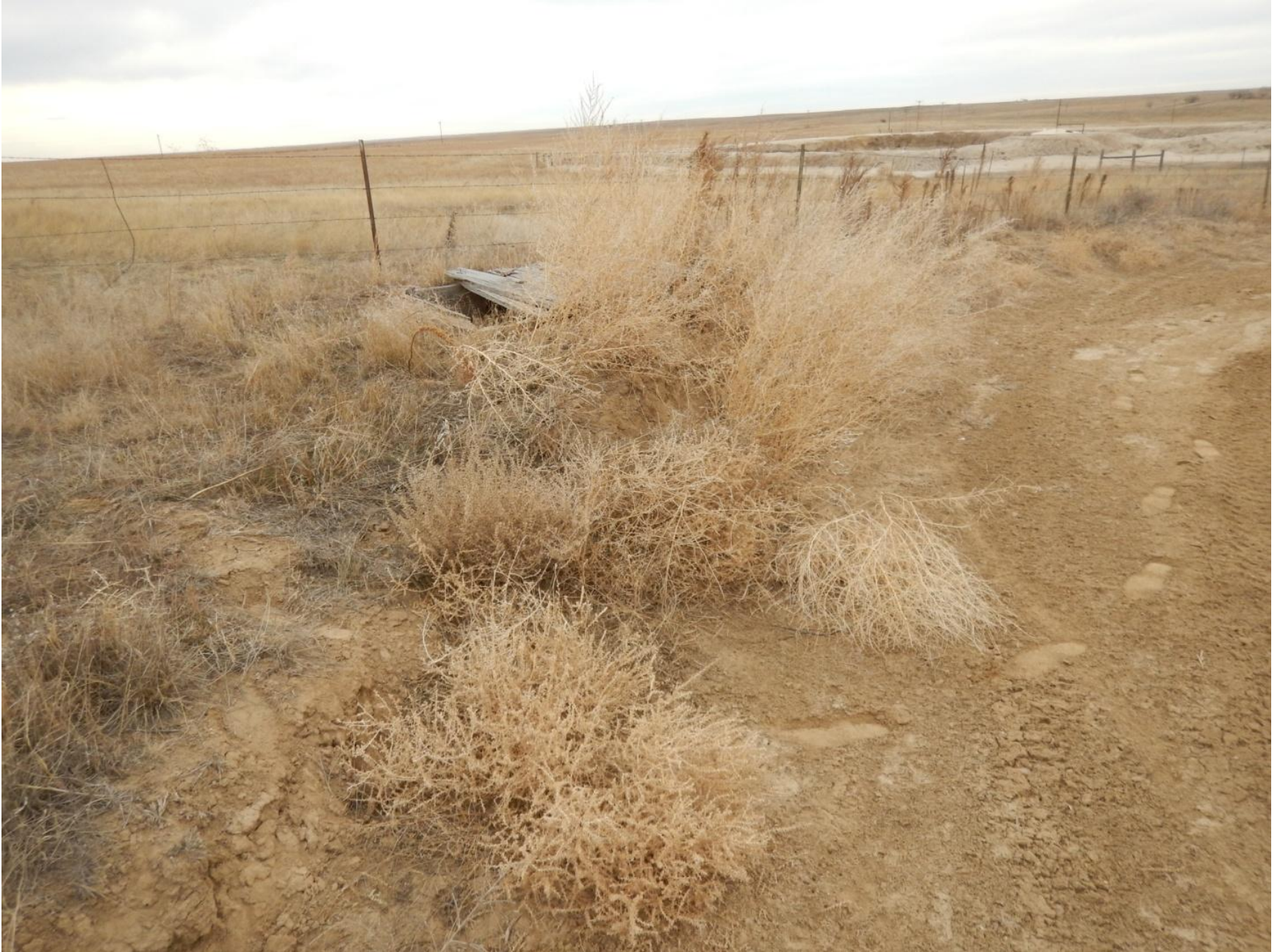
Figure 10: Photo taken from northwest end of location. Photo shows broken door of wooden sub-surface structure, and weed debris.
