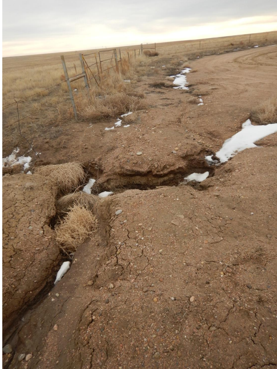
Figure 1: Photo taken from east end of location, facing north. Photo of gully formation. Note Russian thistle weed debris and insufficient stormwater BMPs.
