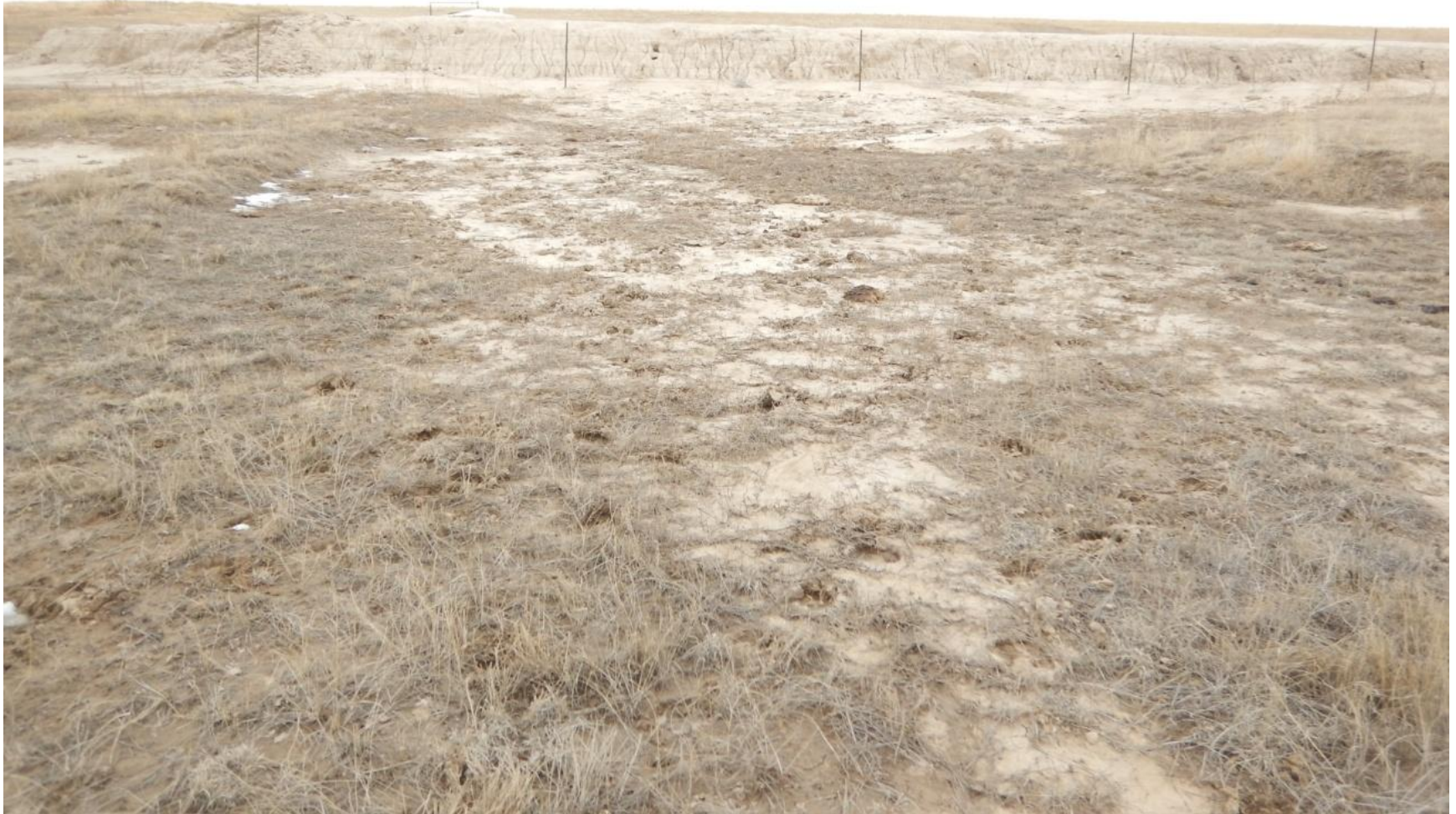
Figure 17: Photo taken from east of pit location facing west. Photo shows stormwater erosion on pit's containment berm, sediment deposition off of location, and insufficient stormwater BMPs.
