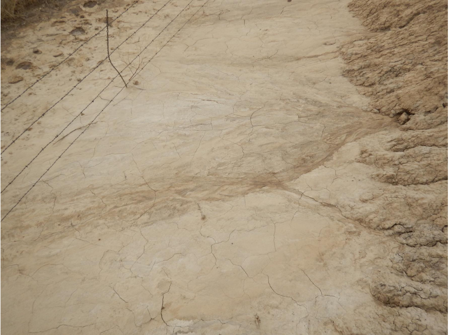
Figure 28: Photo taken from west end of pit location . Photo shows stormwater erosion on pit's containment berm and sediment deposition off of location.
