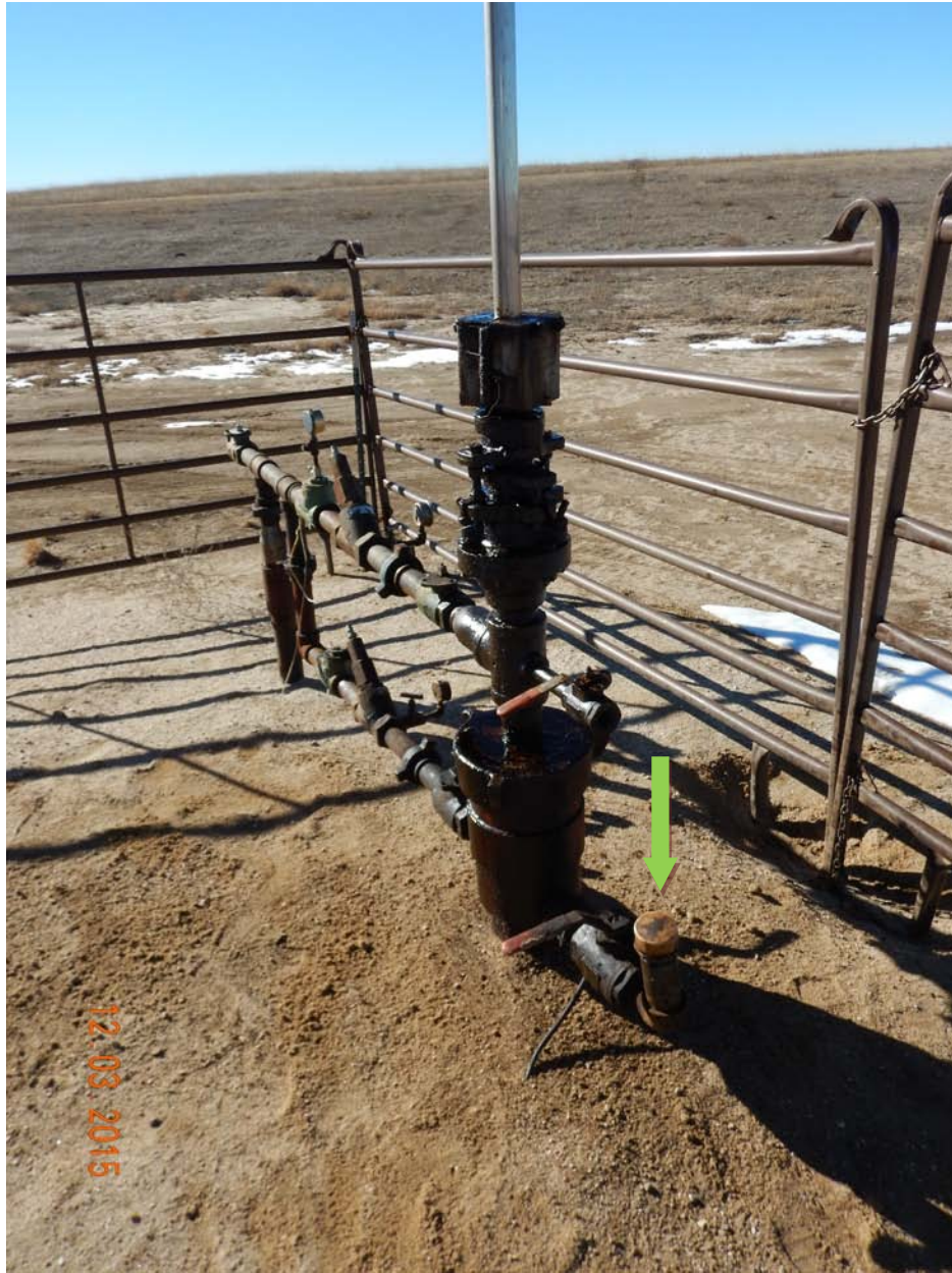
Figure 2 – Photo of wellhead. Vent nipple location indicated by green arrow.
