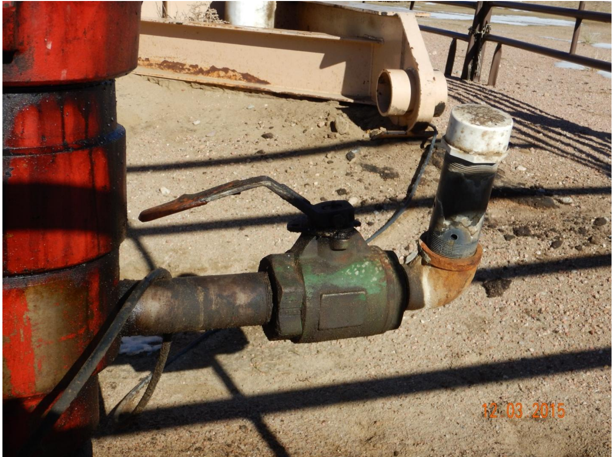
Figure 3 – Close up of vent nipple. COGCC Inspector's personal four-gas meter alarm was tripped for H 2 S and LEL.
