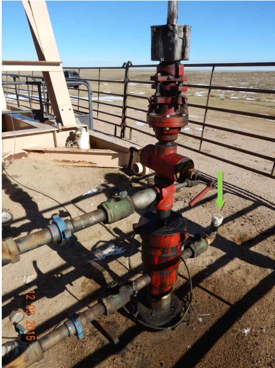
Figure 2 – Photo of actively venting wellhead with localized stained soil. Vent nipple location indicated by green arrow.
