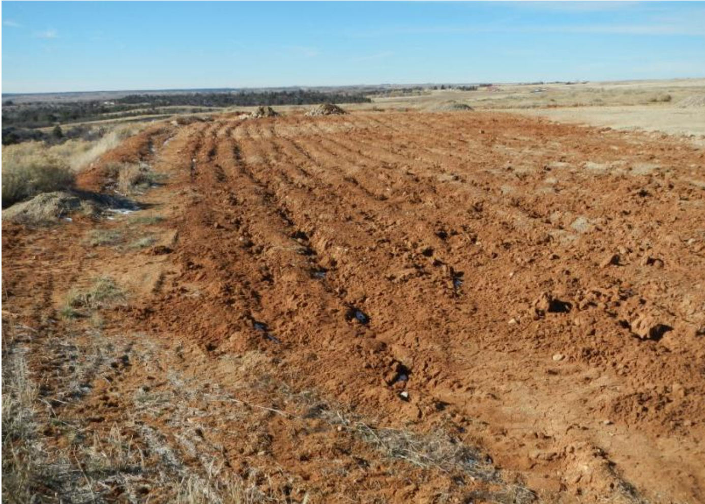
Photo 1. View of the southern portion of the well pad from the southeastern corner facing westward. This portion of the well pad appears to have been recently prepared for interim reclamation. Fill slopes are still present and recontouring needs to be completed.
