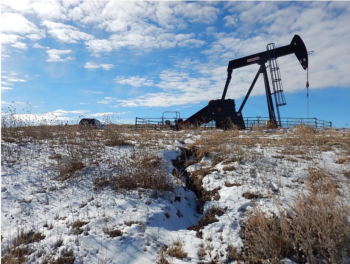
Figure 7 – Erosion channel on north side of drilling pad.
