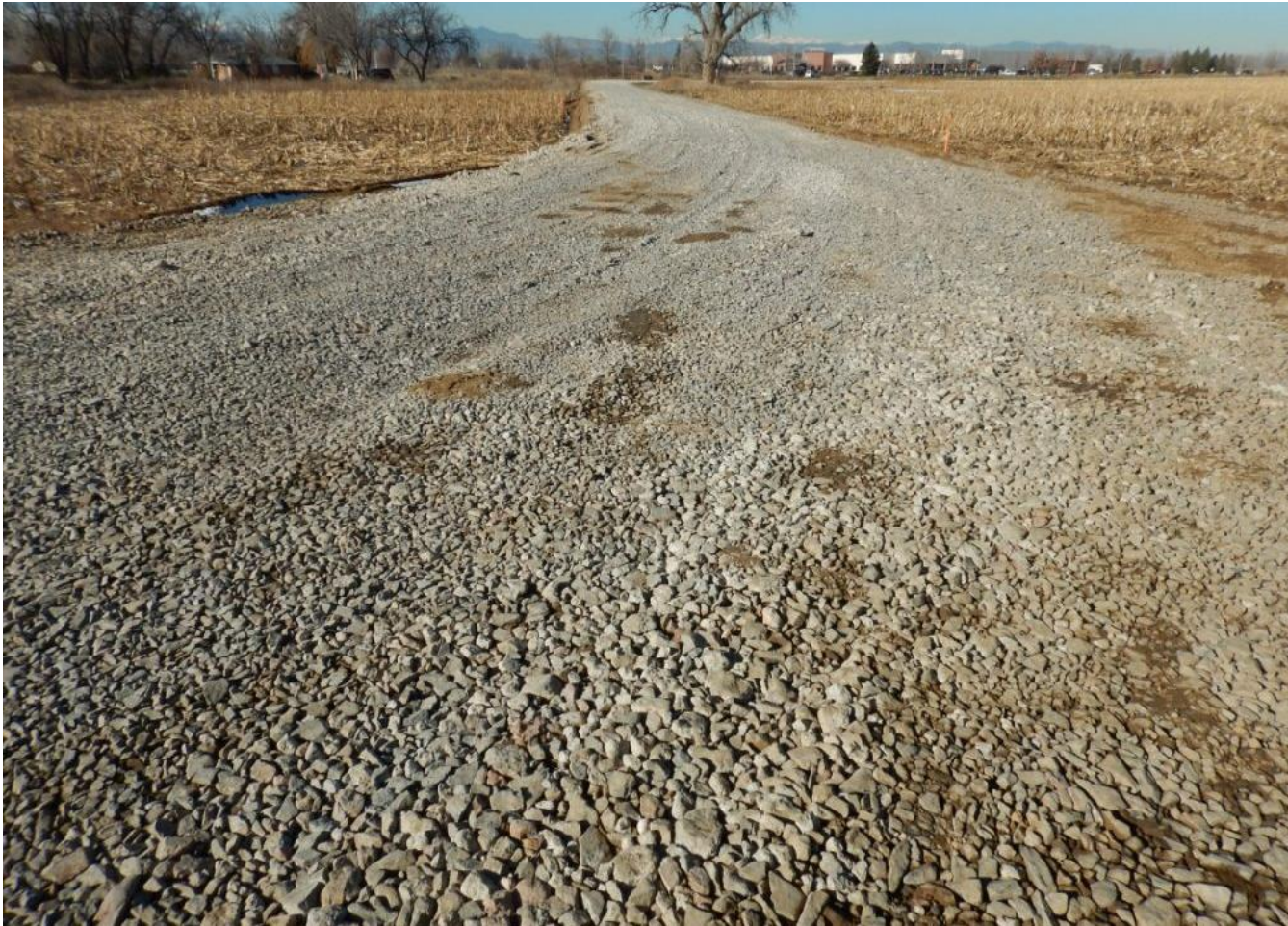
Photo 1. Photo taken from southern location, facing West. Operator installed cobble along entire access road to the pad.
