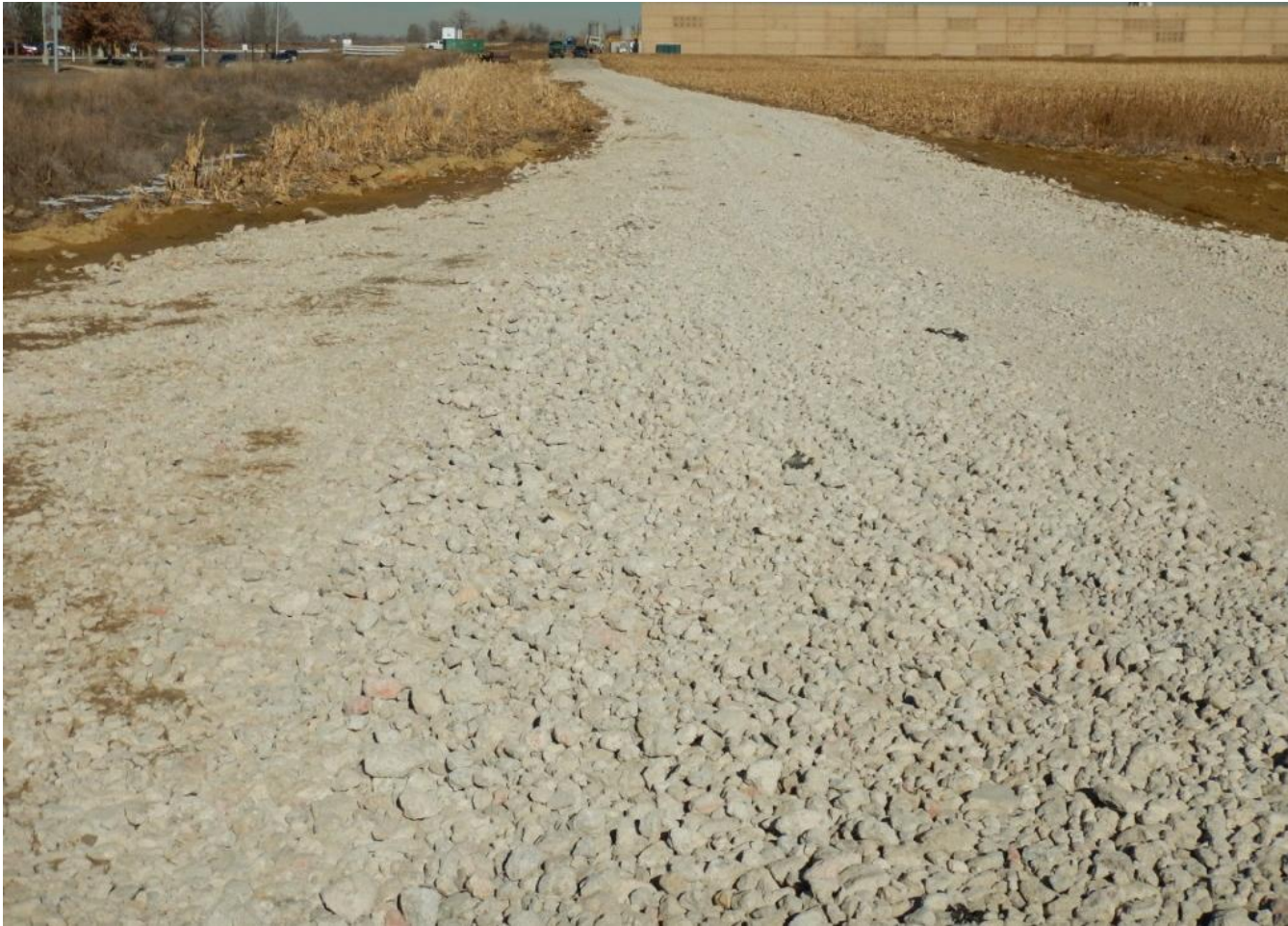
Photo 2. Photo taken from southwest location, facing North. Operator installed cobble along entire access road to the pad.
