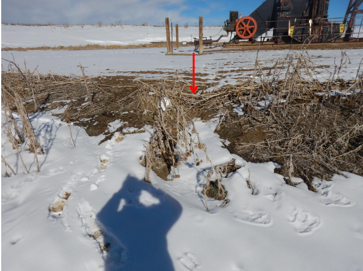
Photo 8: Photo taken from south end of location, facing north. Photo shows insufficient stormwater BMPs, and rill erosion (indicated with arrow). Photo shows Scotch thistle.
