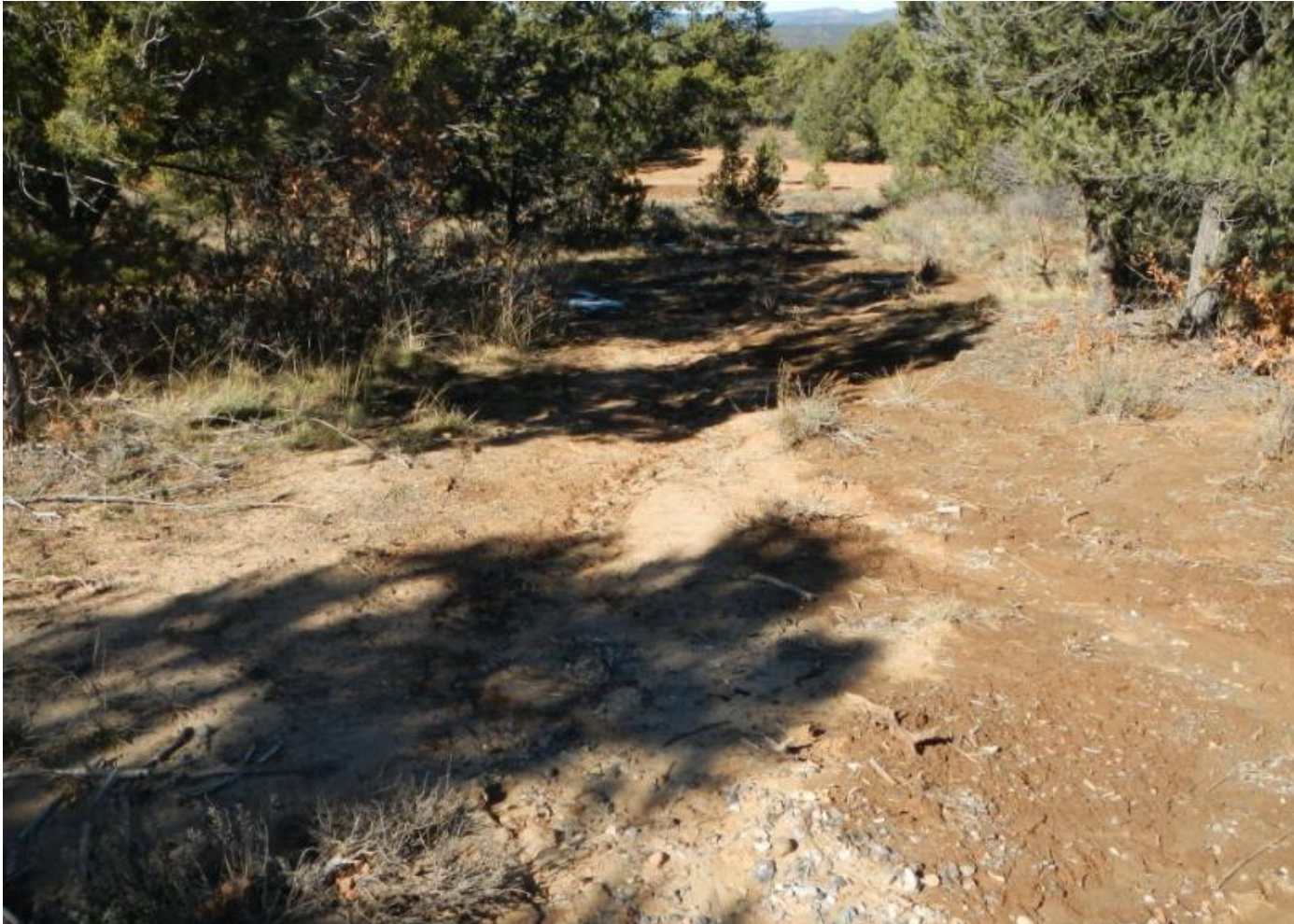
Photo 4. View of stormwater erosion where flows exit the northwestern corner of the project area (downstream).
