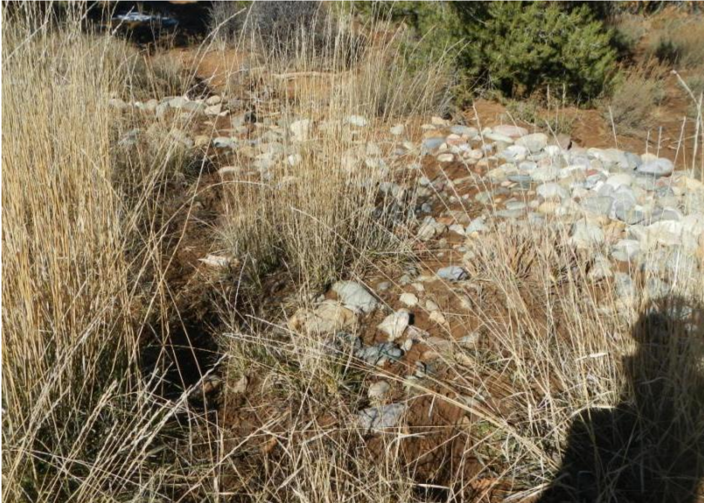
Photo 2. View of stormwater BMP in northeastern corner of project area. Sediment is accumulating here and it appears to need maintenance. If concentrated flows downstream of this area worsen, additional BMPs will be needed.
