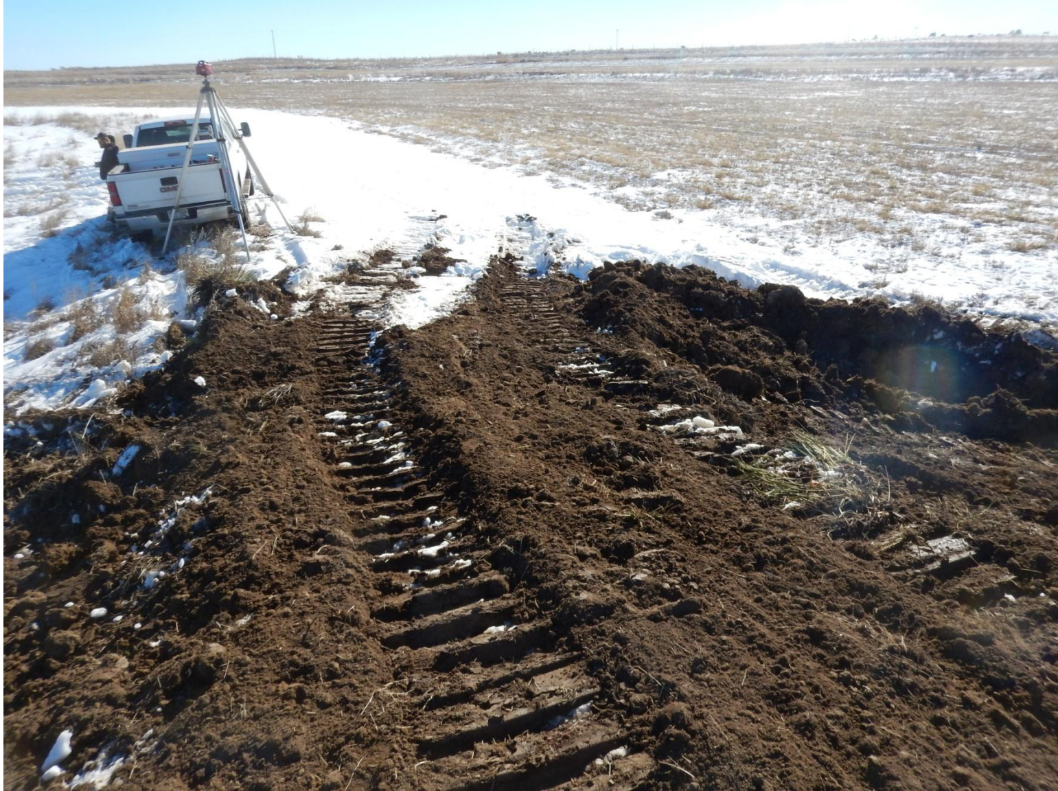
Photo 10: Photo taken from southeast end of location, facing southeast. Photo show insufficient stormwater BMPs in southeast corner of location.
