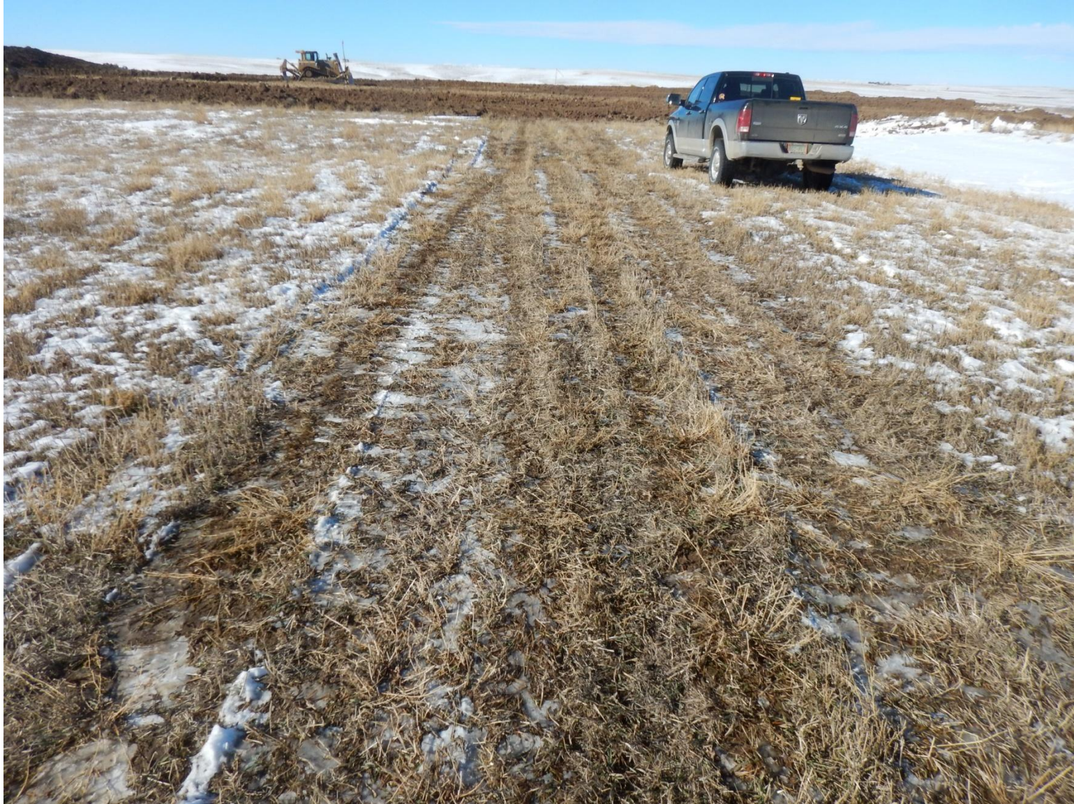
Photo 2: Photo taken east of location facing west. Note no defined access road or vehicle tracking BMPs in place to minimize disturbance and control sediment displacement by vehicles and/or equipment.
