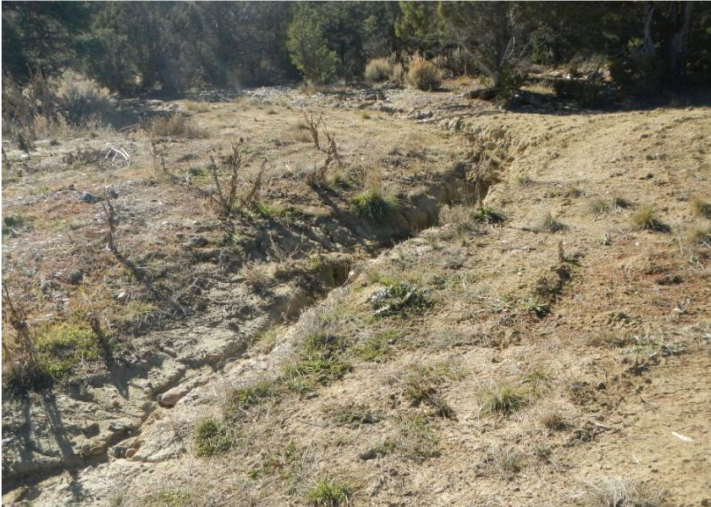
Photo 4. View of diversion channel that is eroding in northwestern portion of the project area. This portion of the project area needs stabilization measures and stormwater BMPs.
