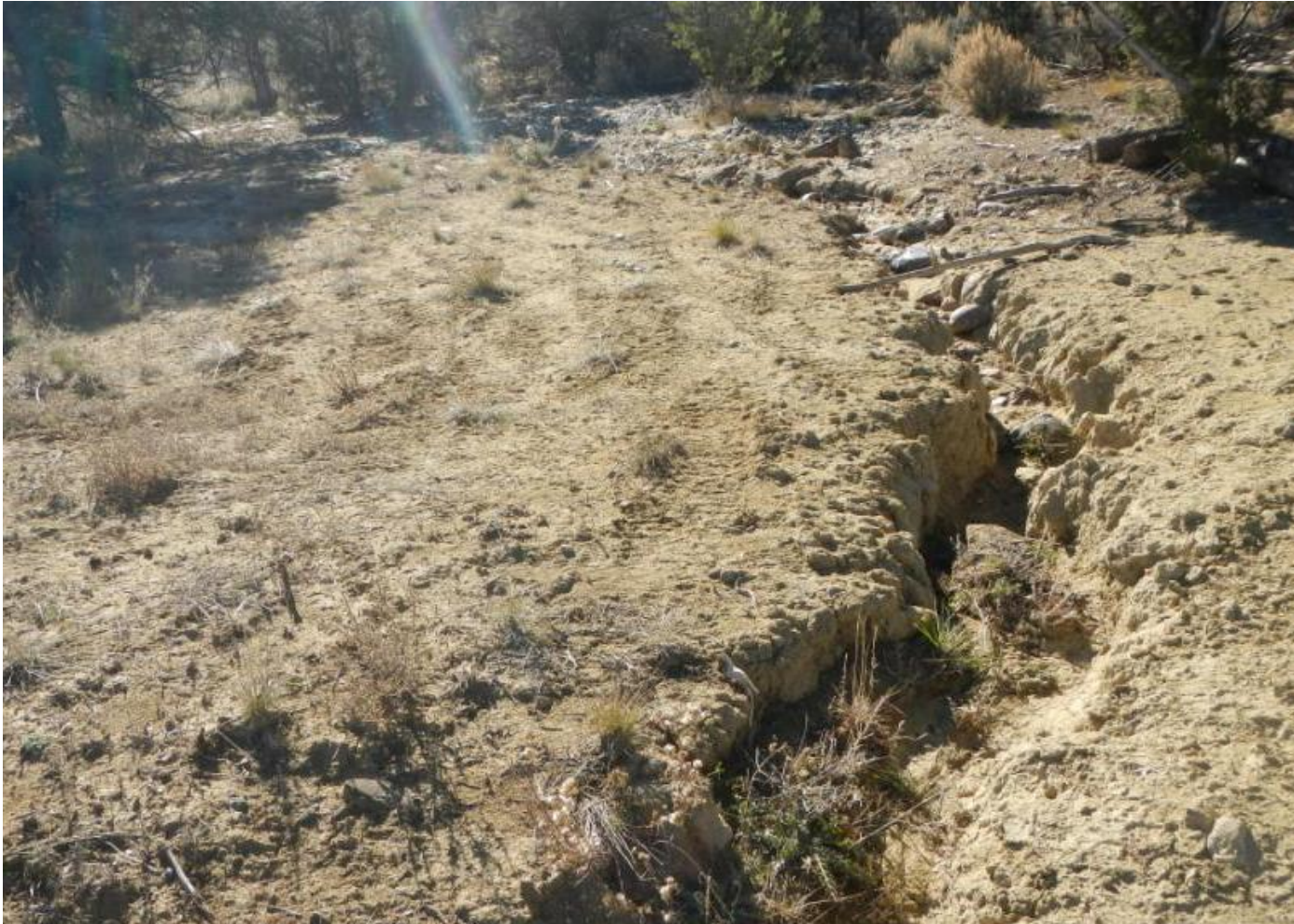
Photo 5. Another view of stormwater erosion in the northwestern corner of the project area (approximately 2 feet wide and 1.5 feet deep).
