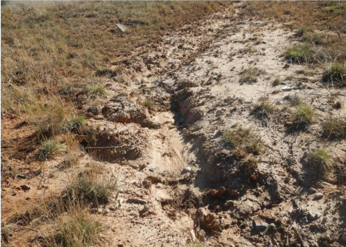
Photo 3. View of where stormwater diversion is eroding in northwestern corner of the project area. Erosional channel is approximately 2 feet wide and 1 foot deep. Stormwater BMPs are needed to de-energize and filter stormwater flows in this area.
