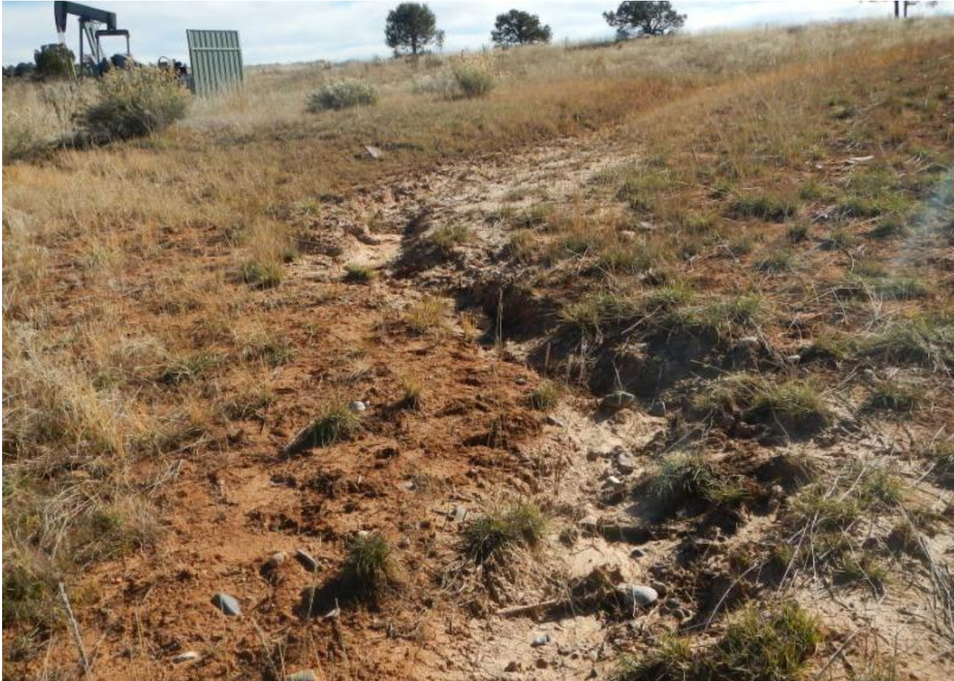
Photo 4. Another view of diversion channel that is eroding in northwestern portion of the project area. Stormwater BMPs are needed here.
