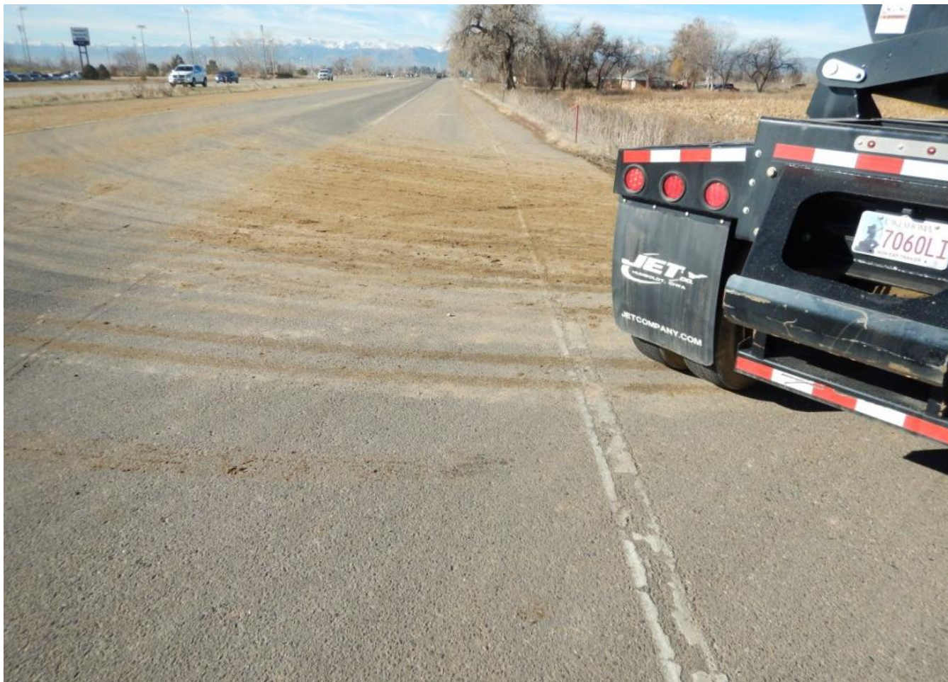
Photo 3. Photo taken from CO 119, facing West. Sediment leaving area from access road onto CO 119. Need to control sediment leaving area as mud attached to vehicle tires.
