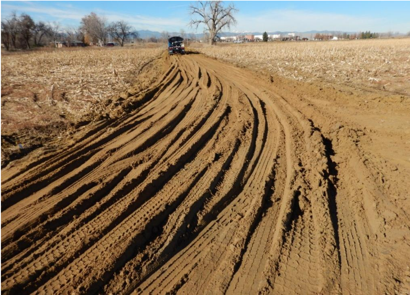
Photo 2. Photo taken from southern access road off CO 119. Need to control sediment leaving the area. Refer to photo #3.
