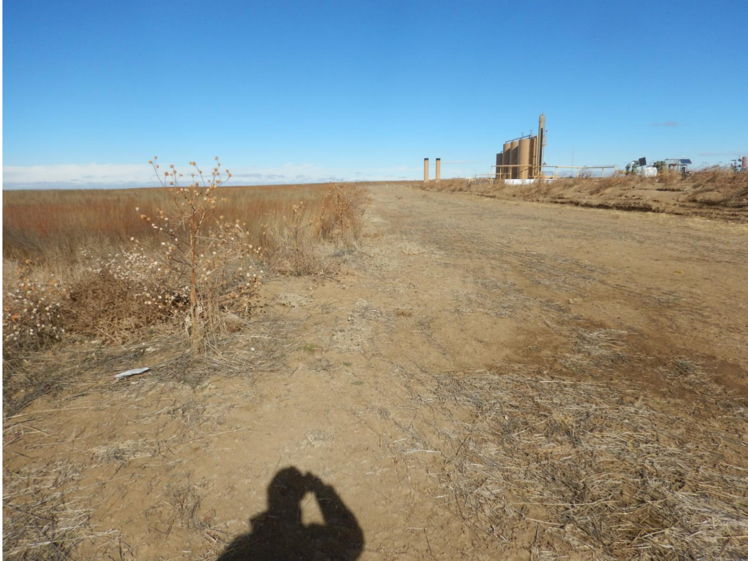
Photo 2: Photo taken from southwest portion of location, facing north.
