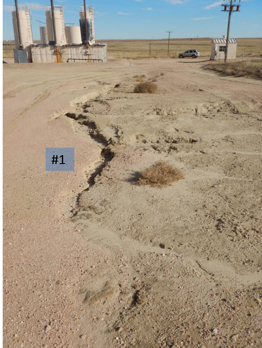
Photo 4: Photo taken from southern end of location, facing east. Note the rill erosion forming stormwater erosion channel #1.
