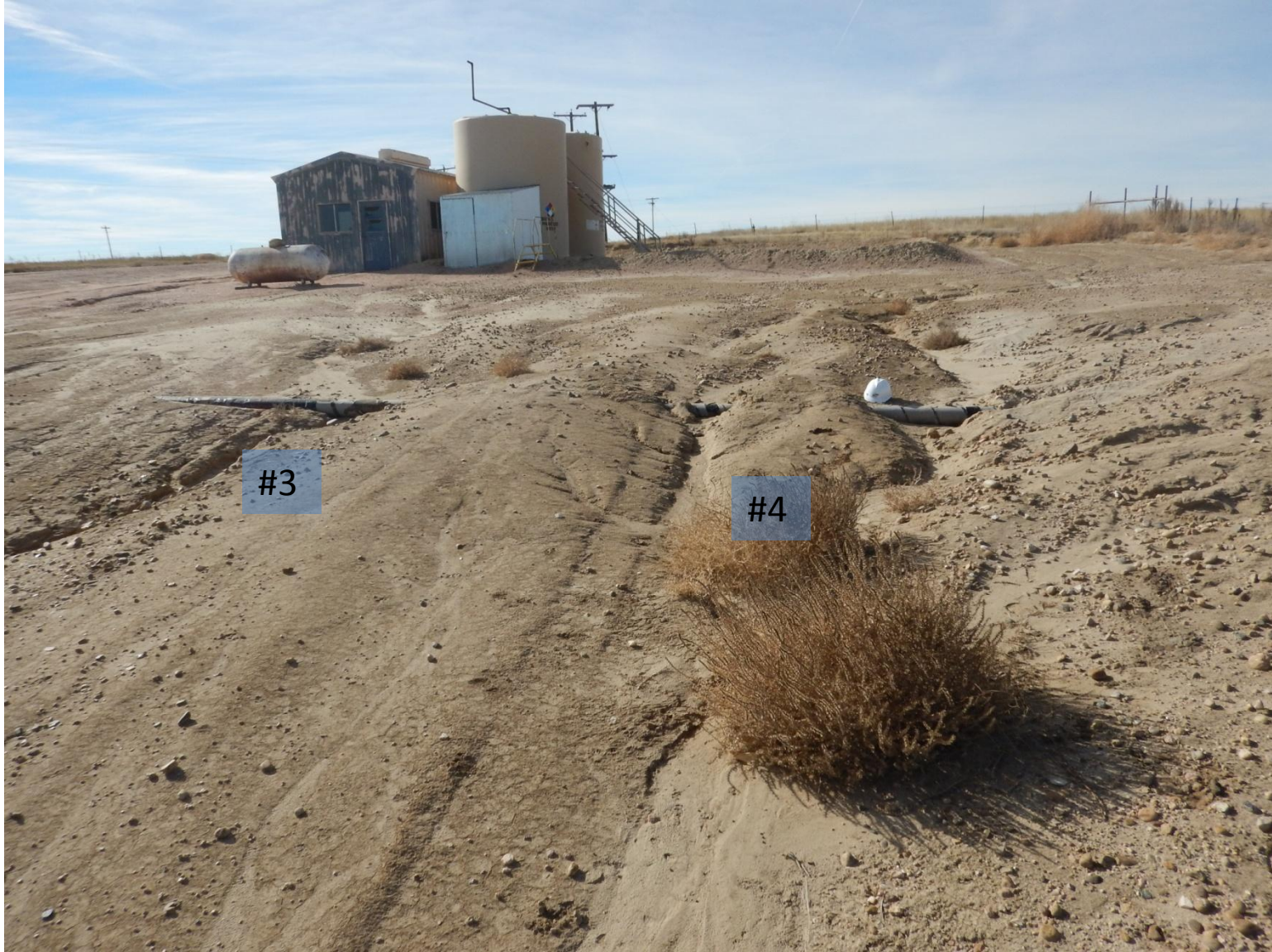
Photo 10: Photo taken from northern end of location facing west. Stormwater erosion channels #3 and #4 shown on northern half of location.
